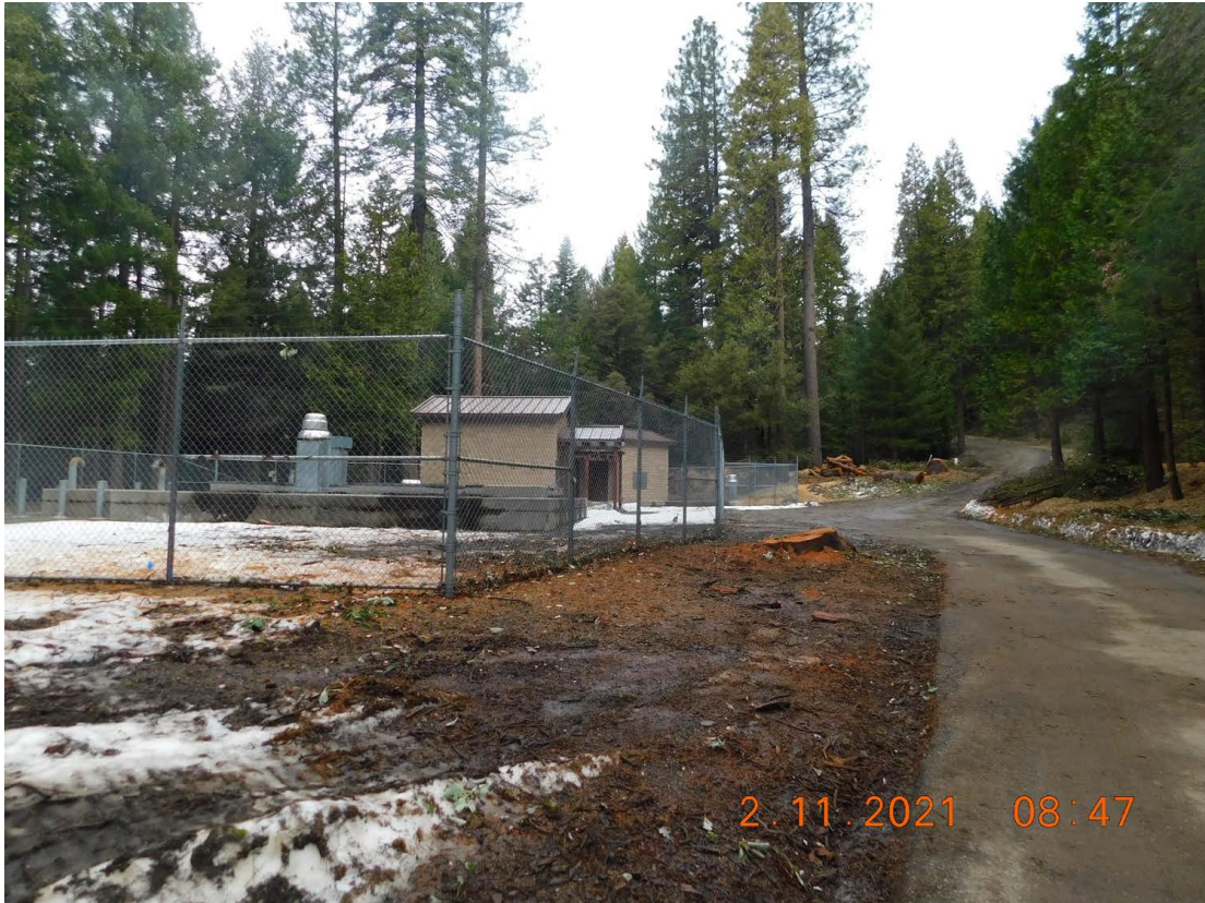
Post-removal conditions with hazard trees removed.
