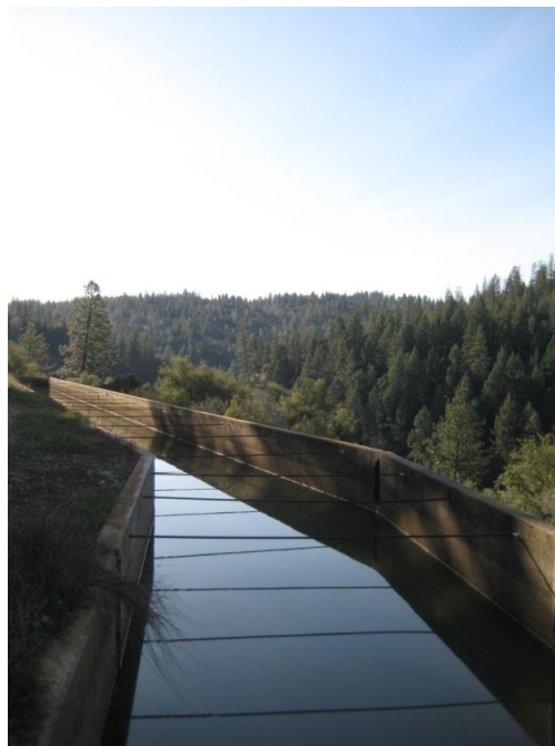
Combie Phase 1 Canal Narrow Wall at Risk and Stabilized with Tieback Supports
