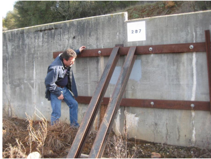
Combie Phase 1 Canal Typical Joint Separation Leaks and Temporary Repair
