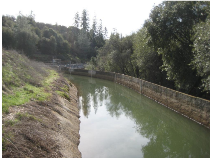
Photo 1-1 Combie Phase 1 Canal
