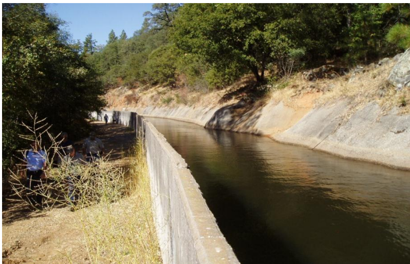
Photo 2-2 Combie Phase 1 Canal Narrow Concrete Wall
