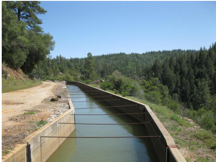
Combie Phase 1 Canal with Tie-backs for Stabilization
