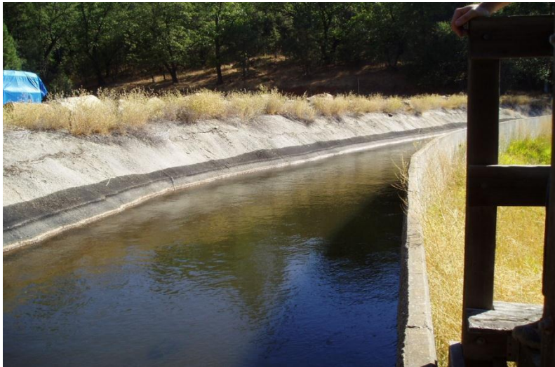
Photo 2-1 Combie Phase 1 Canal
