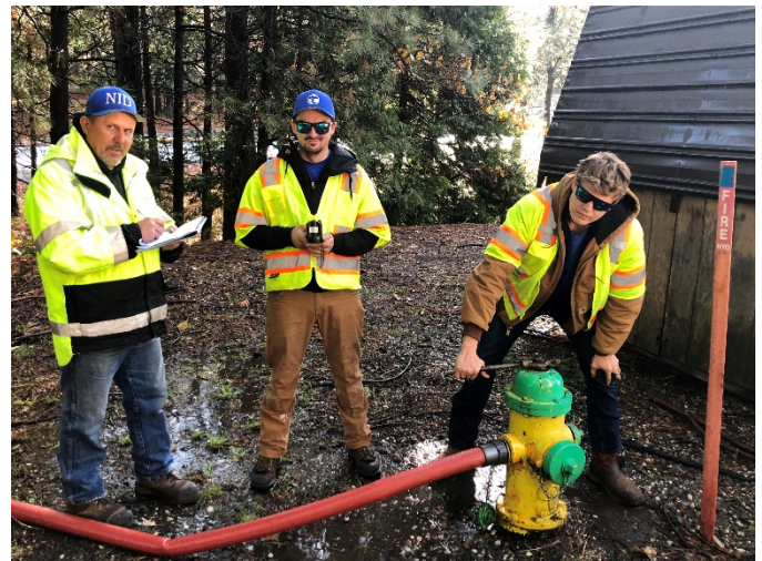
An NID crew cleans pipes by flushing water through a hydrant.
