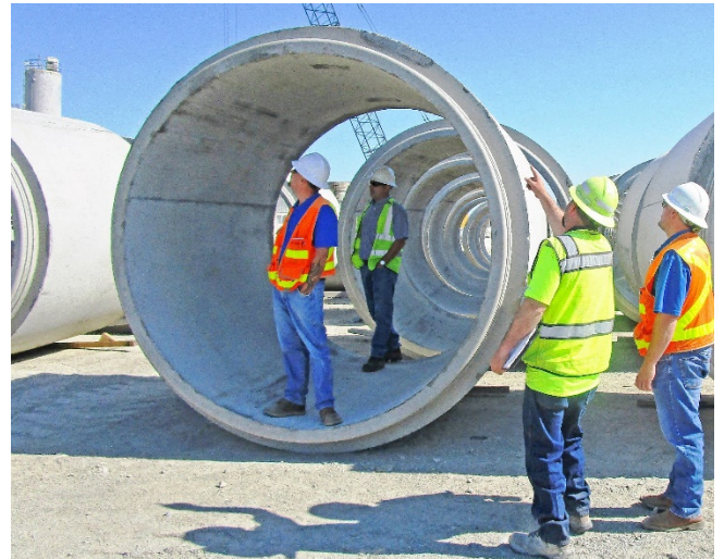
NID personnel inspect new pipe segments that will replace the canal.
