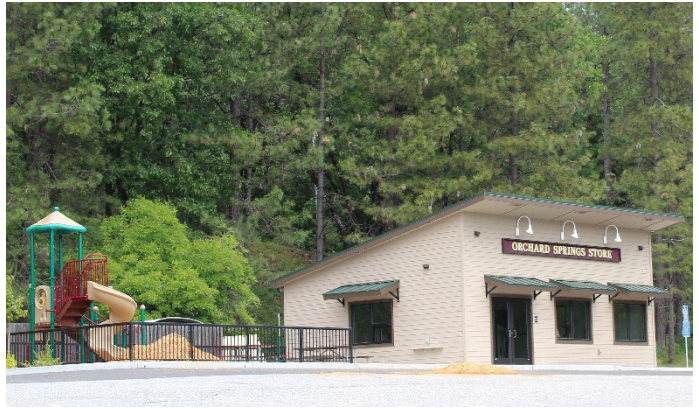
NID built a new camp store and added a kids' playground and native plant garden at the Orchard Springs marina at Rollins Reservoir.
