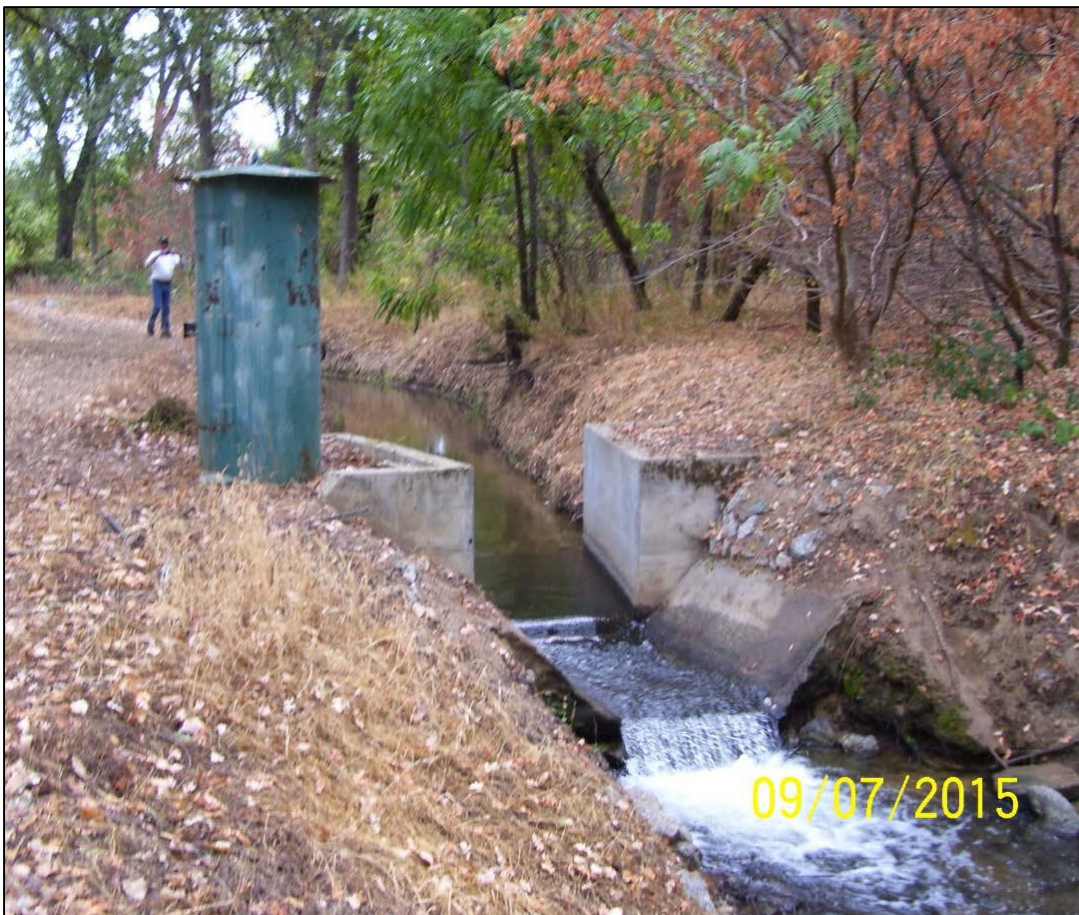
PHOTO 3-4 HEMPHILL CANAL AT THE PARSHALL FLUME
