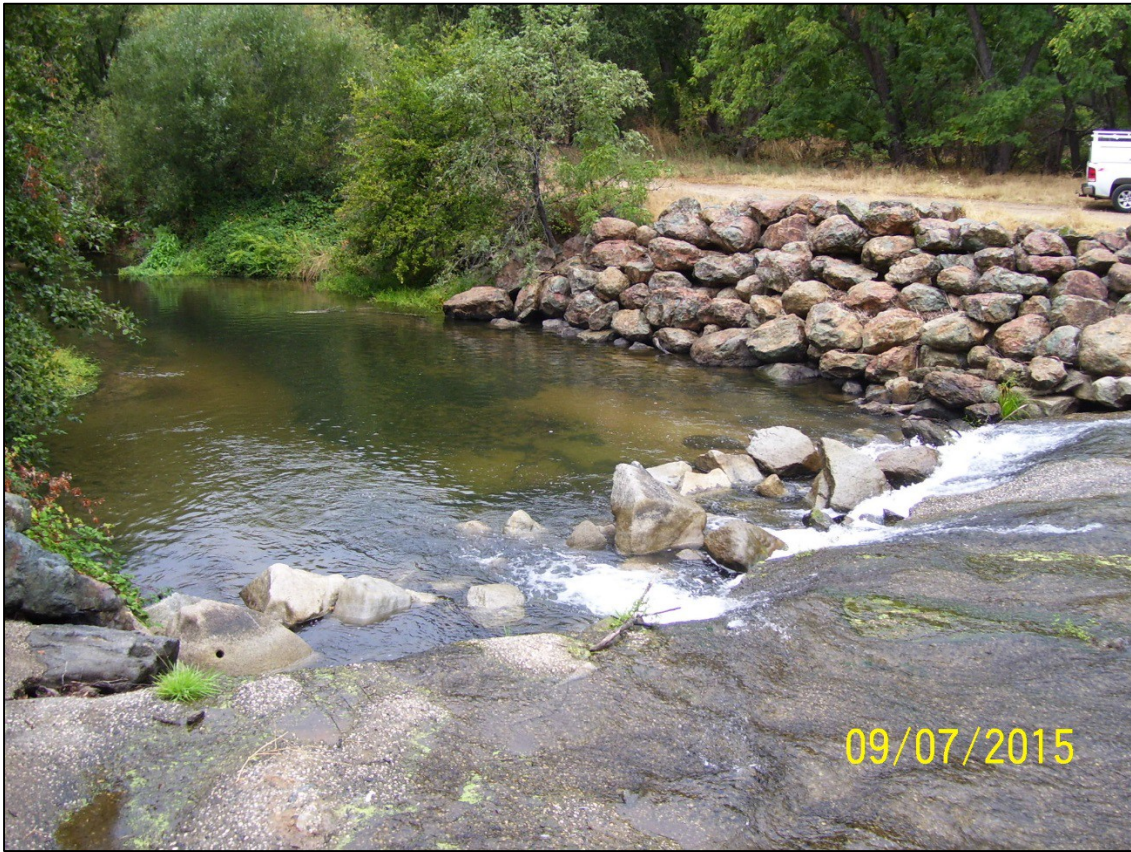
PHOTO 3-1 HEMPHILL DIVERSION STRUCTURE LOOKING DOWNSTREAM
