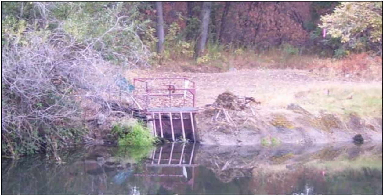
PHOTO 3-2 CANAL INTAKE STRUCTURE
