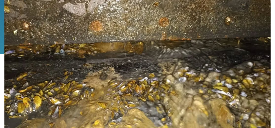
Figure 17: A colony of golden mussels ( Limnoperna fortunei ) in a hydroelectric powerhouse turbine room, Brazil.
