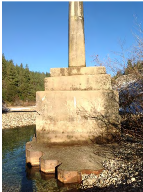
Figure 8 Chicago Park Powerhouse Bridge, Detail Photo, Facing Northeast
