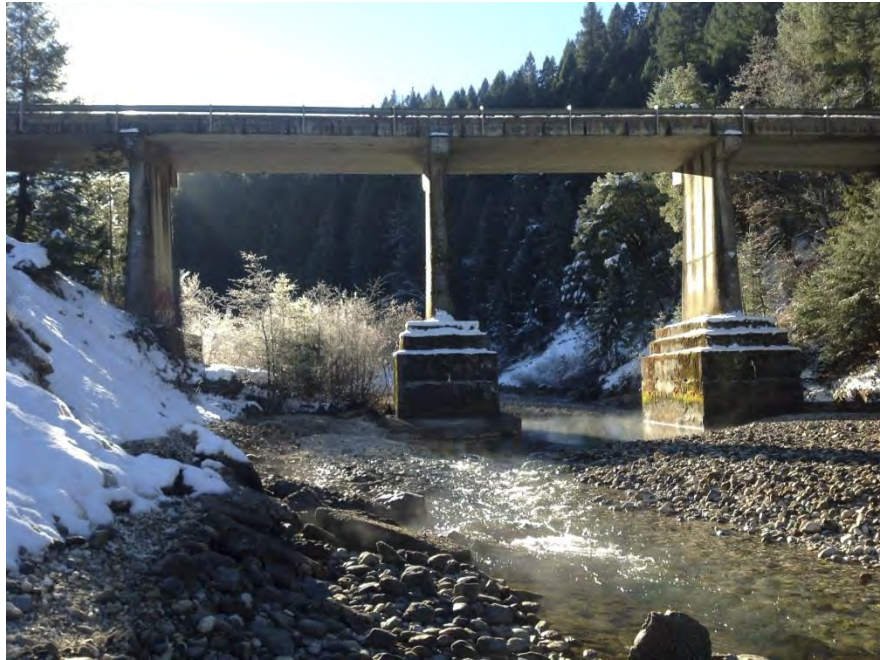
Figure 3.4-2 Chicago Park Powerhouse Bridge, Facing Northwest
