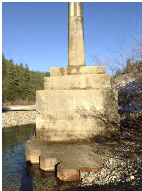
Figure 3.4-3 Chicago Park Powerhouse Bridge, Detail Photo, Facing Northeast
