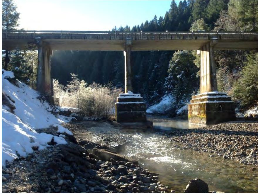
Figure 7 Chicago Park Powerhouse Bridge, Facing Northwest
