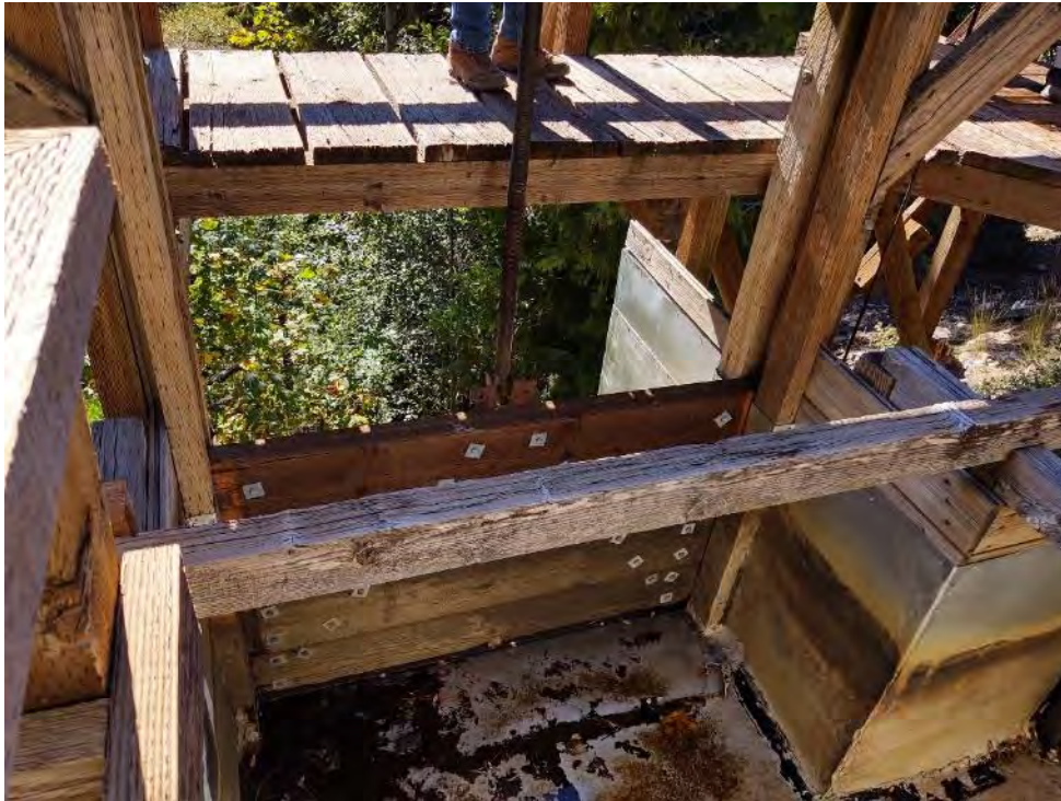
Photo 20 - View of Capehorn Spillway
