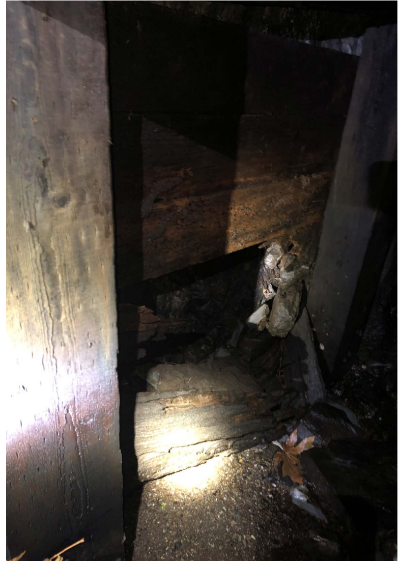
Big Tunnel Timber Sets 5+67
