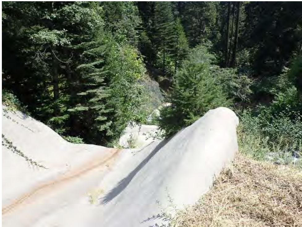
Photo 145 - View of Big Tunnel Spillway
