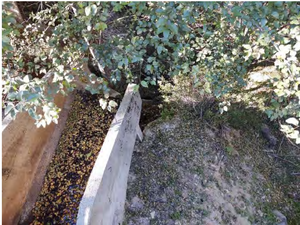
Photo 107 - View of 13 Mile Spillway
