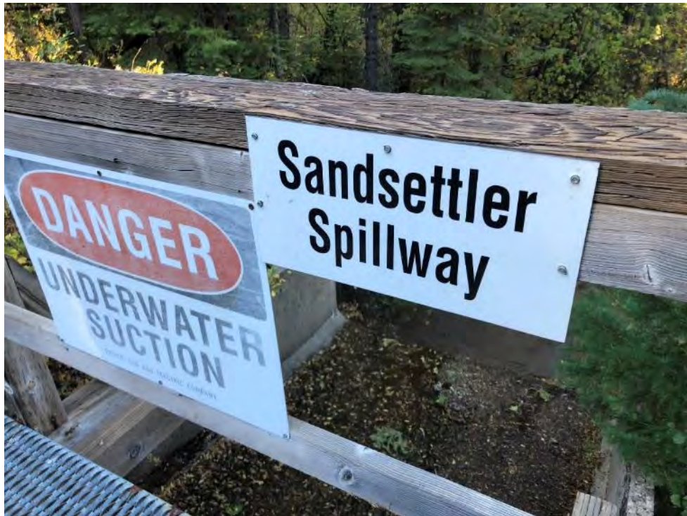
Photo 156 - View of Sandsettler Spillway
