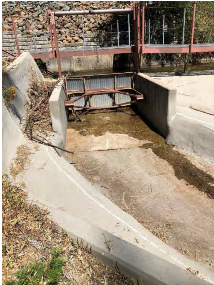
Photo 130 - View of Big Tunnel Spillway
