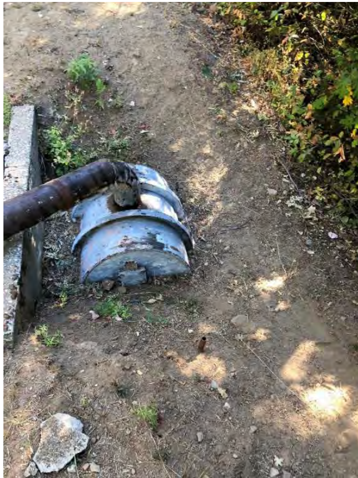
Photo 155 - View of Siphon Upstream of Sandsettler Spill Siphon
