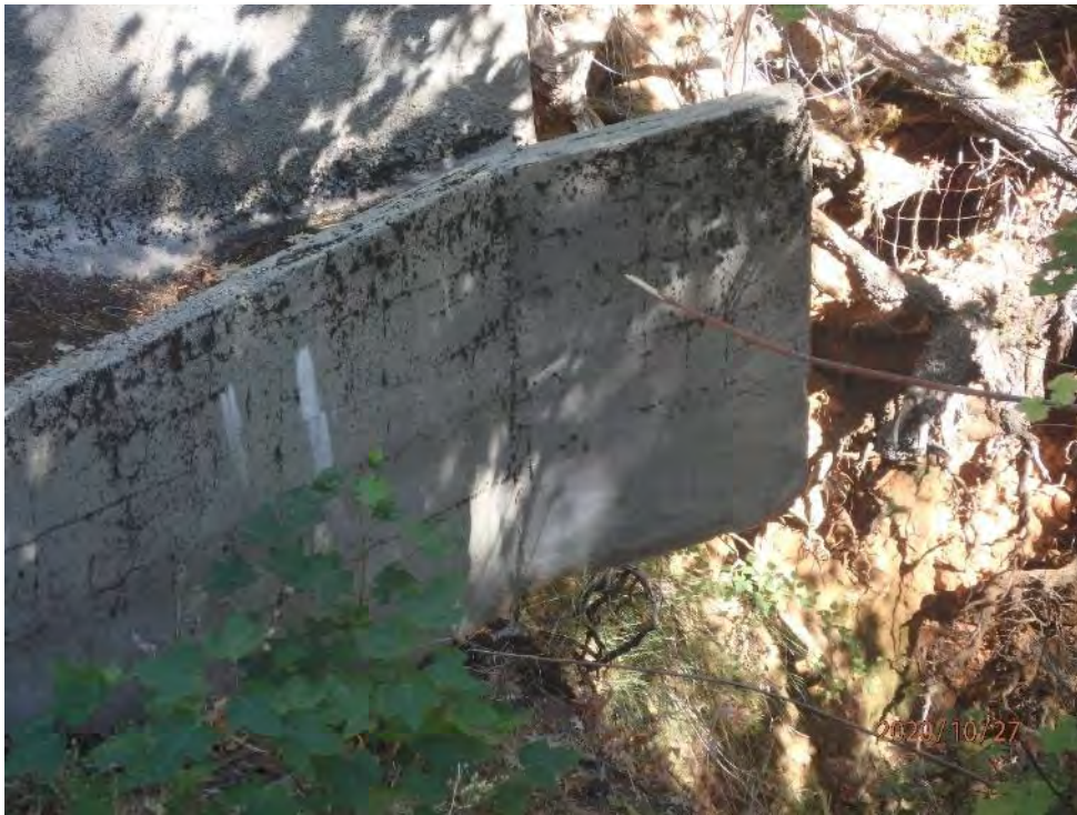
Photo 49 - View of Little Tunnel Spillway
