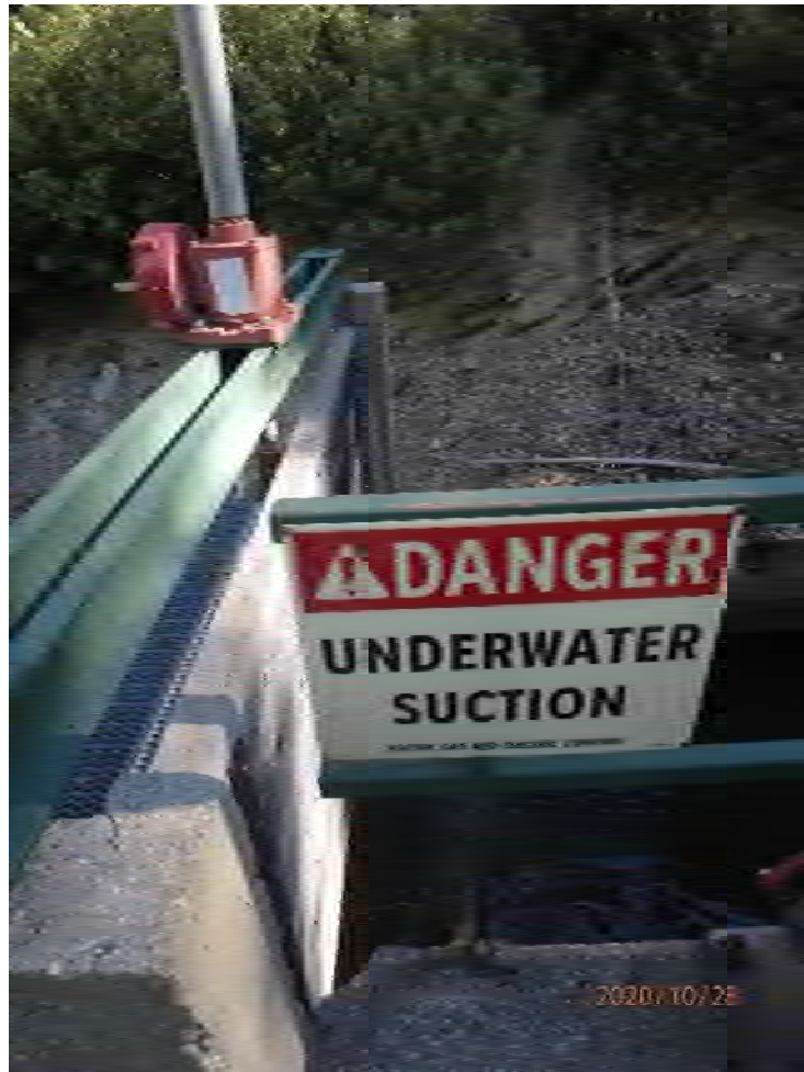
Photo 114 - View of 13 Mile Spillway
