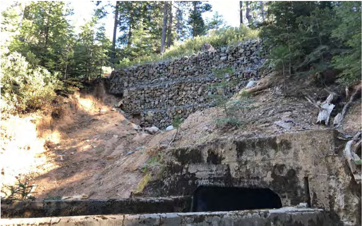
Little Tunnel Downstream Portal1
