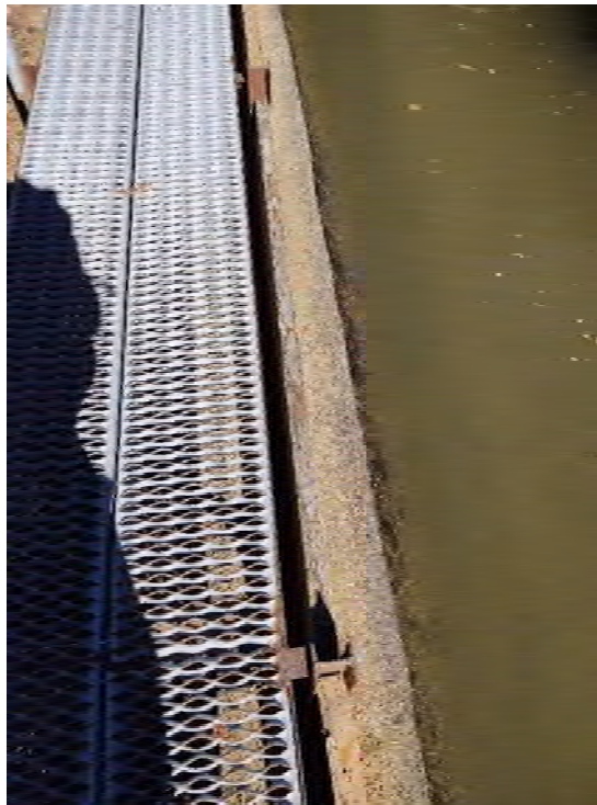
Photo 104 - View of 13 Mile Spillway
