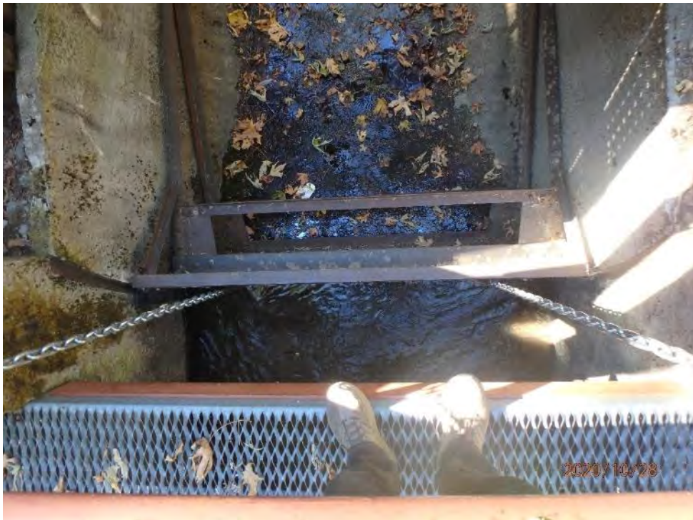
Photo 98 - View of Excelsior Point Gated Spillway
