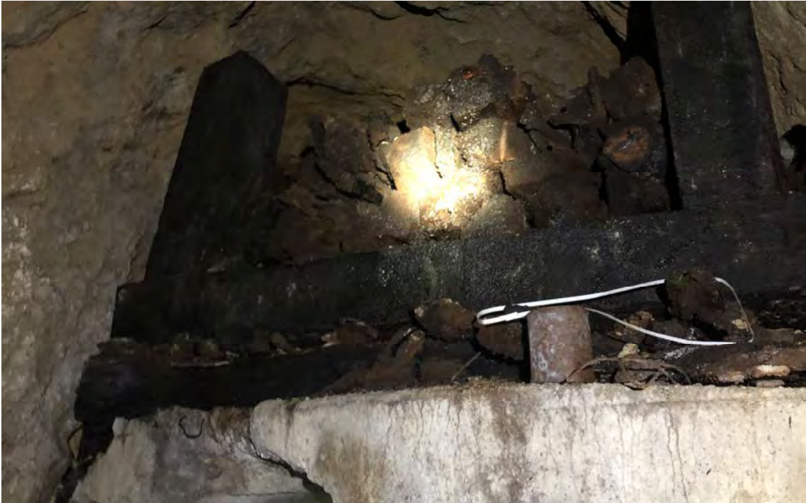
Big Tunnel Timber Crib Above Liner
