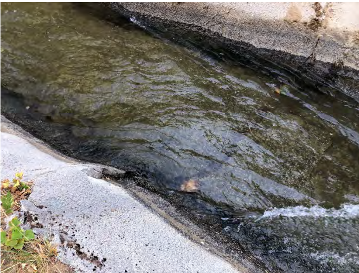
Photo 36 Potential Leak in Liner
