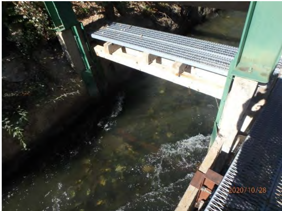
Photo 121 - View of 14 Mile Spill
