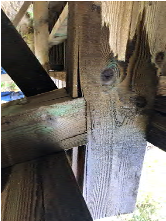
Photo 28 Crushed Girder in Timber Flume
