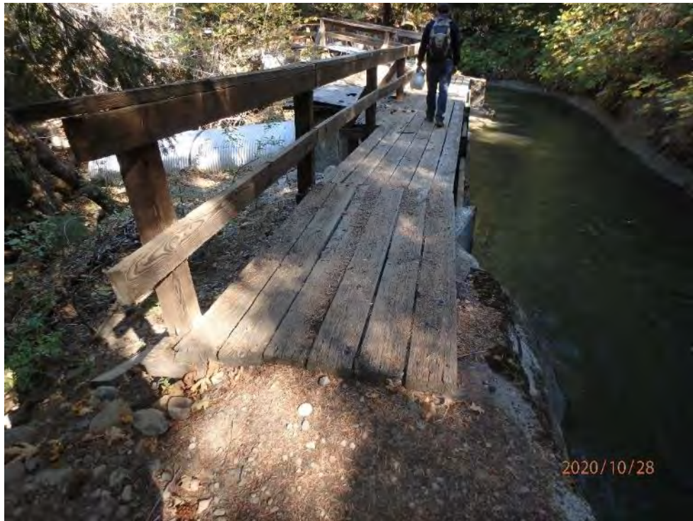
Photo 90 - View of Excelsior Point Flashboard Weir
