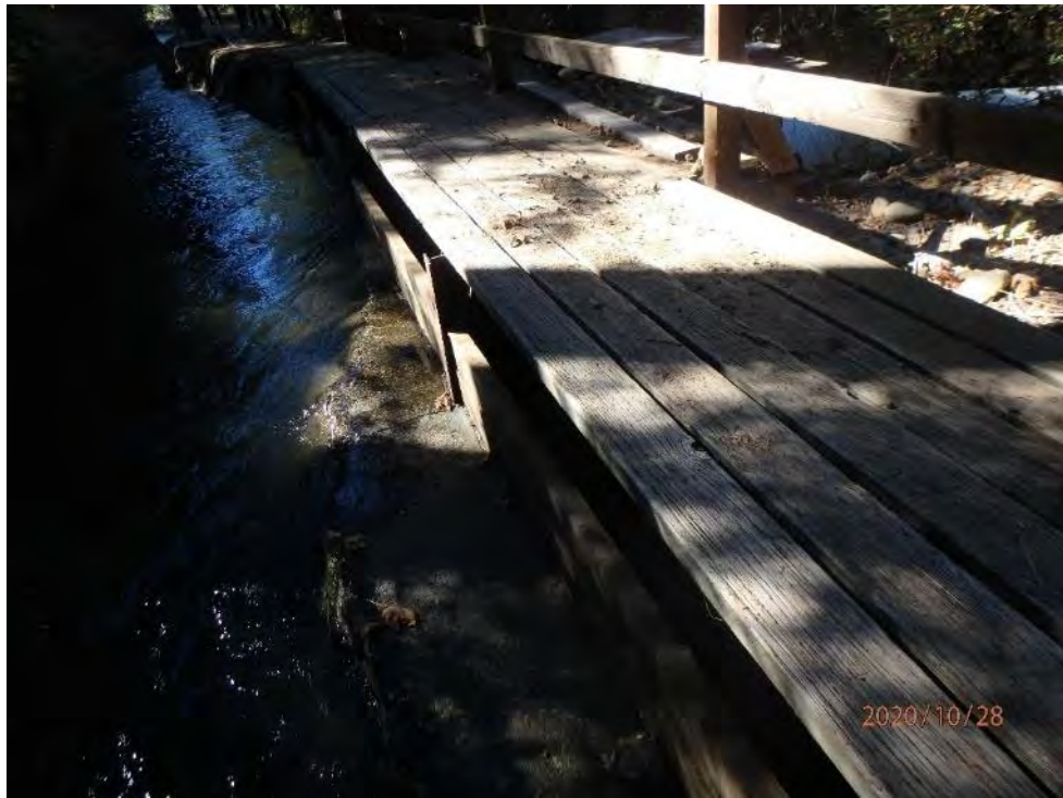
Photo 92 - View of Excelsior Point Flashboard Weir
