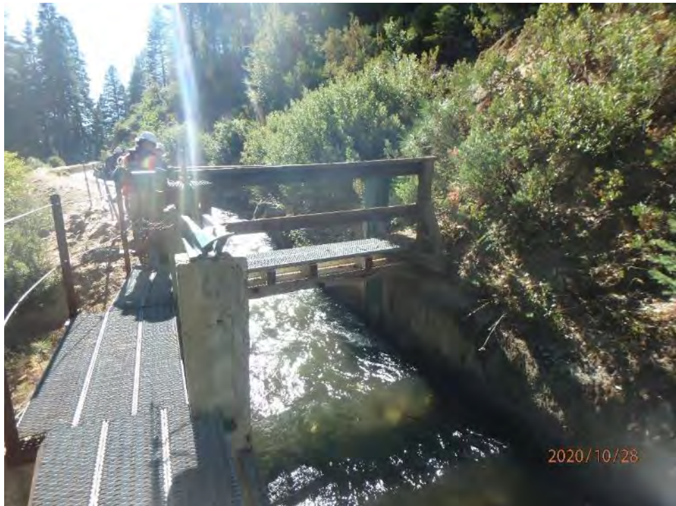
Photo 119 - View of 14 Mile Spill
