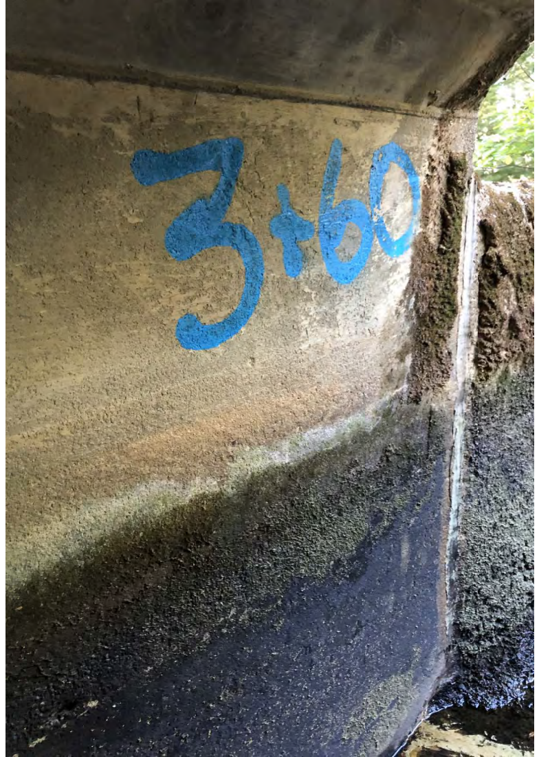
Little Tunnel Liner 3+60
