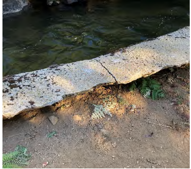
Photo 35 Void in Liner
