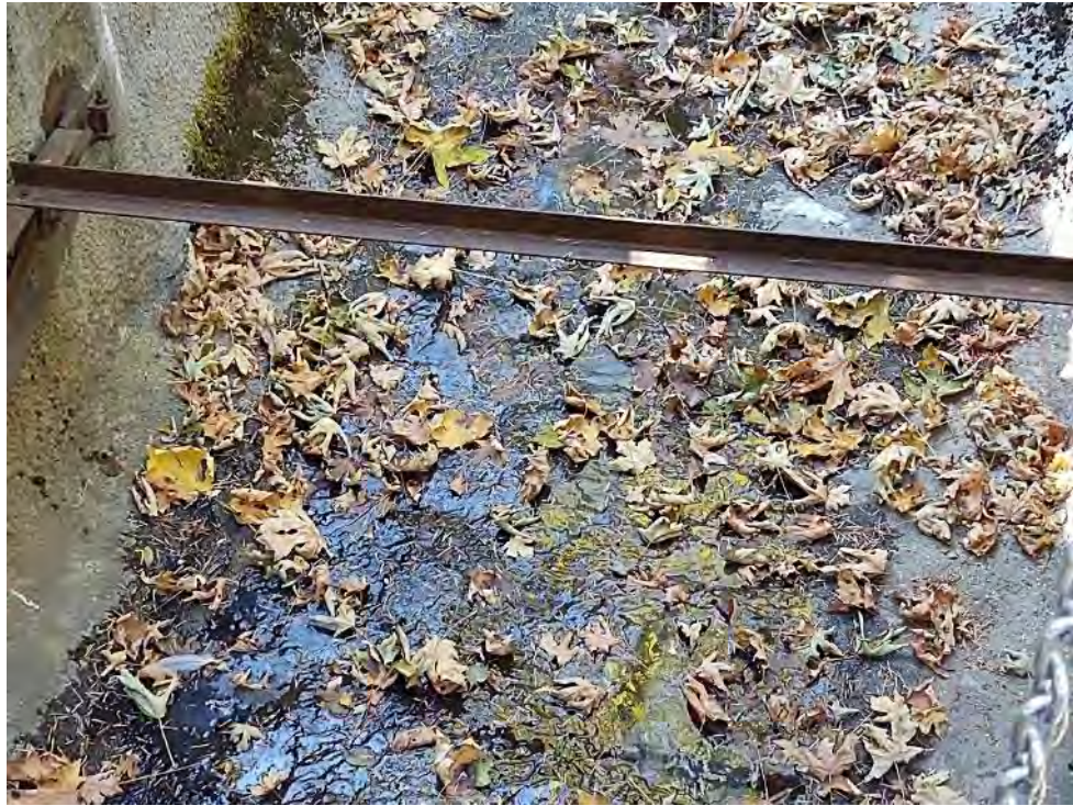
Photo 93 - View of Excelsior Point Gated Spillway
