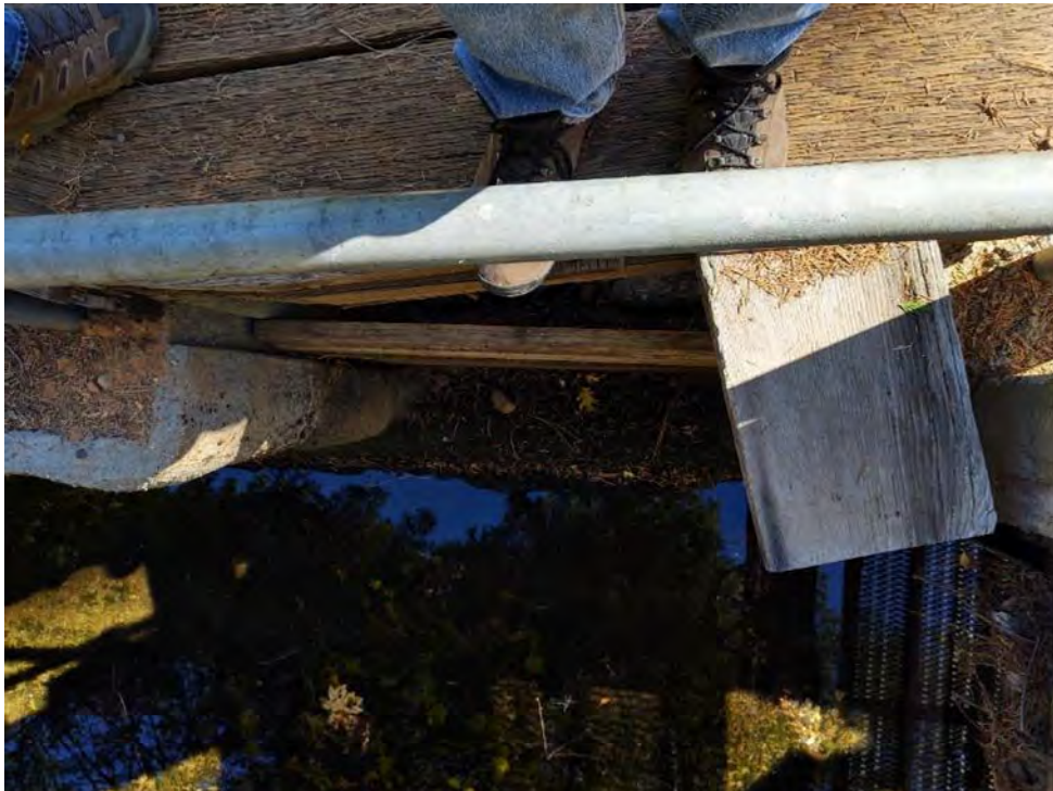
Photo 35 - View of Little Tunnel Spillway
