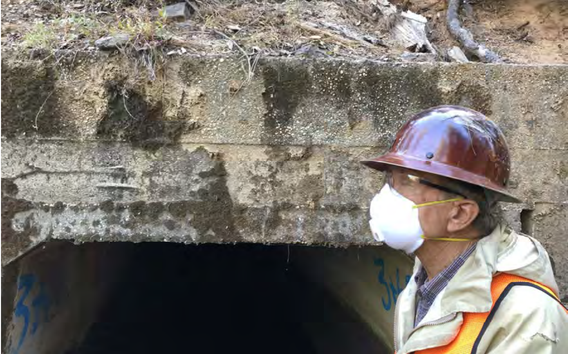
Little Tunnel Downstream Portal (2)
