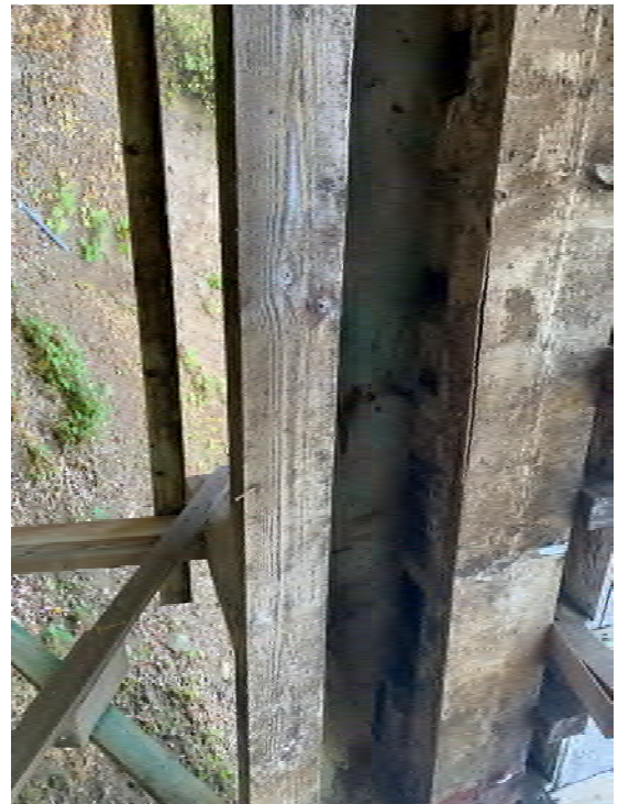
Photo 29 Split Girder in Timber Flume
