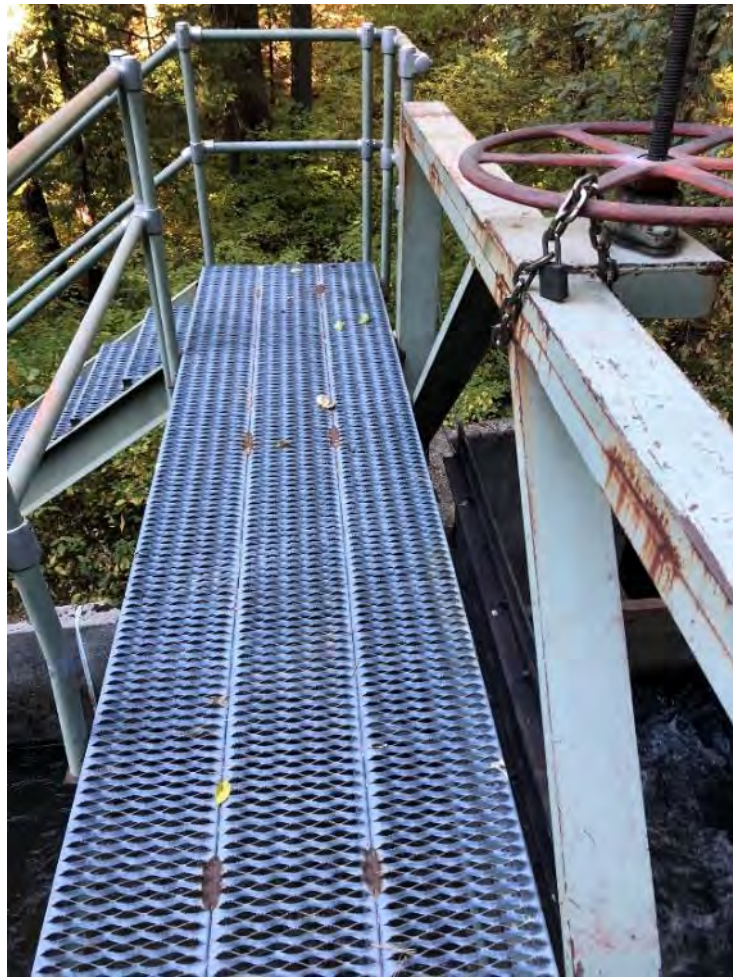
Photo 149 - View of Sand Bunker Spill
