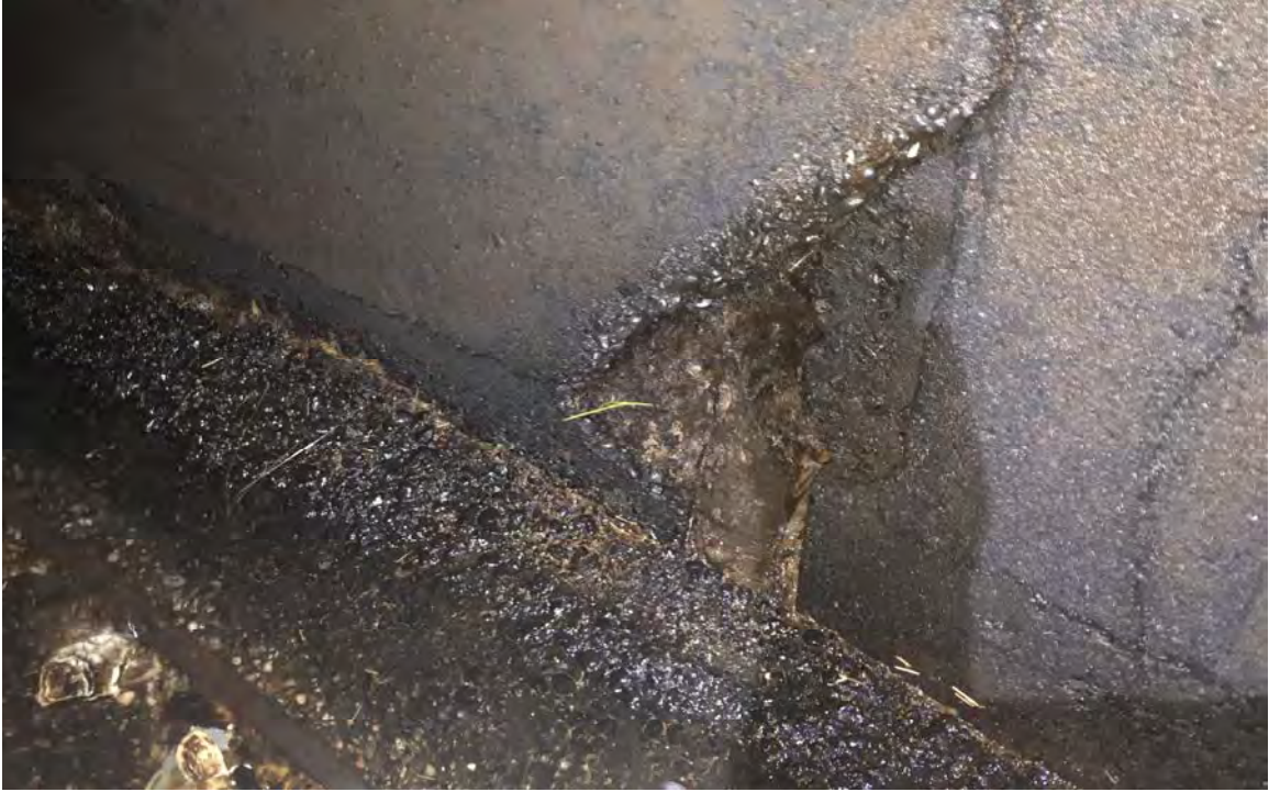
Big Tunnel 0+70 Thin Cover
