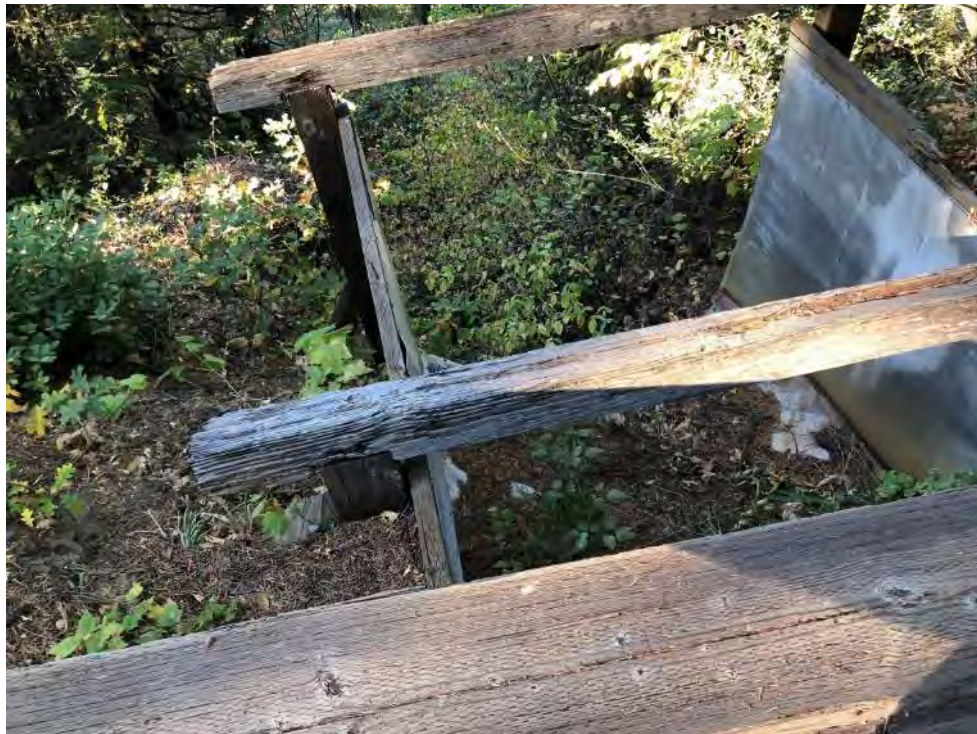
Photo 164 - View of Yunks Spill
