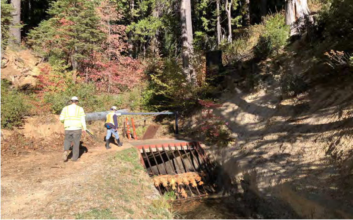
Big Tunnel Portal
