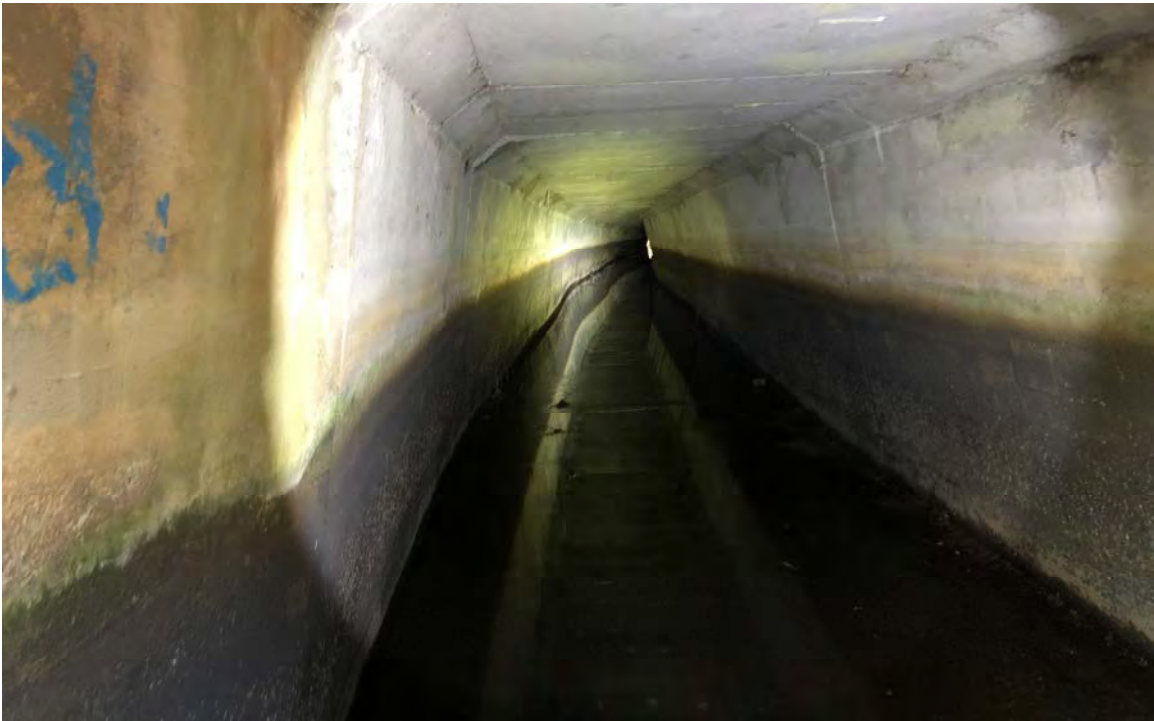
Little Tunnel Liner 3+60 (4)
