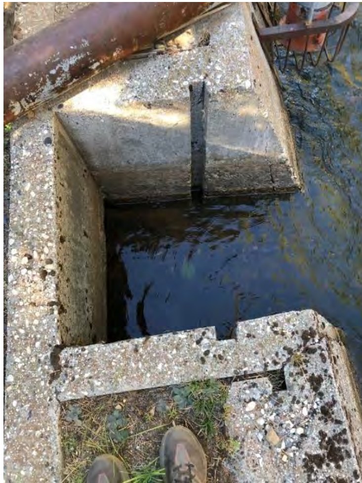
Photo 64 - View of 9 ½ Mile Spill Siphon
