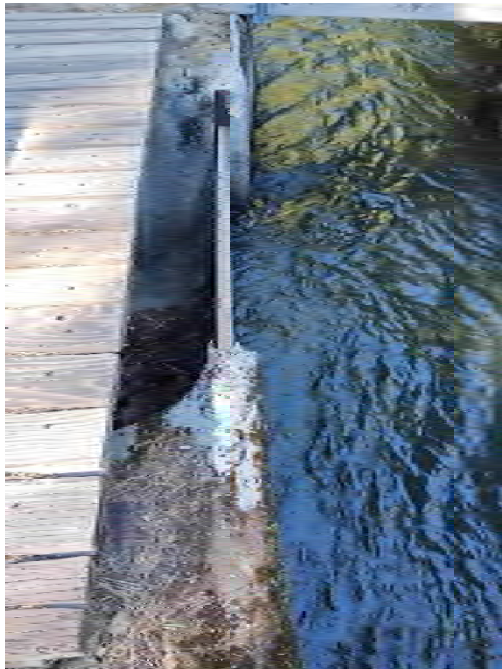
Photo 75 - View of Hickman Spill
