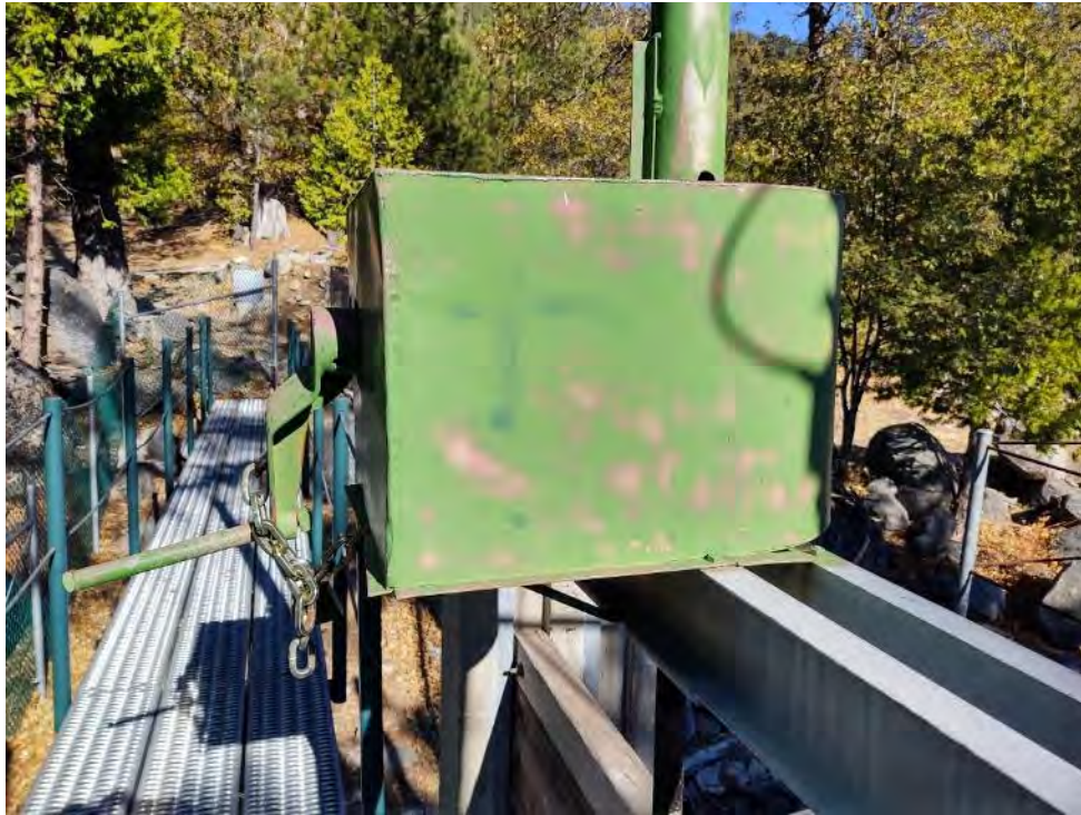
Photo 9 - View of Bear Valley Spillway
