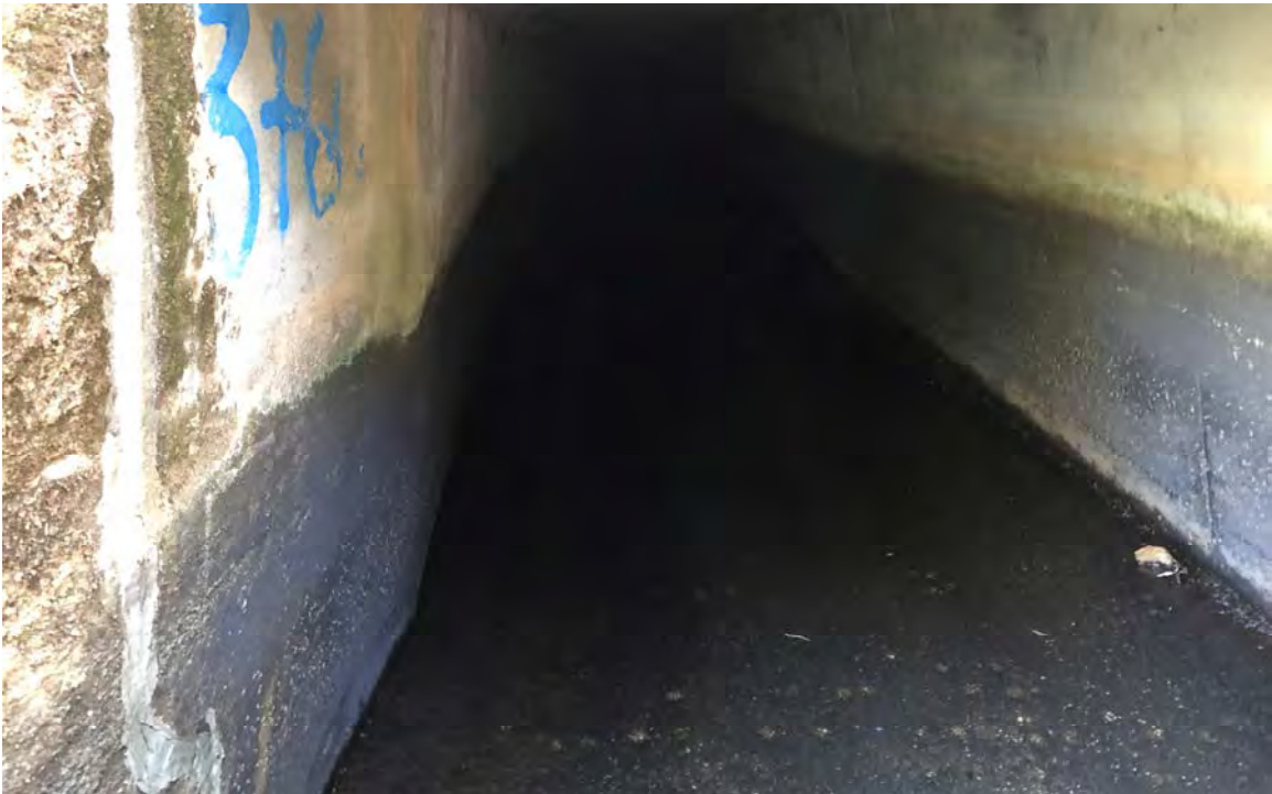
Little Tunnel Liner 3+60 (2)
