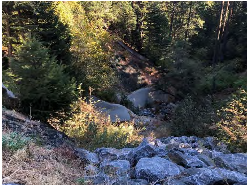
Photo 140 - View of Big Tunnel Spillway
