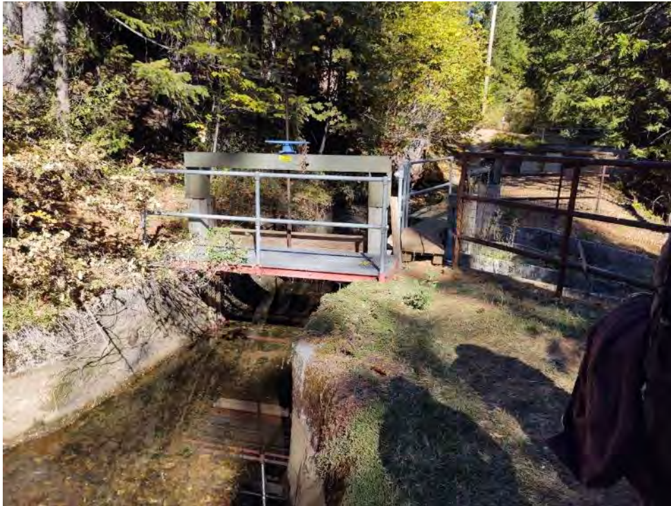
Photo 39 - View of Little Tunnel Spillway
