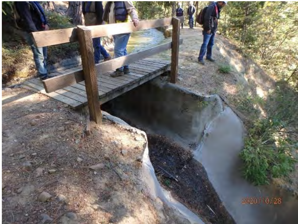
Photo 80 - View of Hickman Spill
