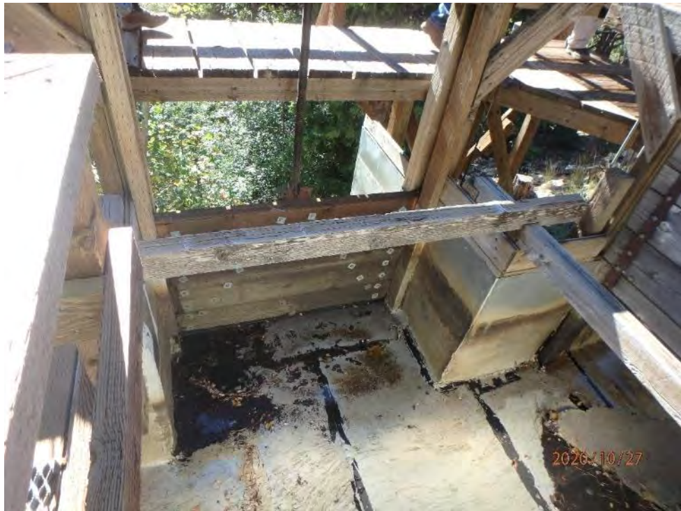
Photo 26 - View of Capehorn Spillway
