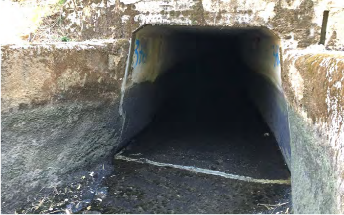
Little Tunnel Downstream Portal
