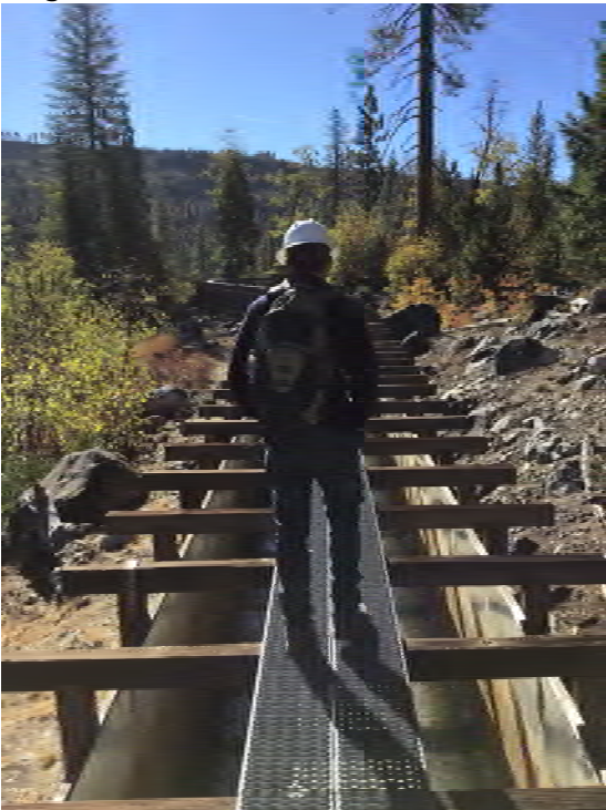
Photo 11 Flume out of Plumb
