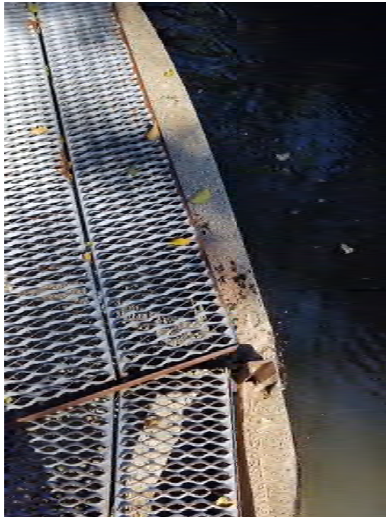
Photo 105 - View of 13 Mile Spillway
