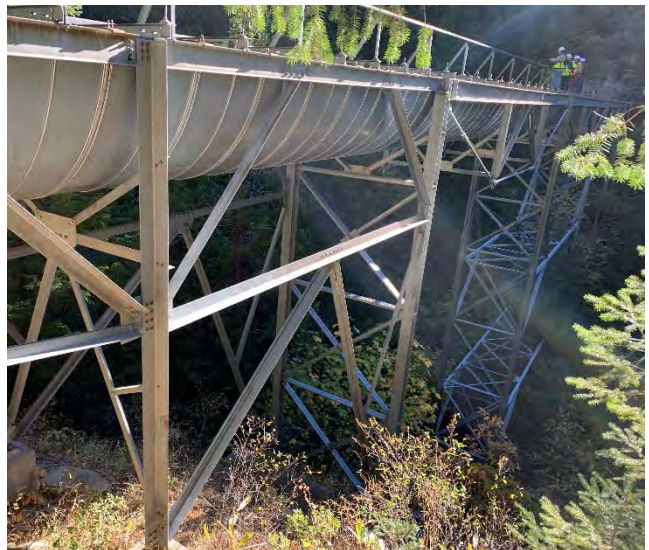
Photo 21 Steep Hollow #1 Lennon Flume
