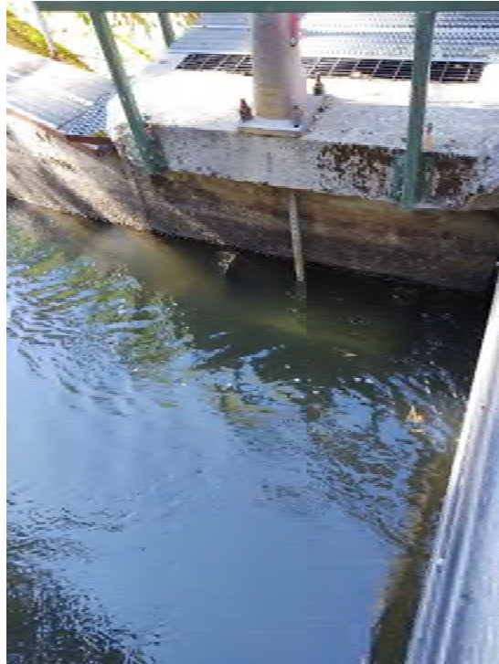
Photo 110 - View of 13 Mile Spillway
