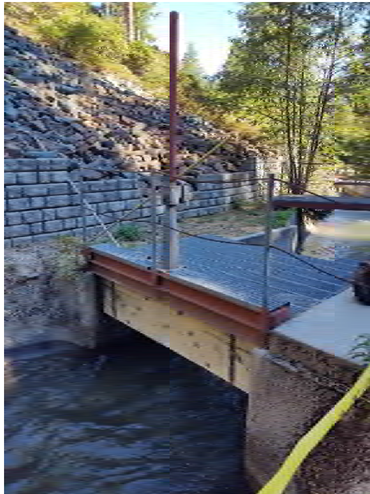
Photo 141 - View of Big Tunnel Spillway
