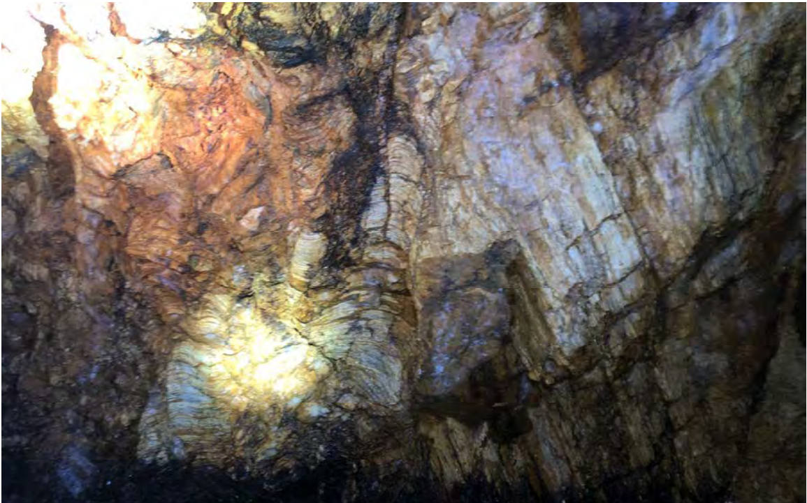
Big Tunnel 19+91 Shear2
