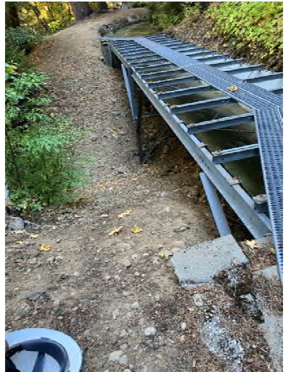
Photo 25 Historic Landslide at Flume 11/2
