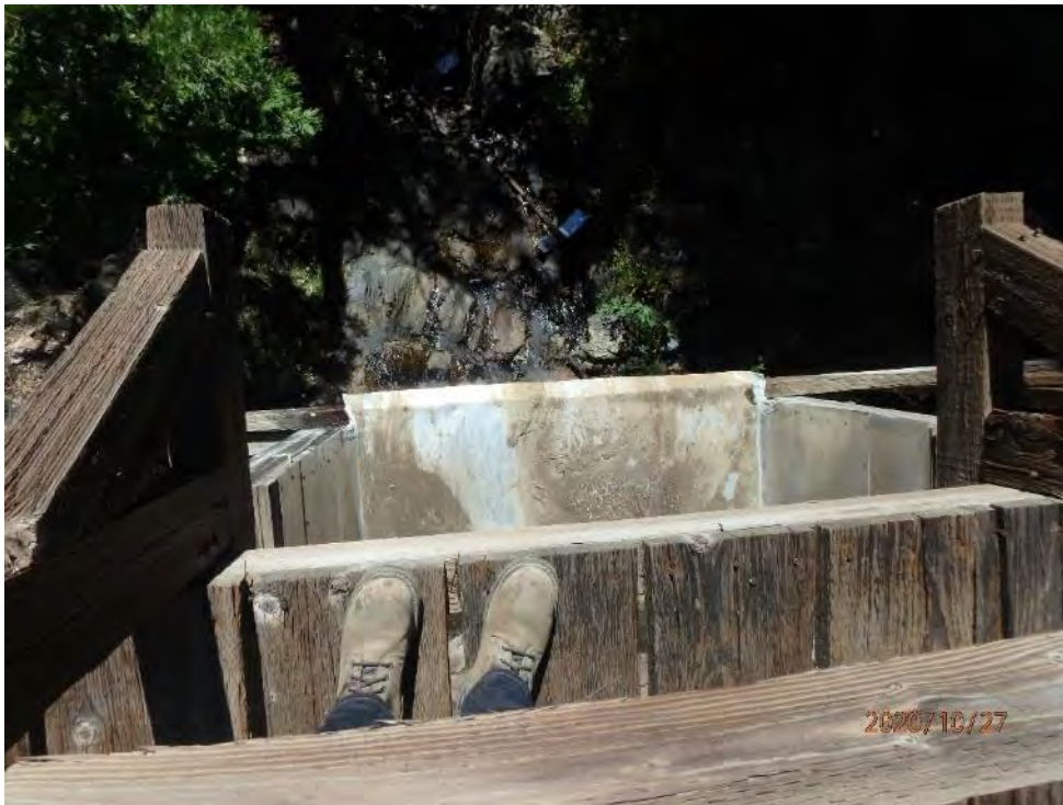
Photo 28 - View of Capehorn Spillway
