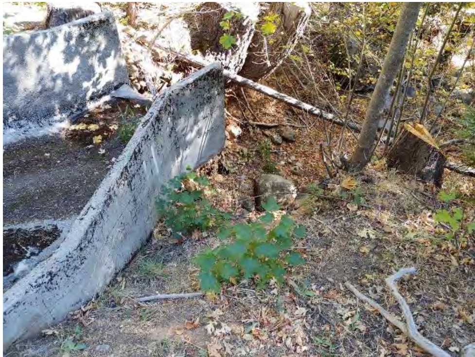
Photo 34 - View of Little Tunnel Spillway
