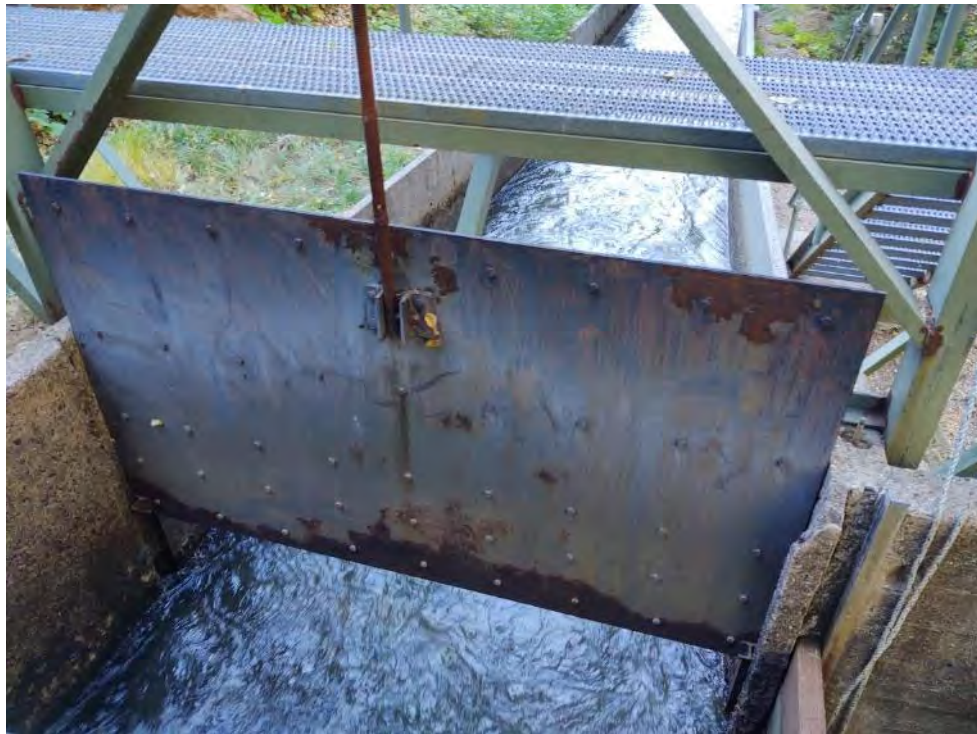
Photo 152 - View of Sand Bunker Spill
