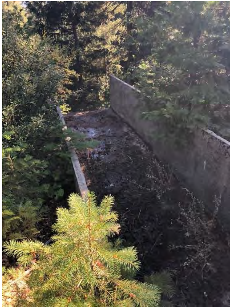
Photo 123 - View of Big Tunnel Side Spill
