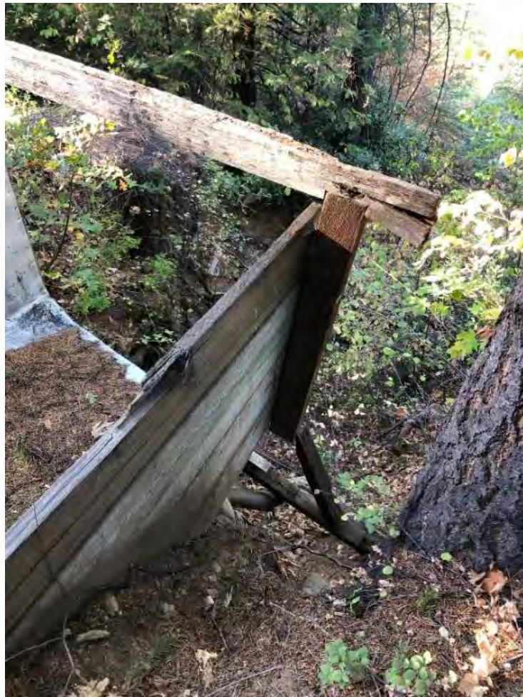
Photo 166 - View of Yunks Spill
