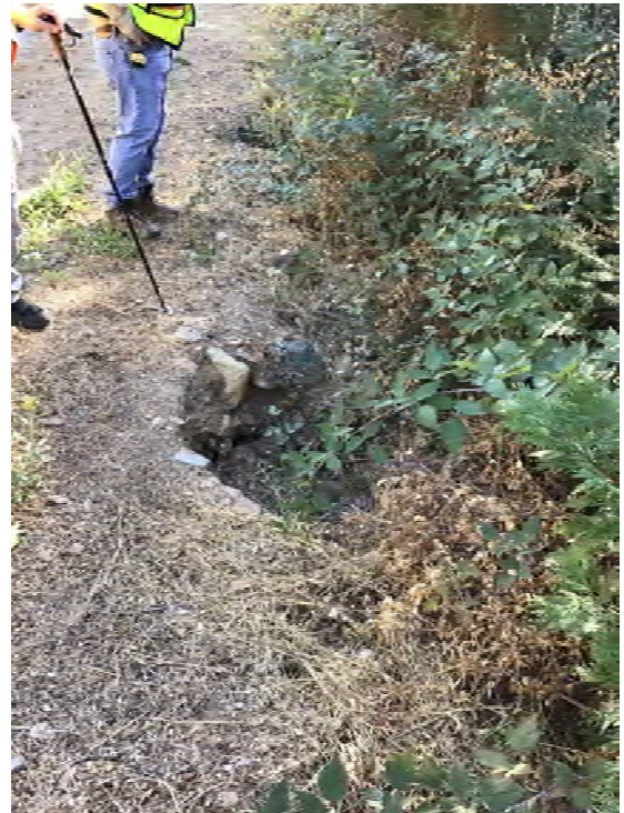
Photo 15 Erosion and Voids in Bench
