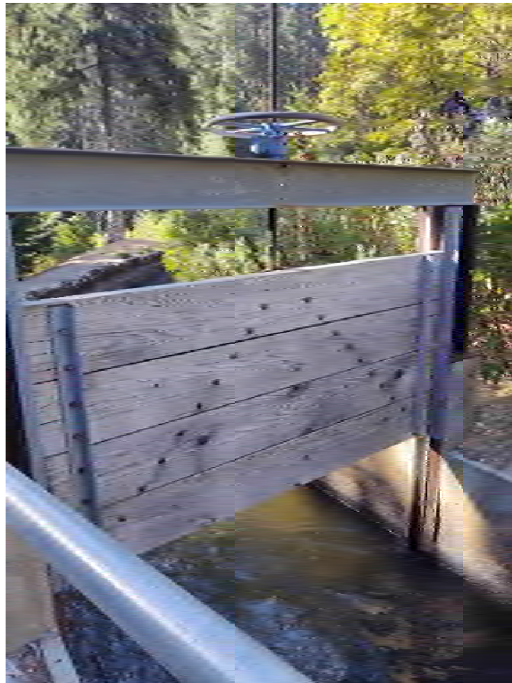
Photo 128 - View of Big Tunnel Side Spill
