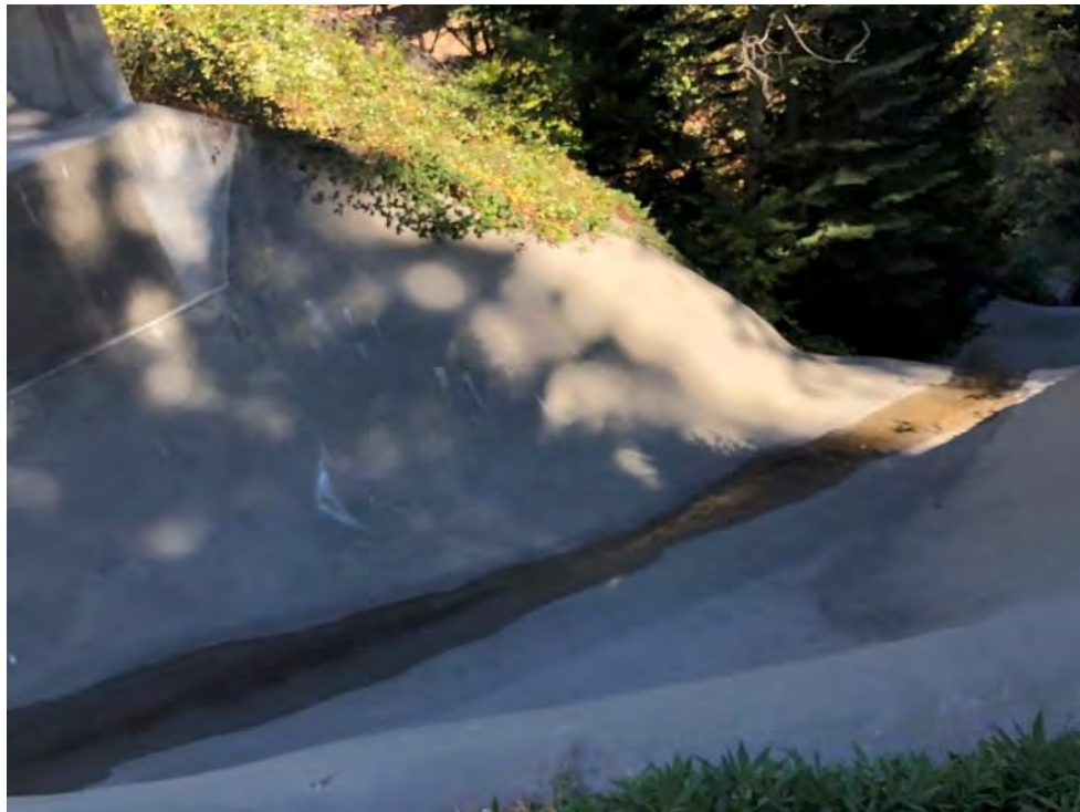
Photo 139 - View of Big Tunnel Spillway
