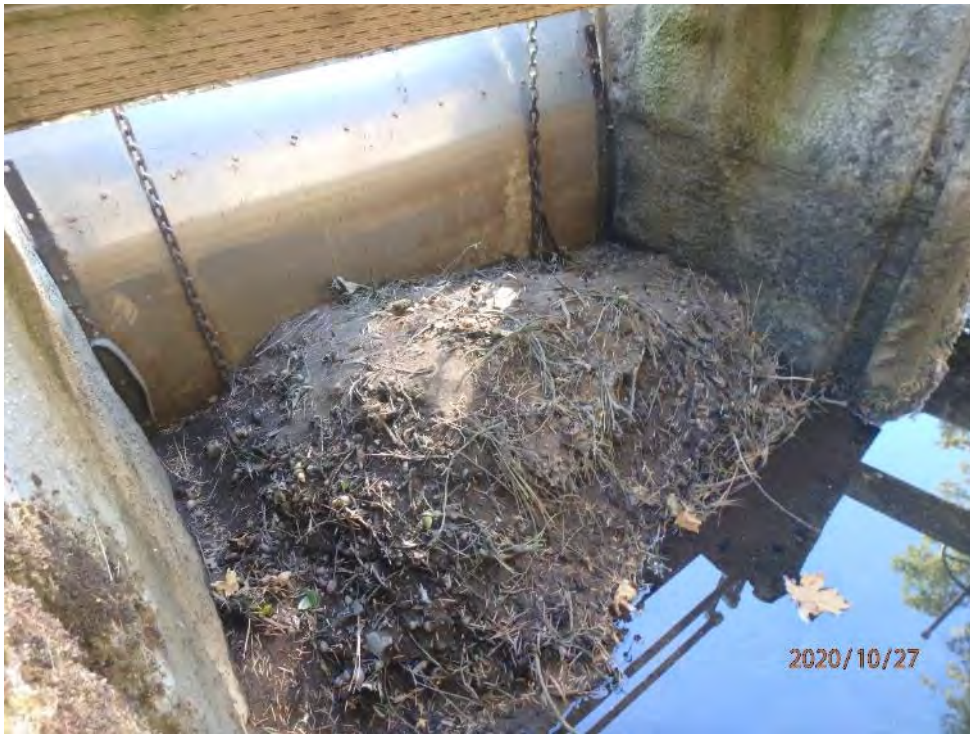
Photo 41 - View of Little Tunnel Spillway
