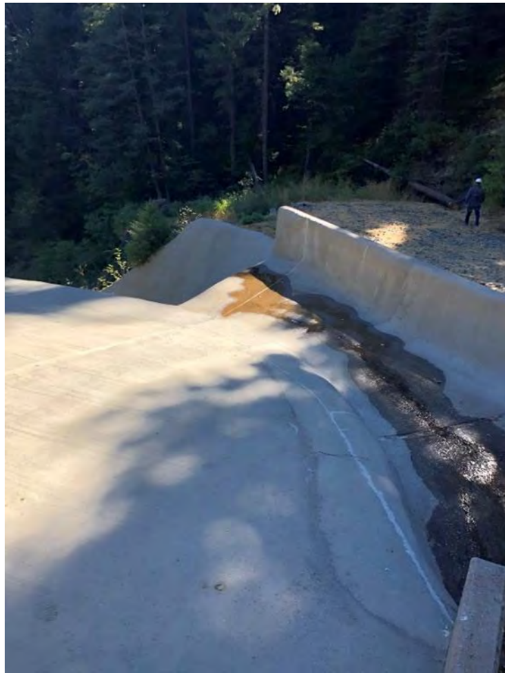
Photo 138 - View of Big Tunnel Spillway
