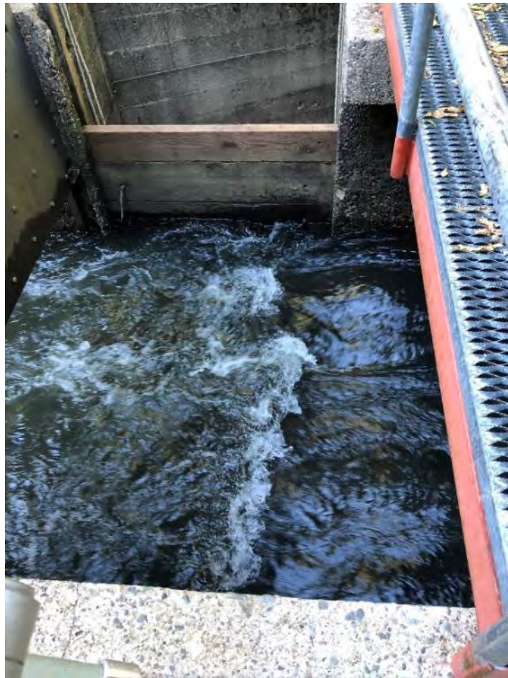
Photo 147 - View of Sand Bunker Spill
