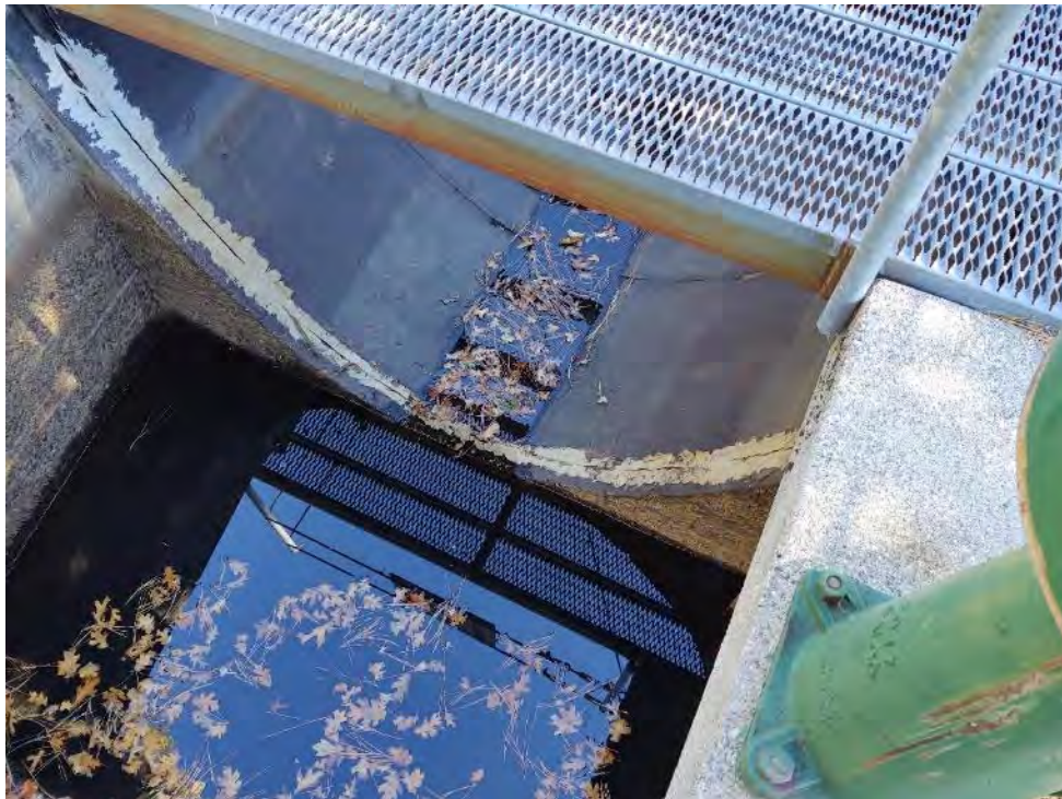
Photo 8 - View of Bear Valley Spillway
