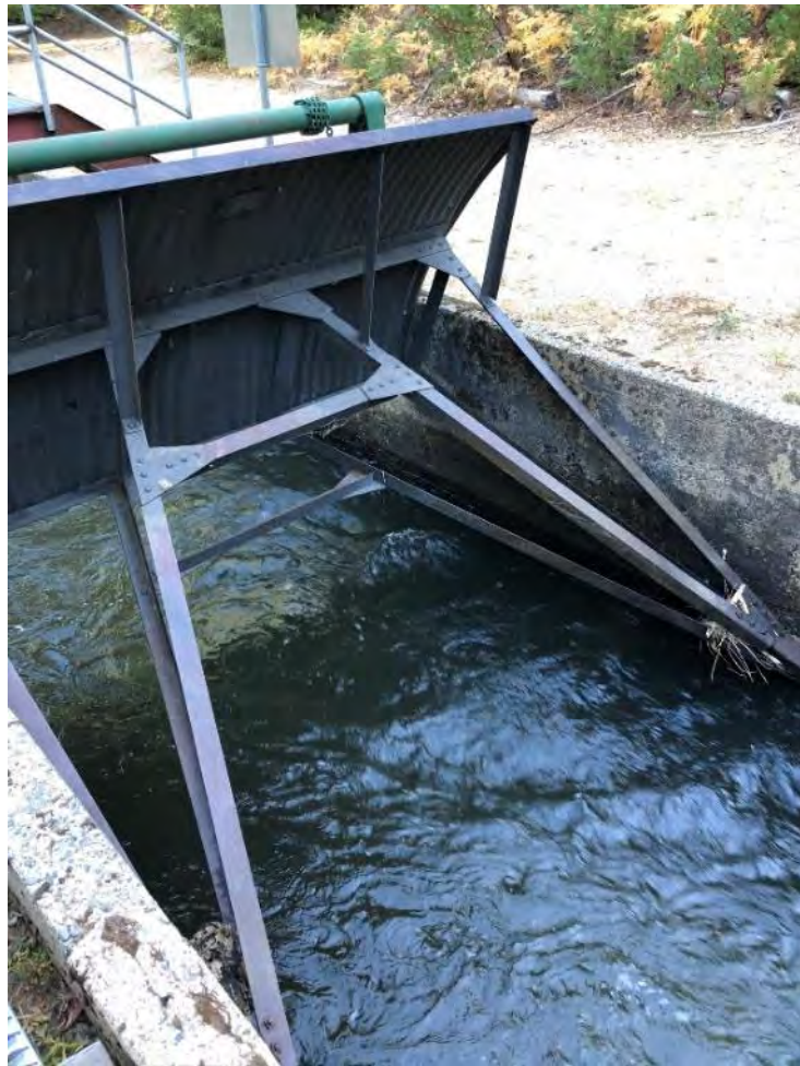
Photo 159 - View of Sandsettler Spillway
