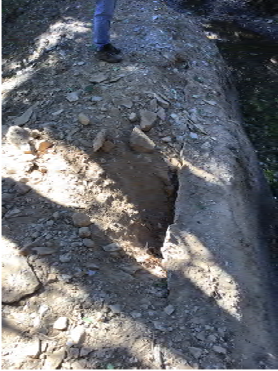
Photo 12 Minor Erosion behind Liner
