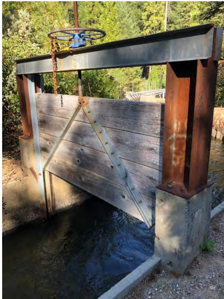
Photo 125 - View of Big Tunnel Side Spill
