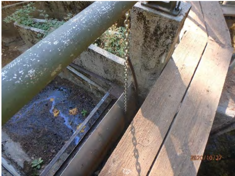
Photo 43 - View of Little Tunnel Spillway
