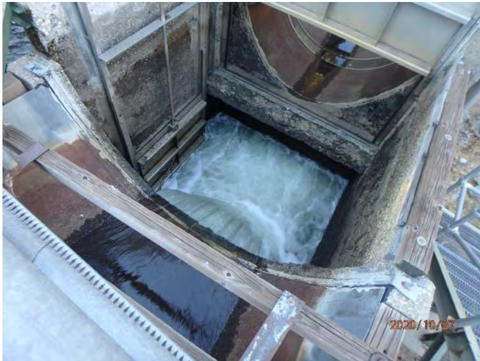
Photo 2 - View of YB139 Spillway
