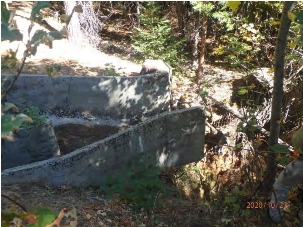
Photo 48 - View of Little Tunnel Spillway
