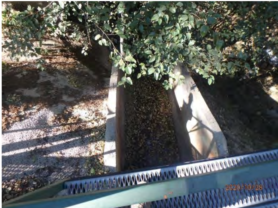
Photo 113 - View of 13 Mile Spillway
