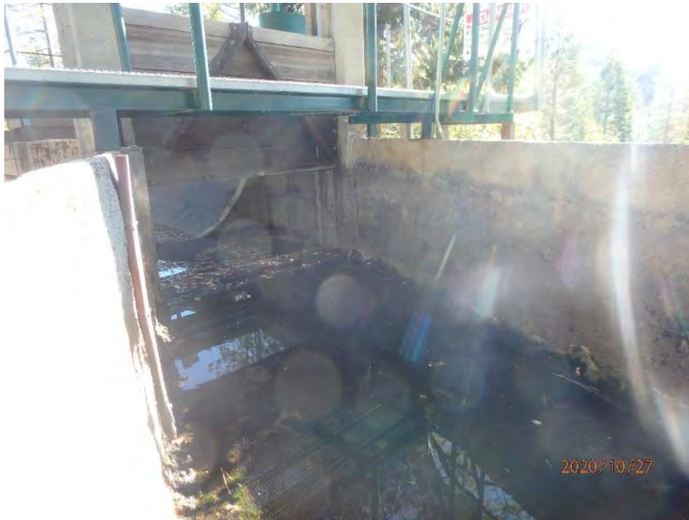
Photo 18 - View of Bear Valley Spillway
