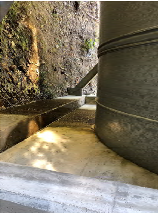
Photo 32 Leakage in Liner at Transition
