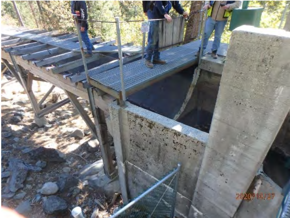
Photo 17 - View of Bear Valley Spillway
