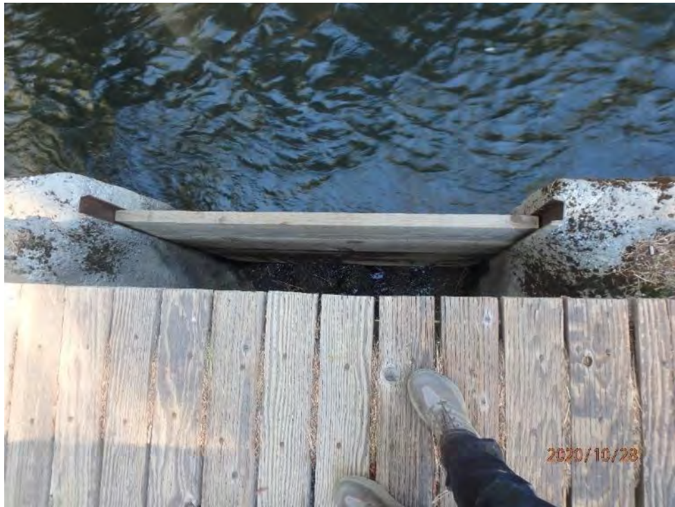
Photo 78 - View of Hickman Spill
