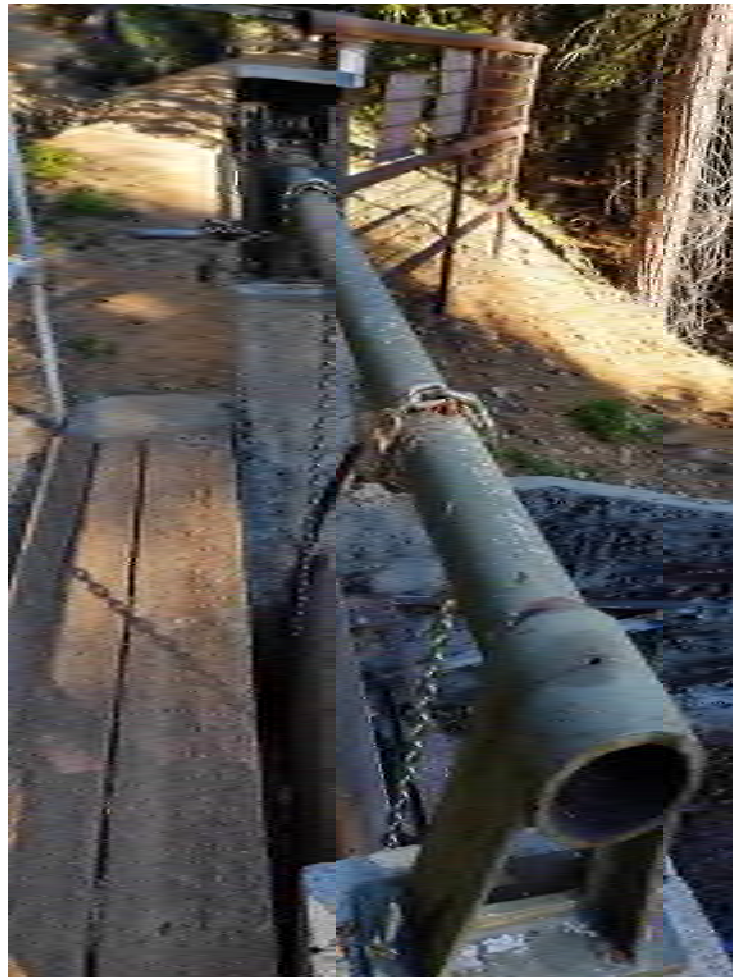
Photo 33 - View of Little Tunnel Spillway
