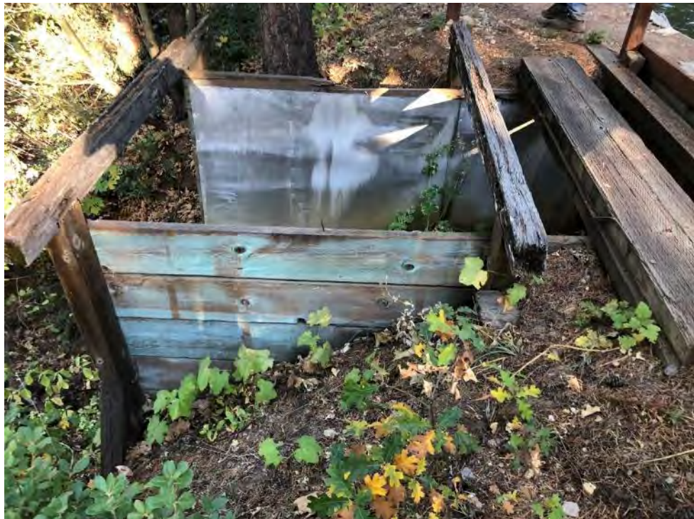
Photo 165 - View of Yunks Spill
