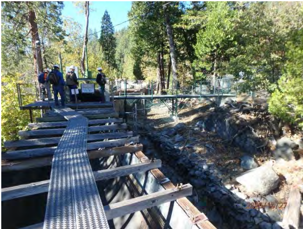
Photo 14 - View of Bear Valley Spillway
