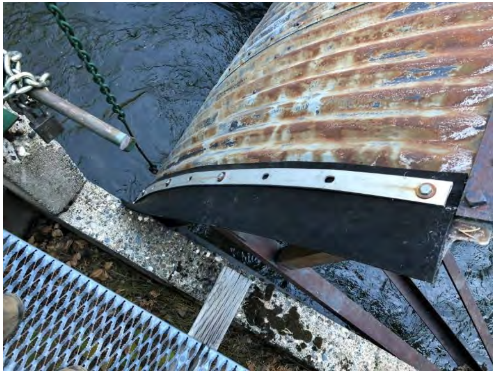
Photo 160 - View of Sandsettler Spillway
