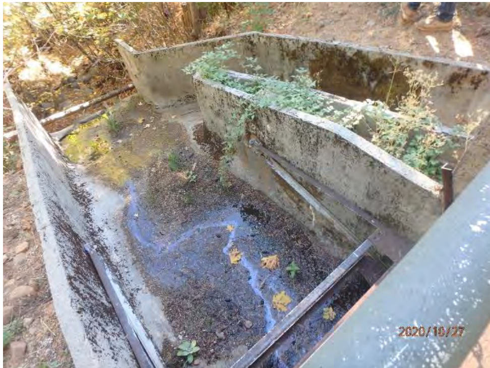
Photo 44 - View of Little Tunnel Spillway
