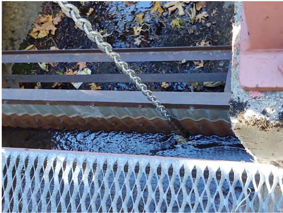
Photo 95 - View of Excelsior Point Gated Spillway
