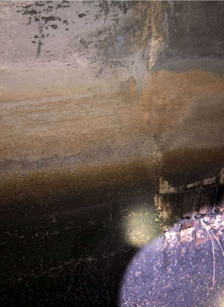
Little Tunnel Liner Thin Cover On Timber
