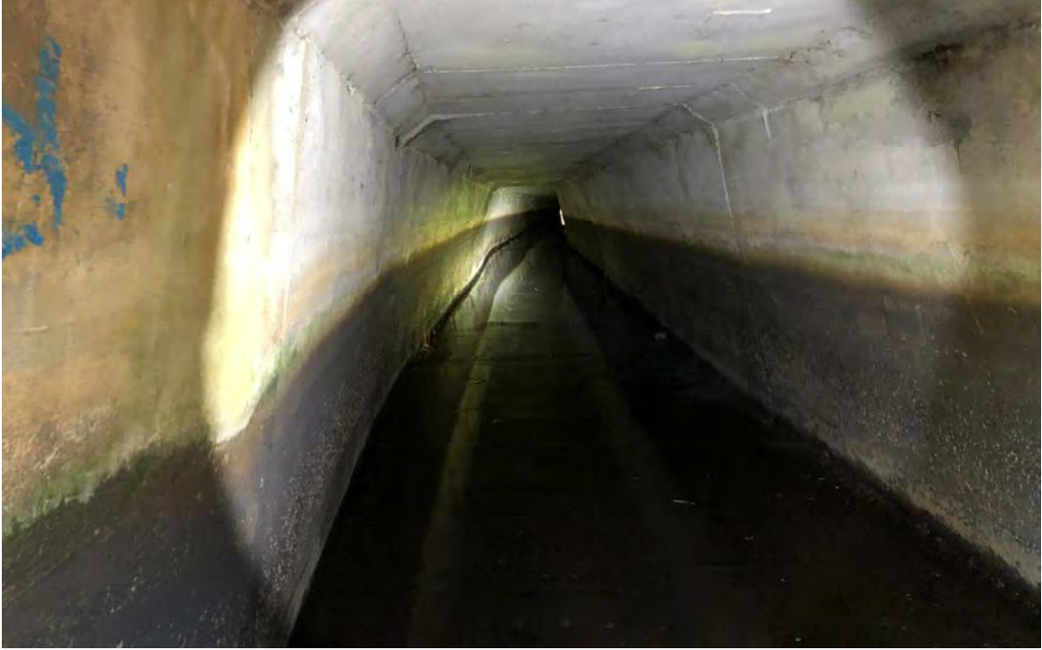
Little Tunnel Liner 3+60 (3)
