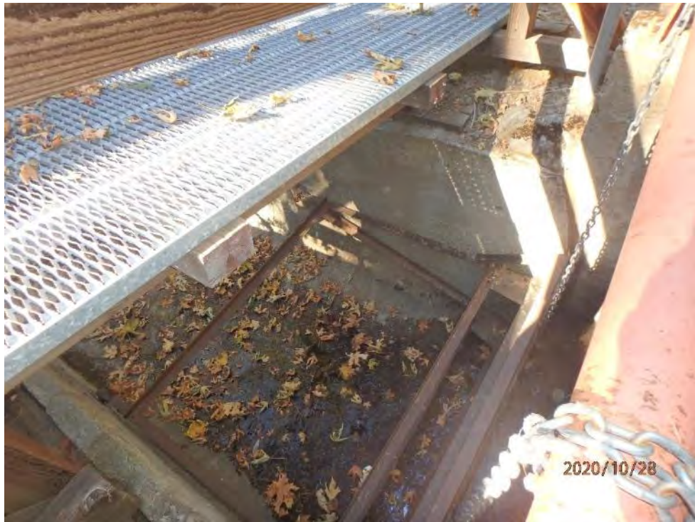
Photo 99 - View of Excelsior Point Gated Spillway
