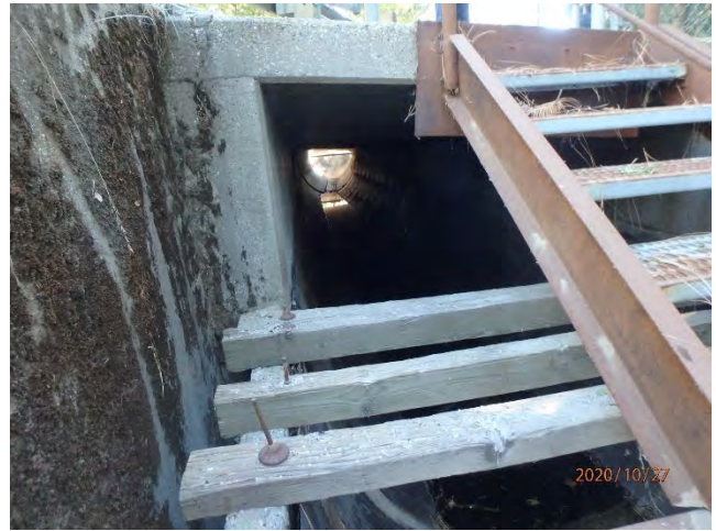
Photo 6 Culvert under Highway 20
