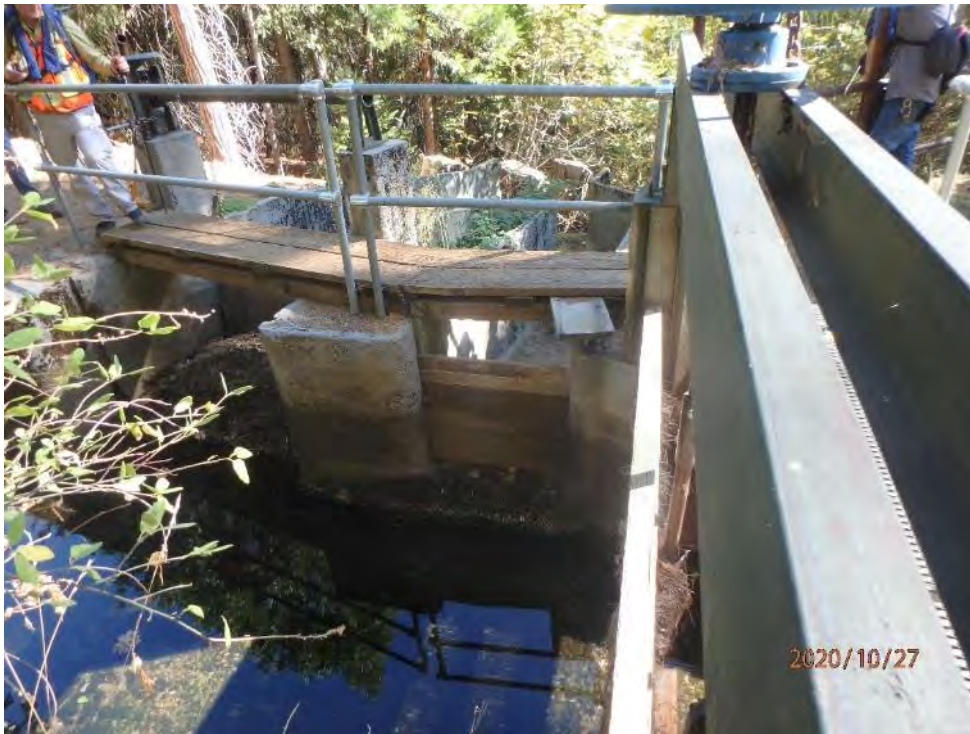
Photo 47 - View of Little Tunnel Spillway
