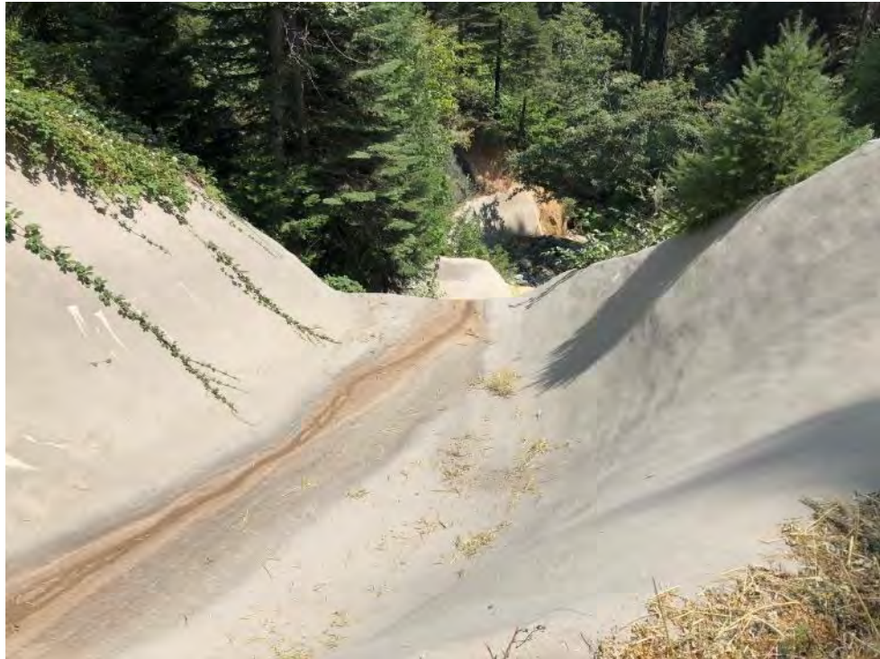
Photo 132 - View of Big Tunnel Spillway
