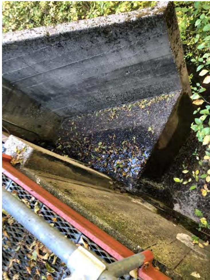
Photo 148 - View of Sand Bunker Spill
