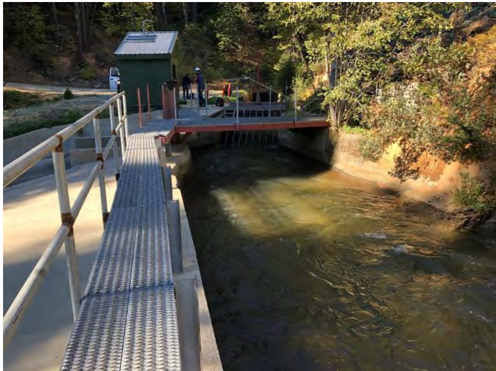
Photo 134 - View of Big Tunnel Spillway
