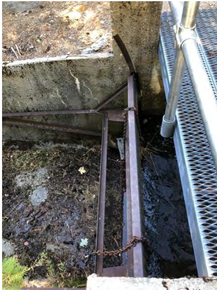
Photo 122 - View of Big Tunnel Side Spill
