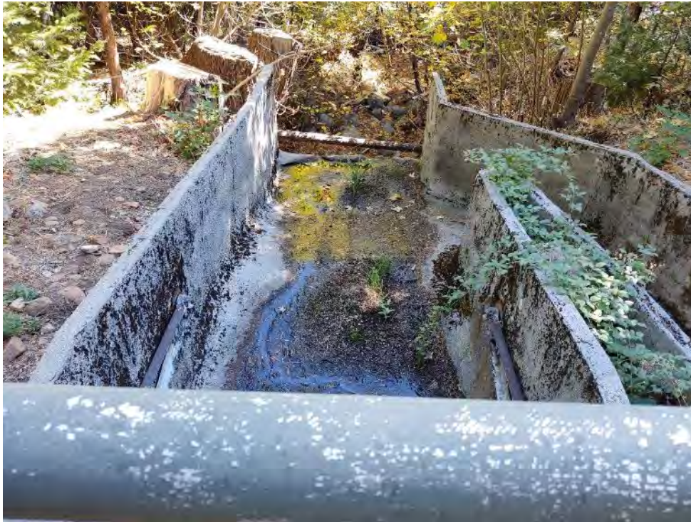
Photo 30 - View of Little Tunnel Spillway
