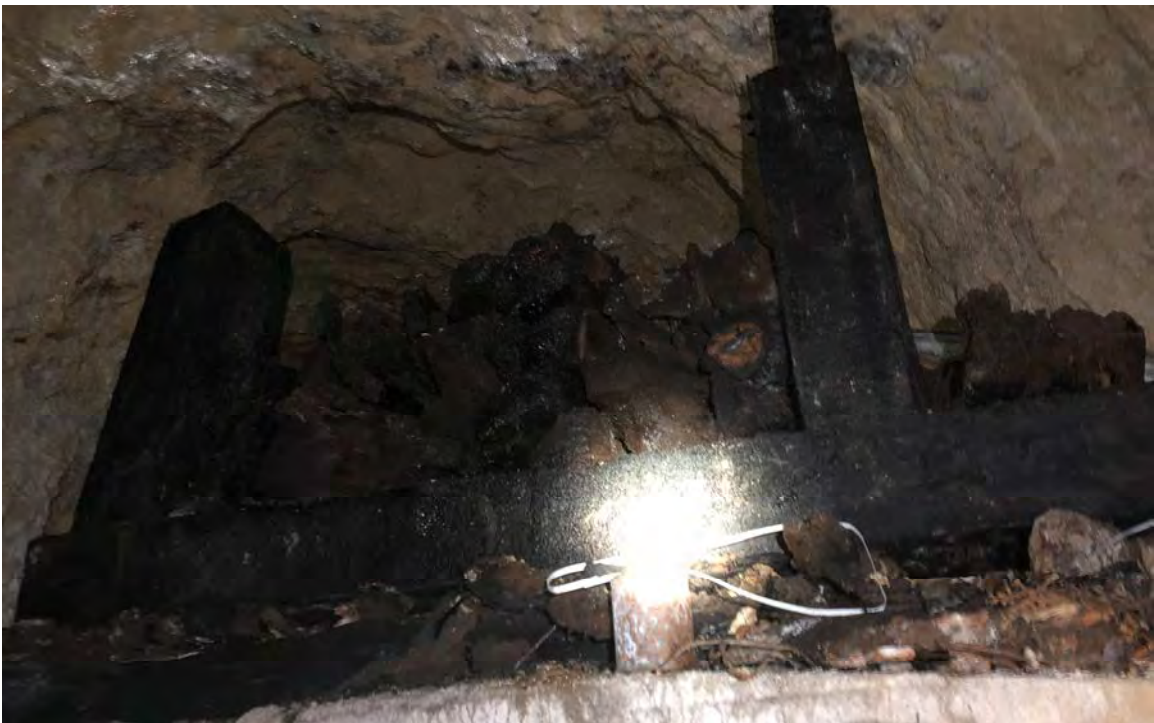
Big Tunnel Timber Crib Above Liner1
