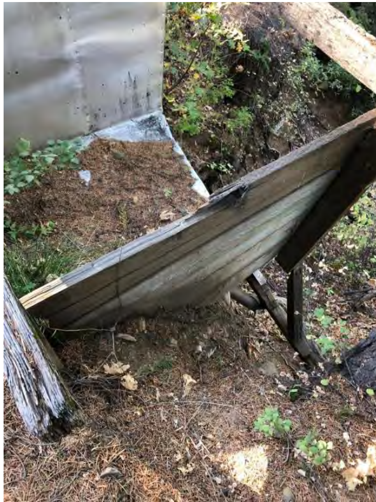
Photo 167 - View of Yunks Spill
