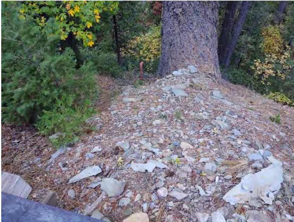
Photo 69 - View of 9 ½ Mile Spill Siphon
