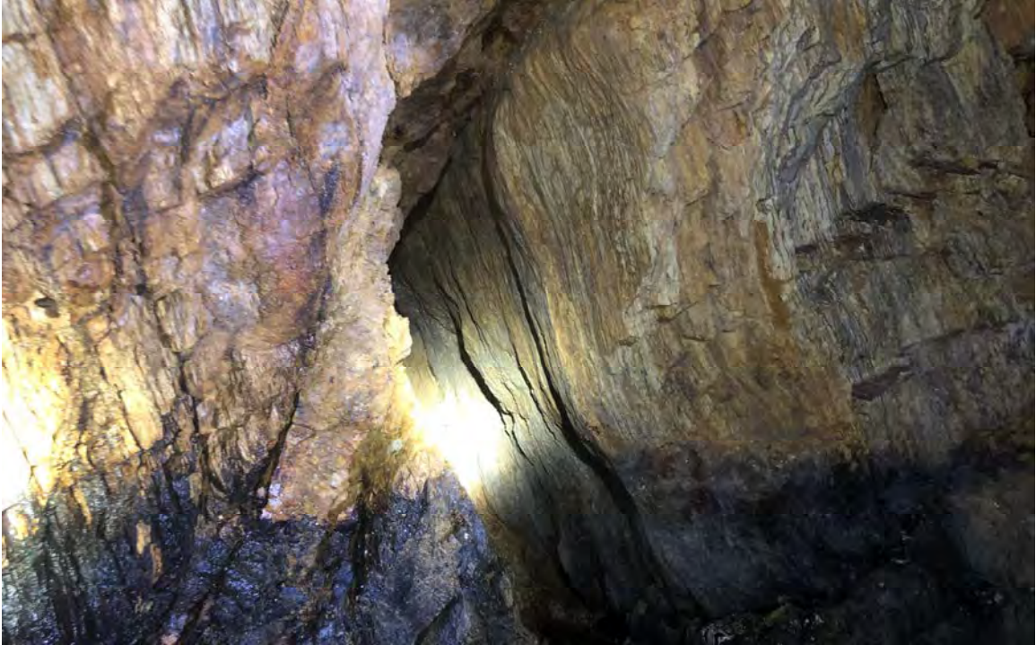
Big Tunnel 19+91 Shear1
