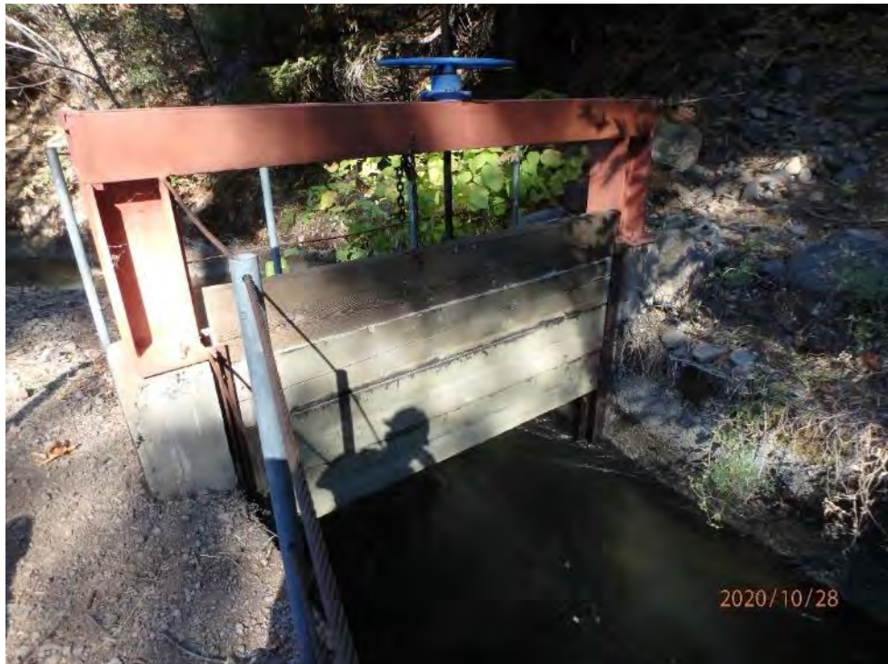
Photo 100 - View of Excelsior Point Gated Spillway
