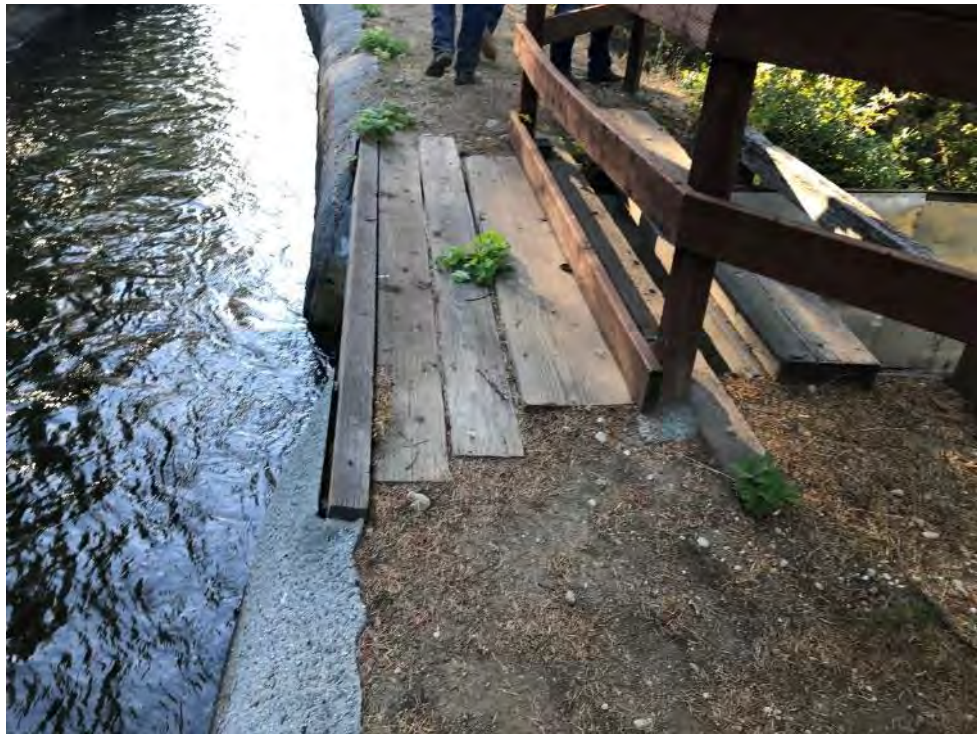
Photo 162 - View of Yunks Spill
