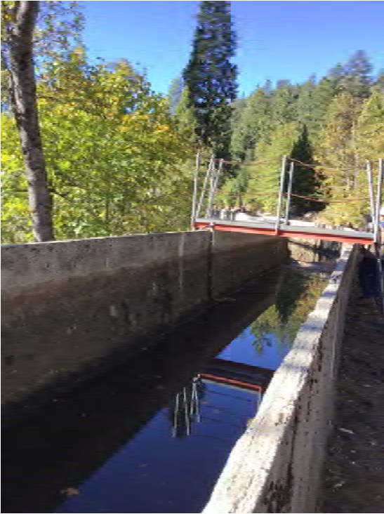
Photo 10 Typical Concrete Box
