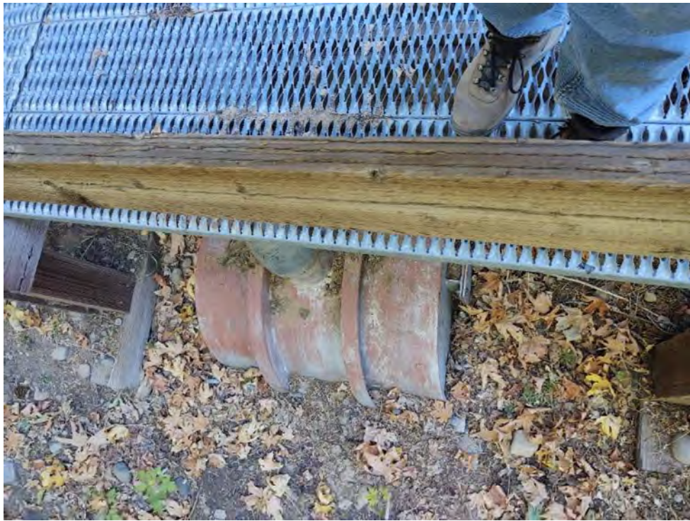
Photo 84 - View of Excelsior Point Spill Siphon
