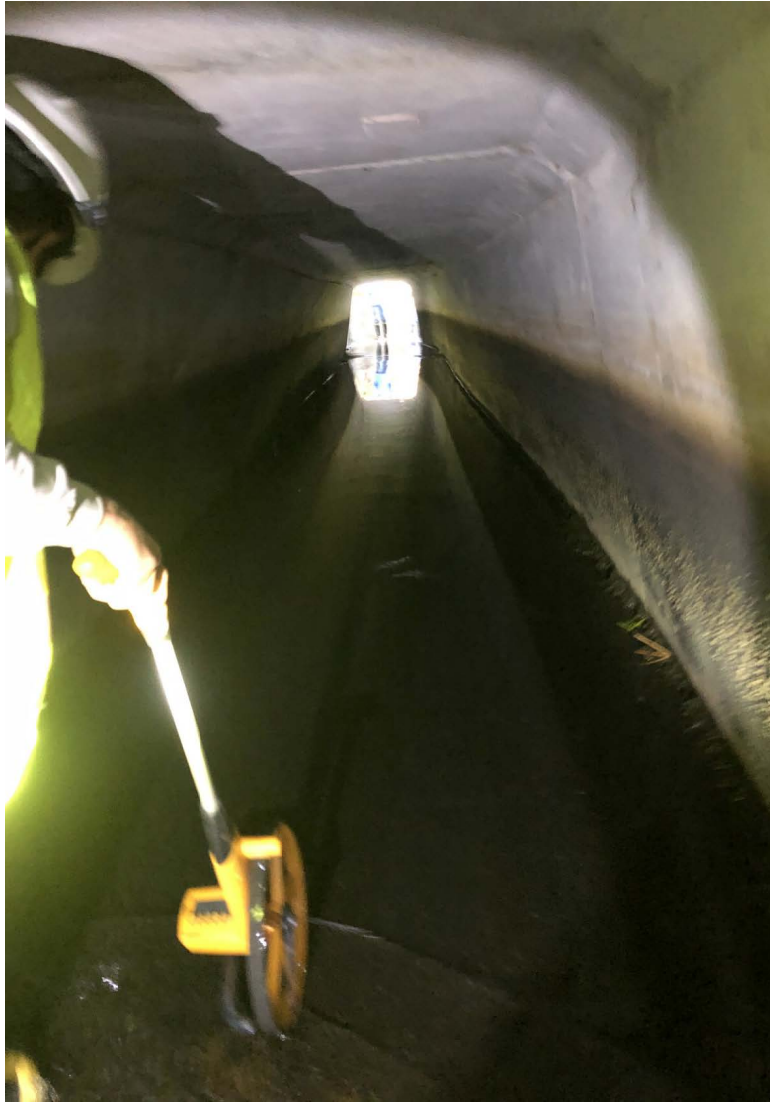
Little Tunnel Liner
