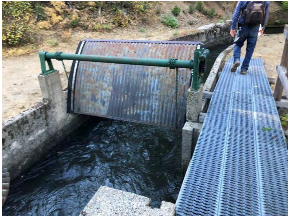
Photo 158 - View of Sandsettler Spillway
