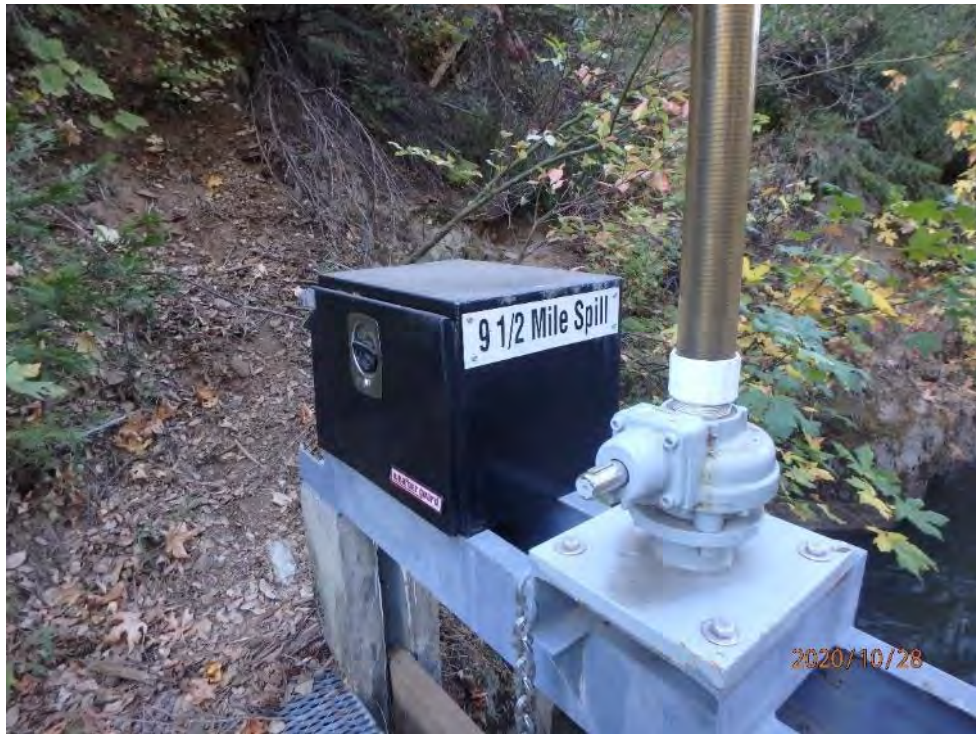
Photo 59 - View of 9 1/2 Mile Spill
