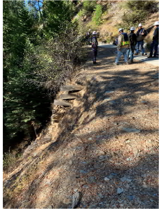
Photo 23 Potential Slope Distress at Hickman Spill
