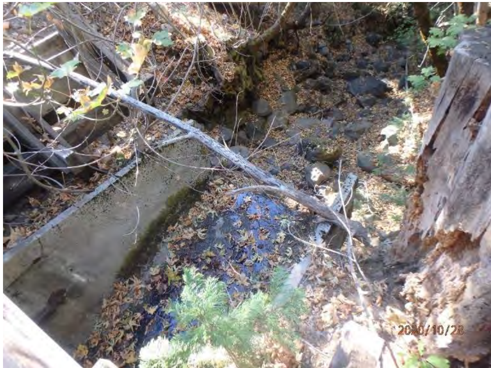
Photo 97 - View of Excelsior Point Gated Spillway
