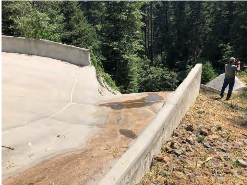
Photo 131 - View of Big Tunnel Spillway
