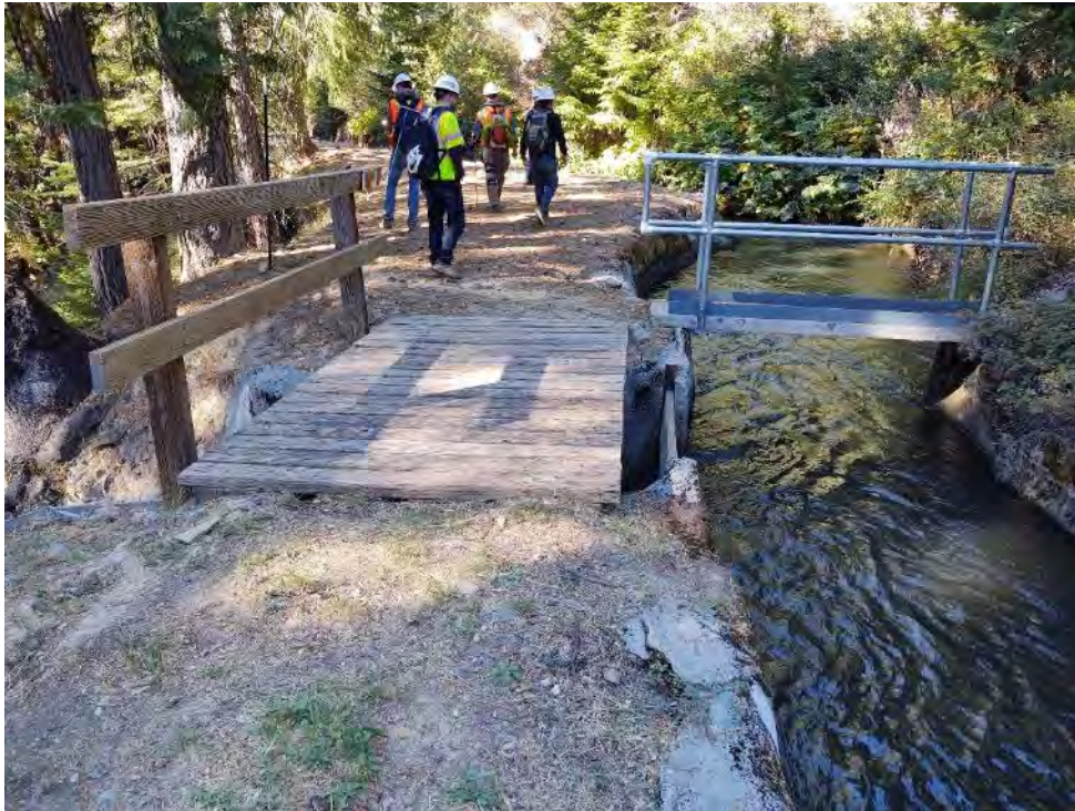
Photo 76 - View of Hickman Spill
