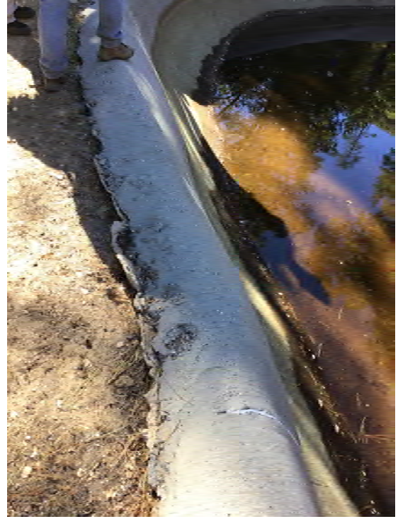
Photo 13 Minor Cracking in Liner
