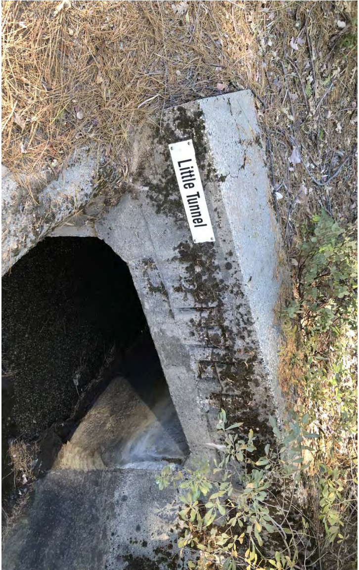
Little Tunnel Upstream Portal
