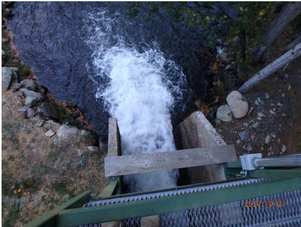
Photo 3 - View of YB139 Spillway
