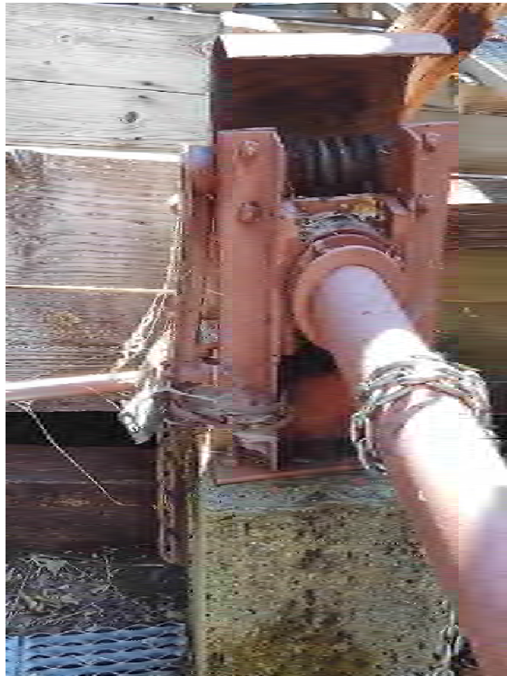
Photo 94 - View of Excelsior Point Gated Spillway
