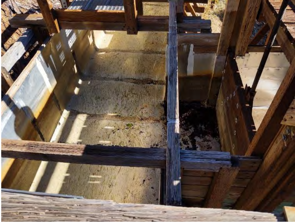
Photo 22 - View of Capehorn Spillway
