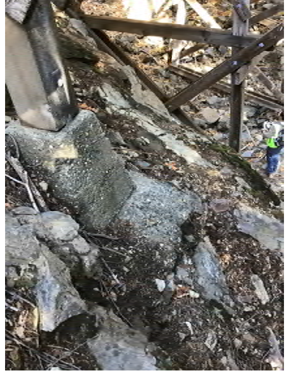
Photo 2 Minor Erosion at Foundation
