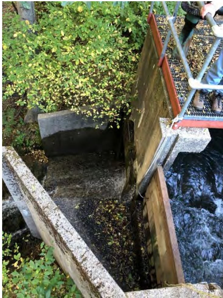
Photo 150 - View of Sand Bunker Spill
