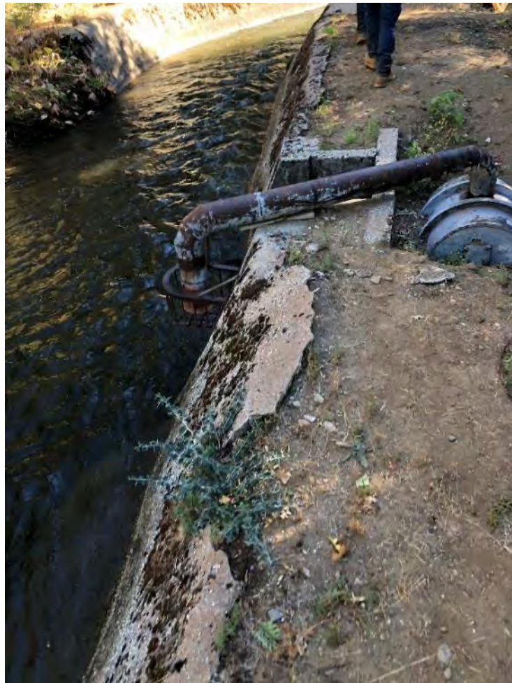
Photo 154 - View of Siphon Upstream of Sandsettler Spill Siphon
