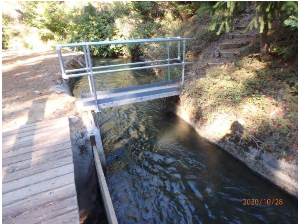
Photo 77 - View of Hickman Spill
