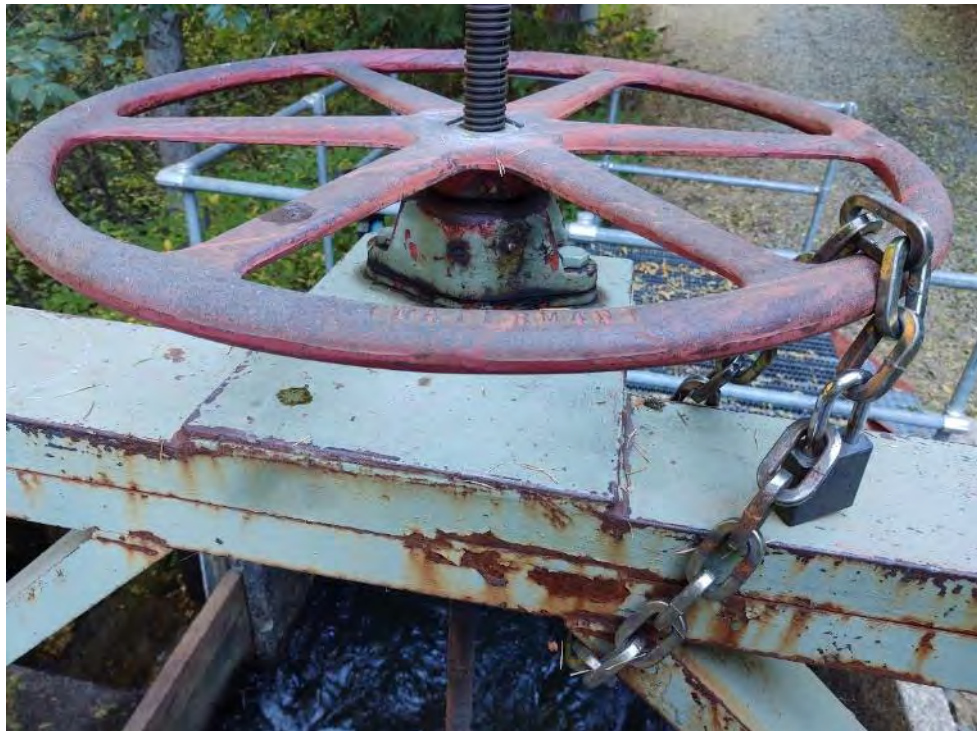
Photo 153 - View of Sand Bunker Spill
