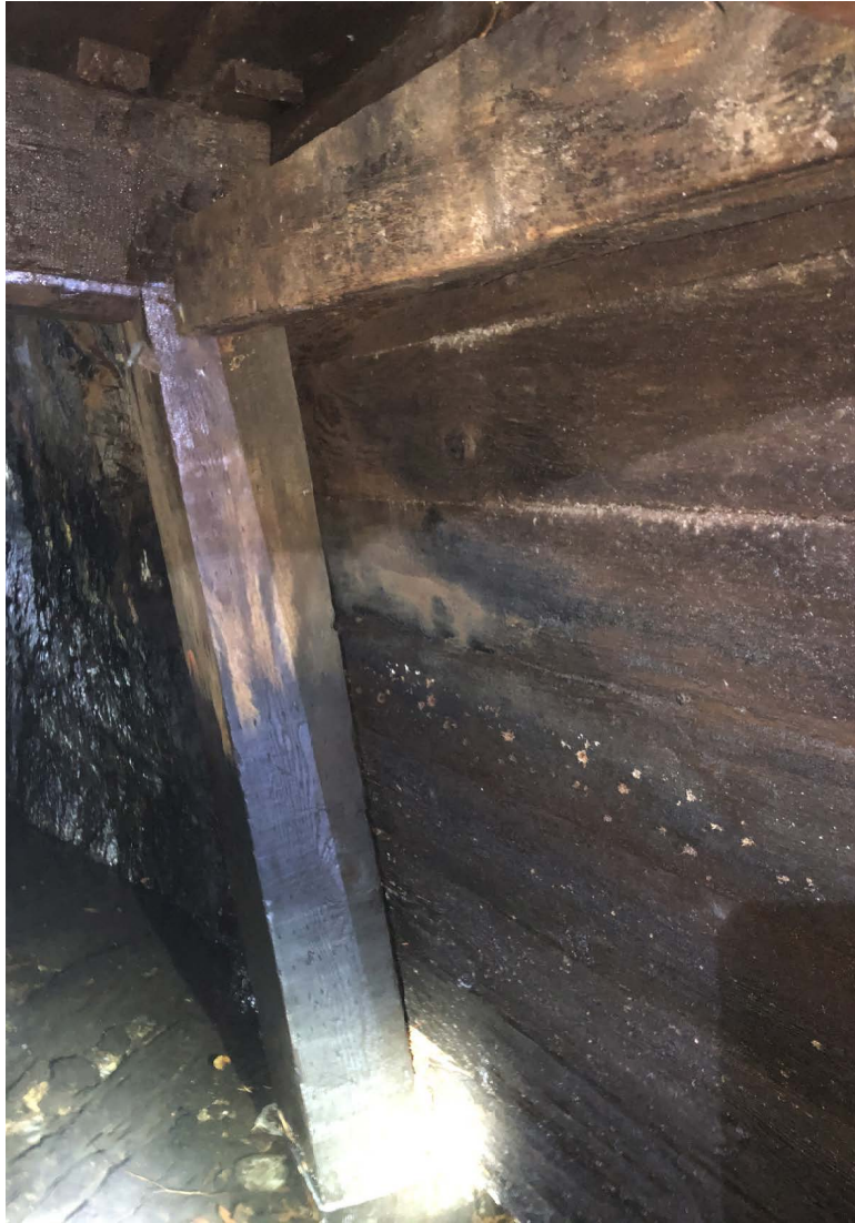
Big Tunnel Timber Sets 5+70
