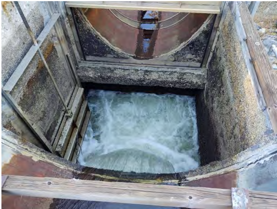
Photo 1 - View of YB139 Spillway
