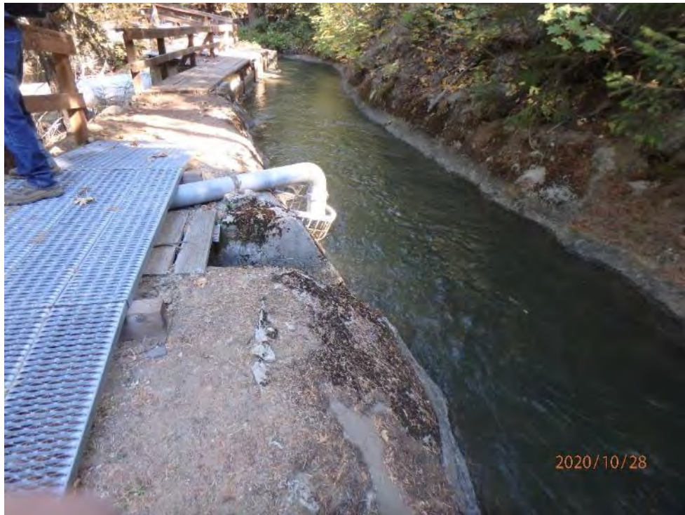
Photo 86 - View of Excelsior Point Spill Siphon
