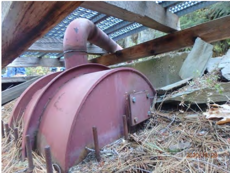
Photo 72 - View of 9 ½ Mile Spill Siphon
