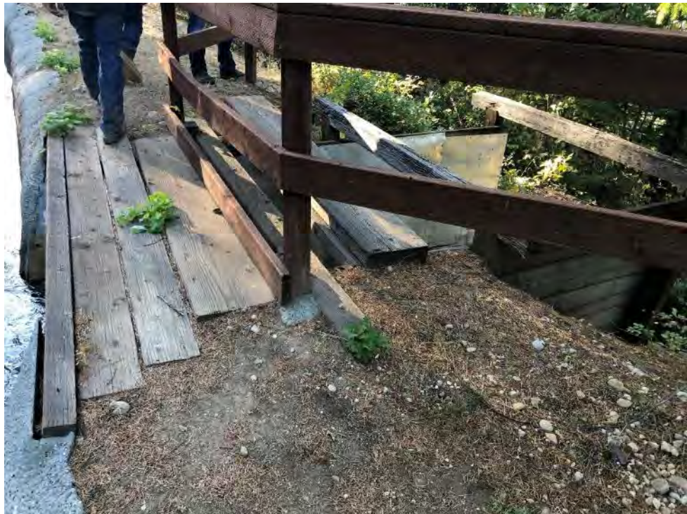
Photo 161 - View of Yunks Spill
