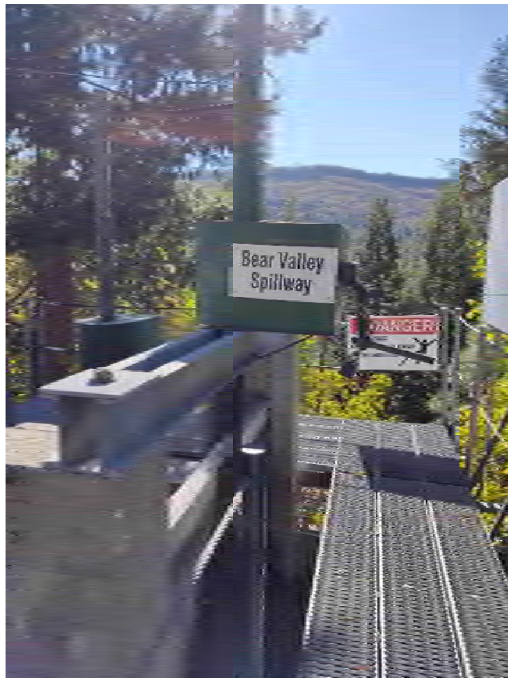
Photo 13 - View of Bear Valley Spillway
