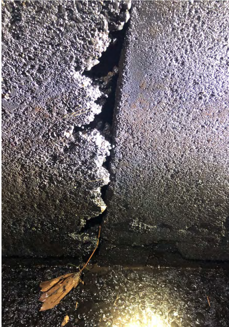
Big Tunnel Construction Joint
