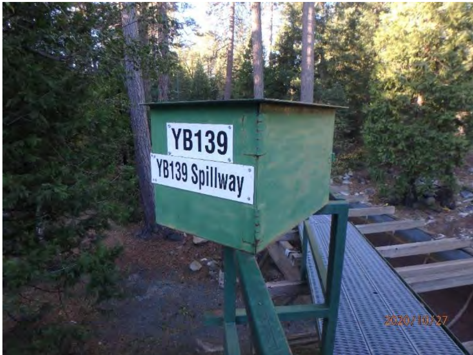
Photo 4 - View of YB139 Spillway
