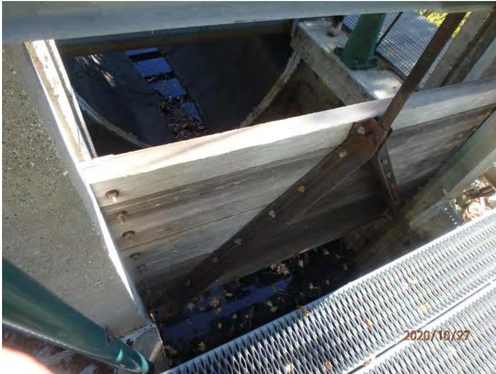
Photo 16 - View of Bear Valley Spillway
