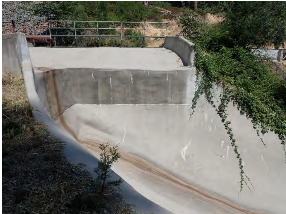
Photo 144 - View of Big Tunnel Spillway
