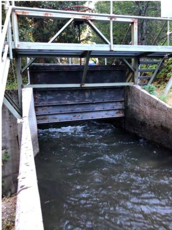
Photo 151 - View of Sand Bunker Spill
