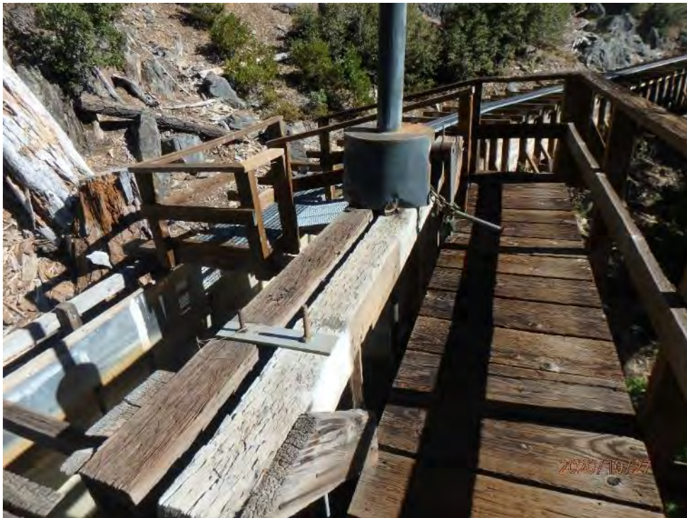
Photo 29 - View of Capehorn Spillway
