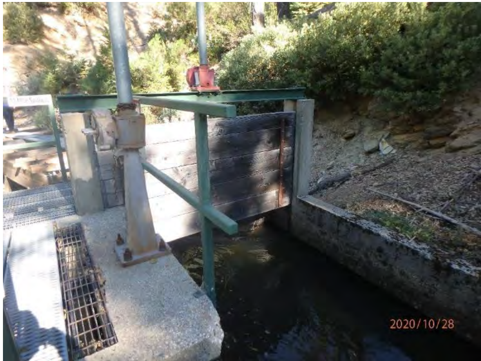
Photo 112 - View of 13 Mile Spillway
