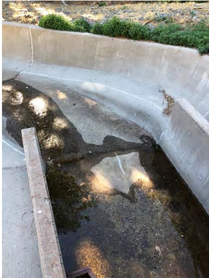
Photo 137 - View of Big Tunnel Spillway
