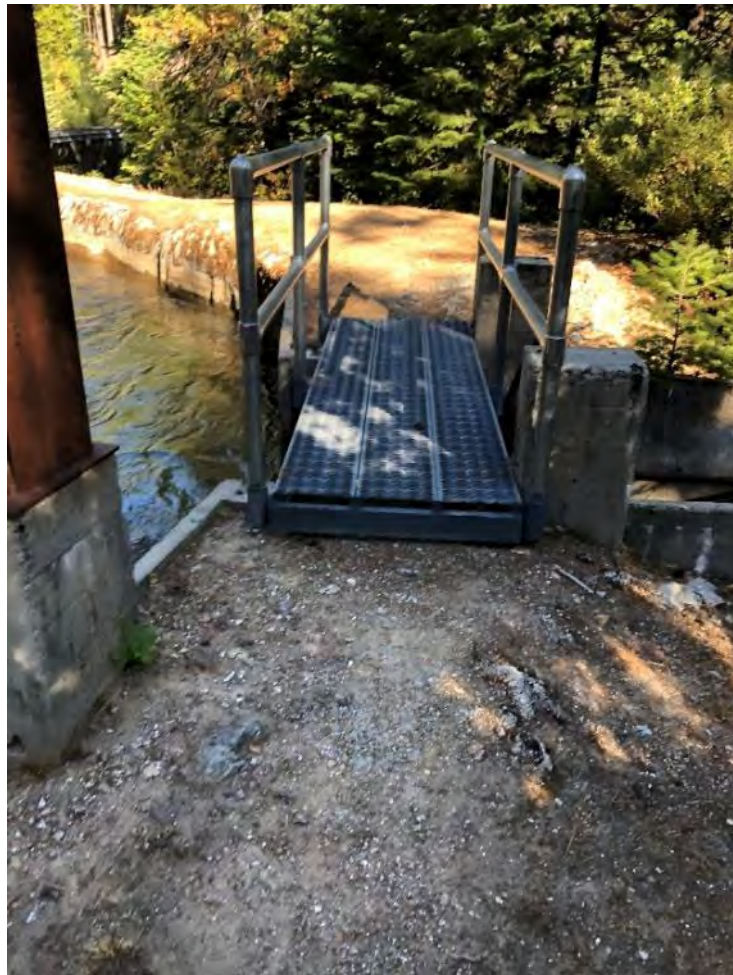
Photo 126 - View of Big Tunnel Side Spill
