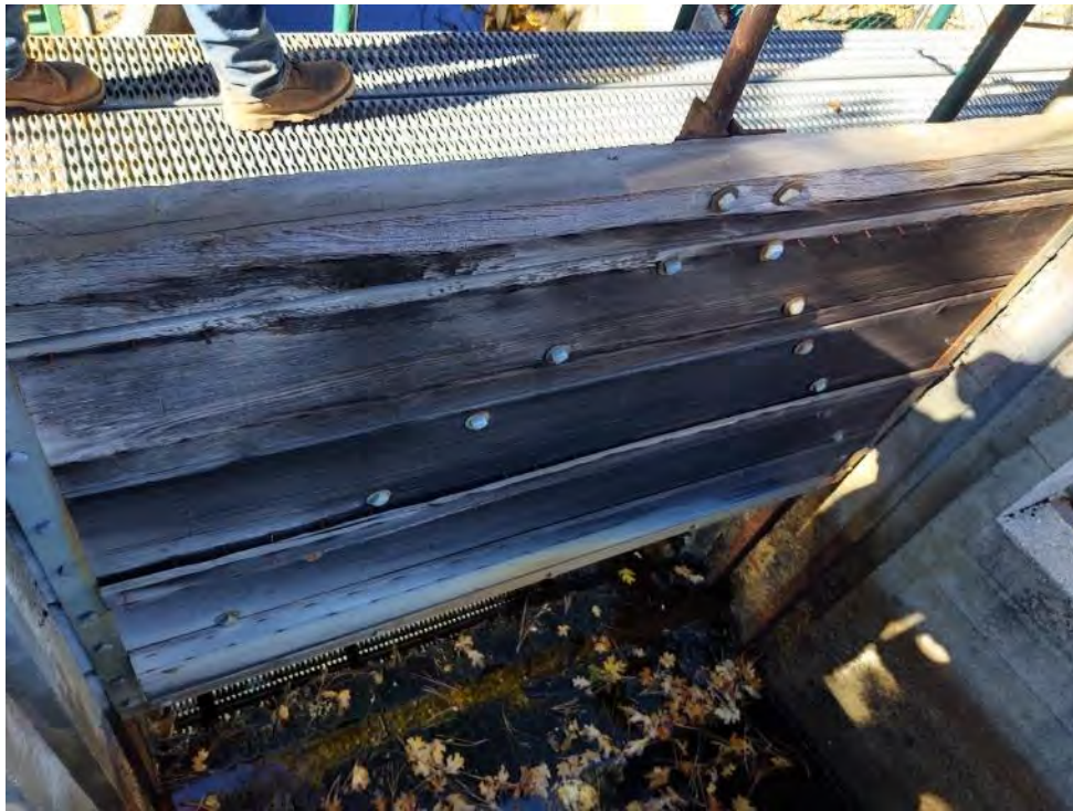
Photo 7 - View of Bear Valley Spillway
