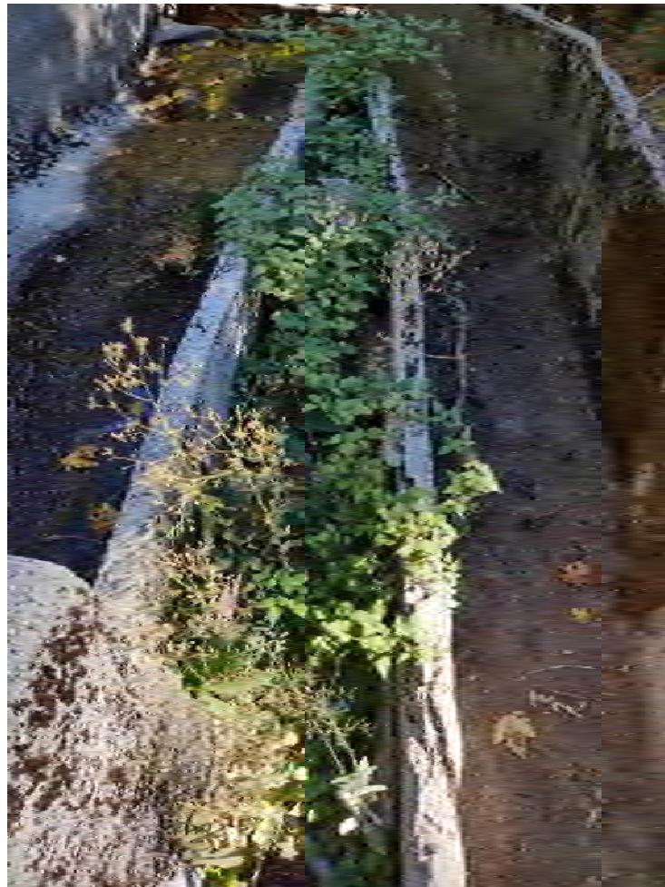
Photo 32 - View of Little Tunnel Spillway
