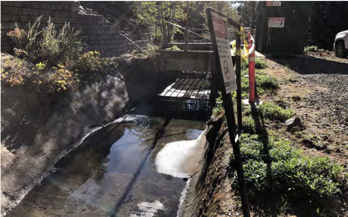
Big Tunnel Upstream
