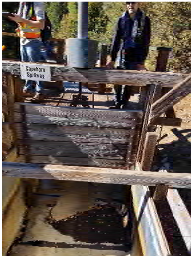
Photo 19 - View of Capehorn Spillway
