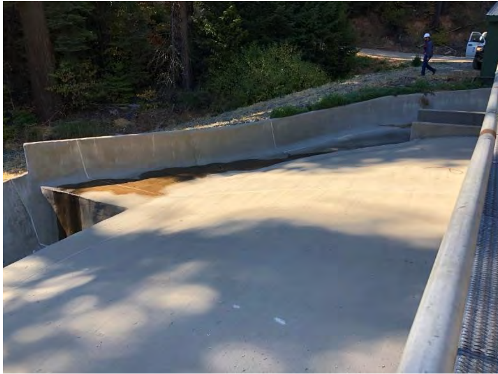
Photo 135 - View of Big Tunnel Spillway
