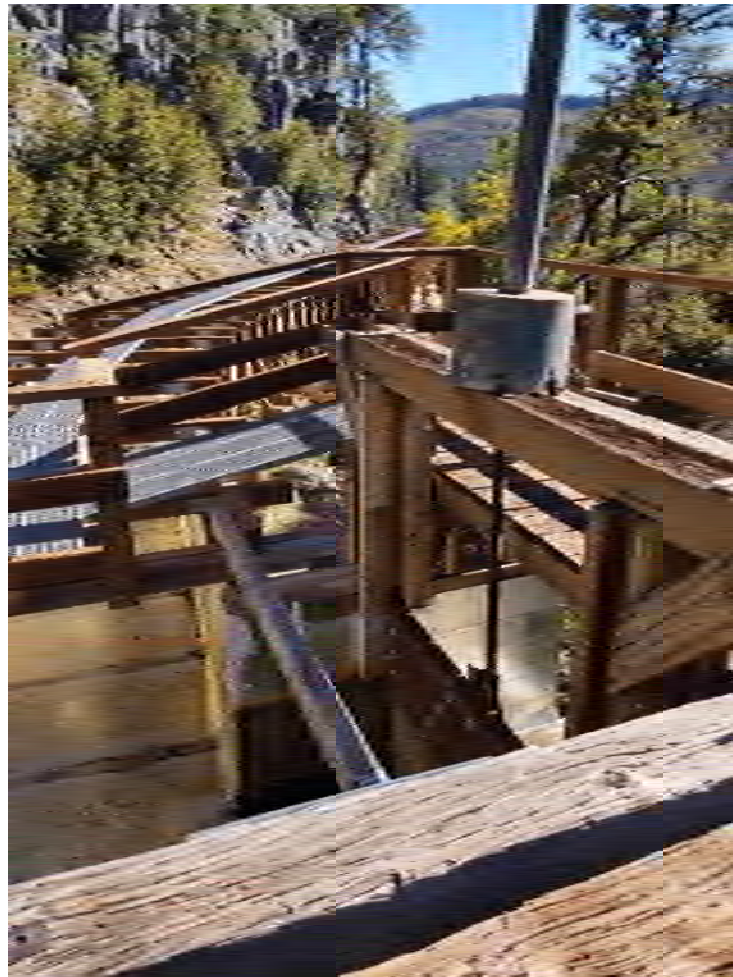
Photo 23 - View of Capehorn Spillway
