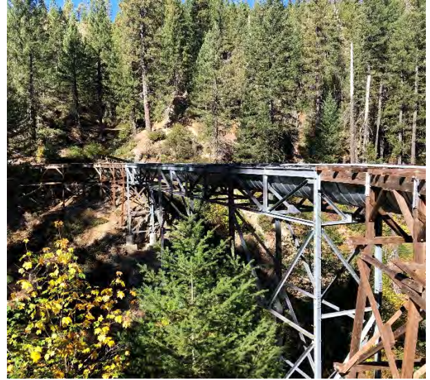
Photo 31 Steep Hollow #2 Lennon Flume
