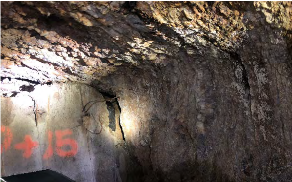
Big Tunnel 19+91 Shear5
