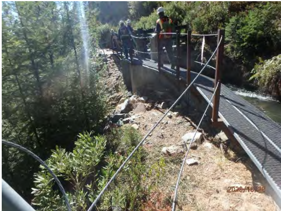
Photo 118 - View of 14 Mile Spill
