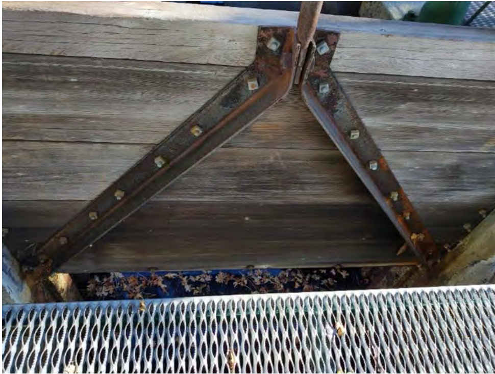
Photo 12 - View of Bear Valley Spillway
