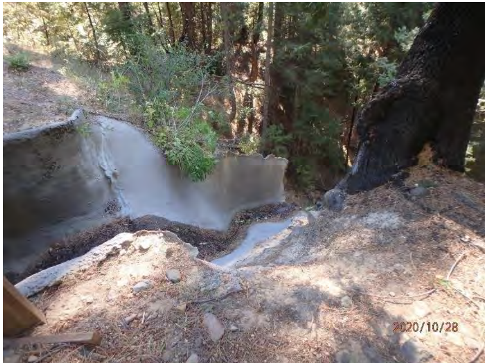
Photo 81 - View of Hickman Spill
