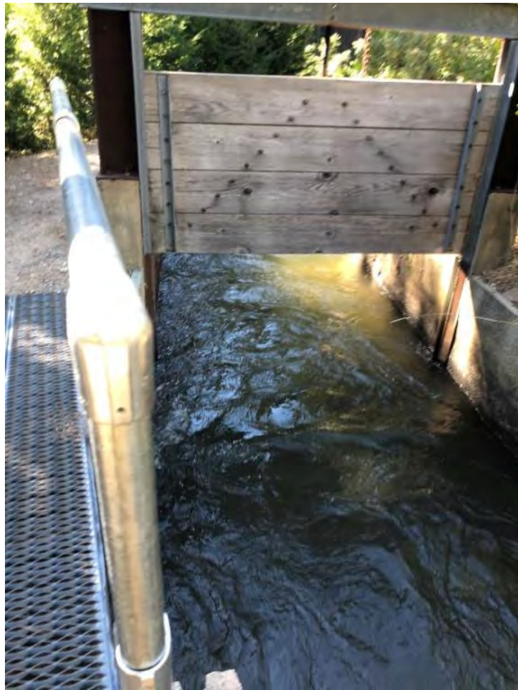
Photo 124 - View of Big Tunnel Side Spill
