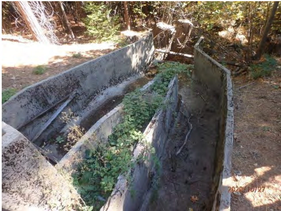
Photo 45 - View of Little Tunnel Spillway
