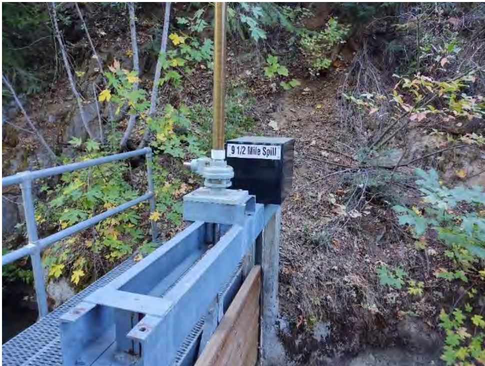
Photo 50 - View of 9 1/2 Mile Spill
