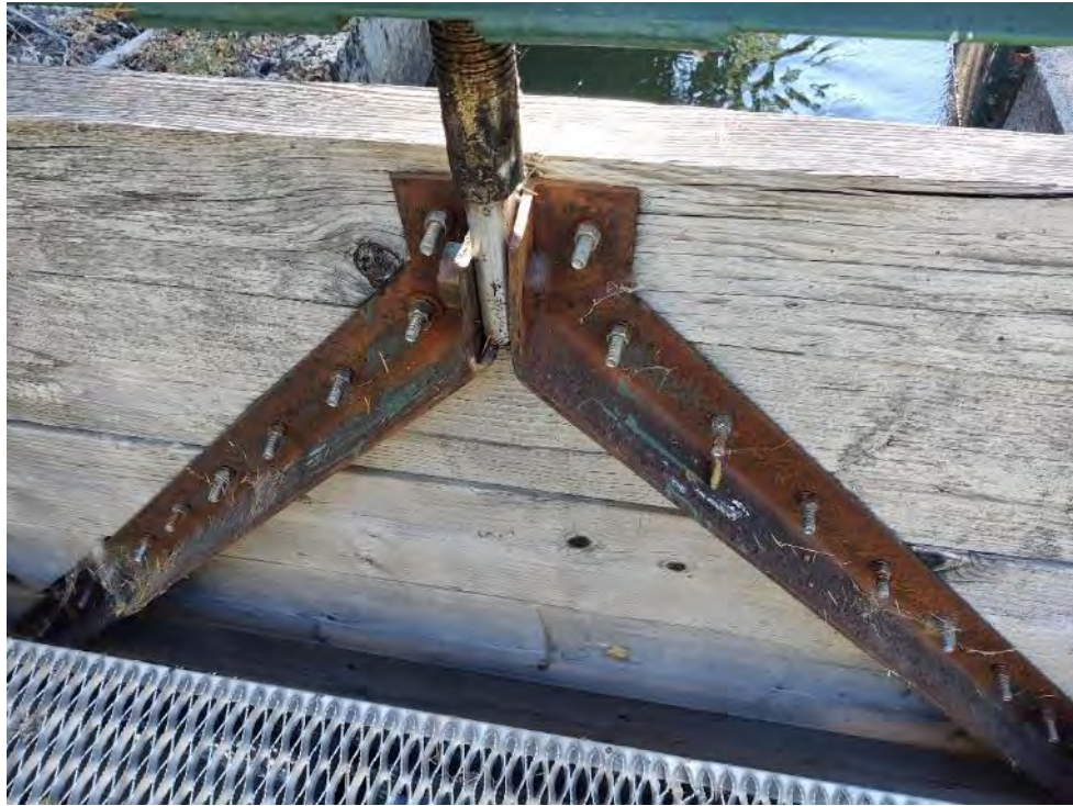
Photo 109 - View of 13 Mile Spillway
