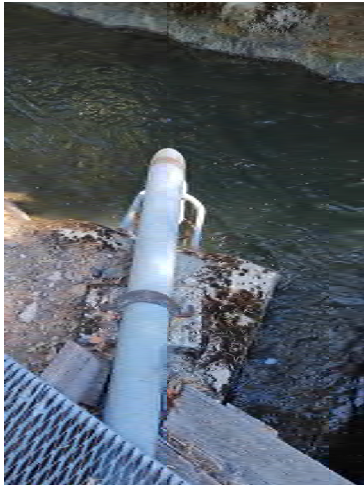
Photo 83 - View of Excelsior Point Spill Siphon
