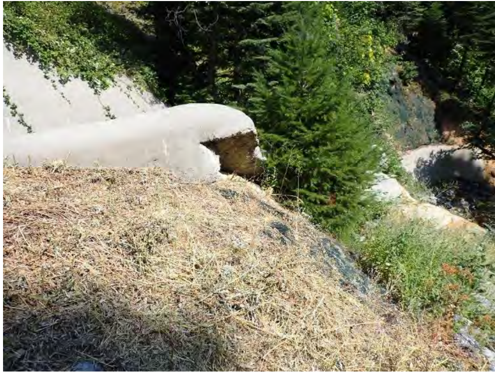
Photo 146 - View of Big Tunnel Spillway
