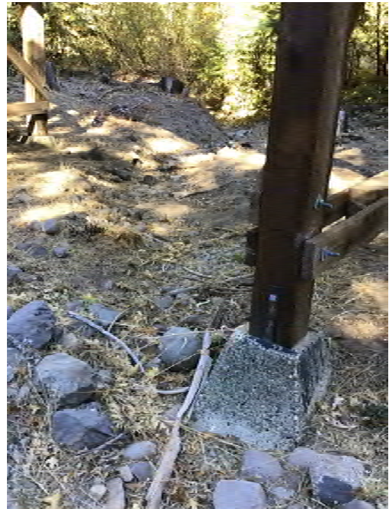
Photo 9 Minor Erosion at Foundation
