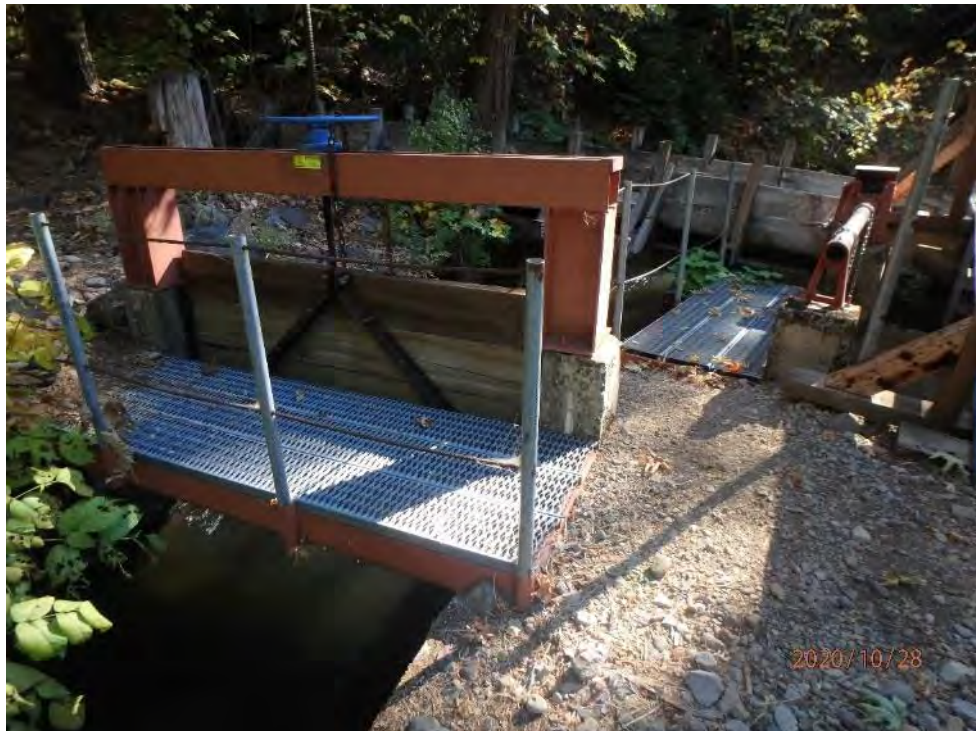
Photo 102 - View of Excelsior Point Gated Spillway
