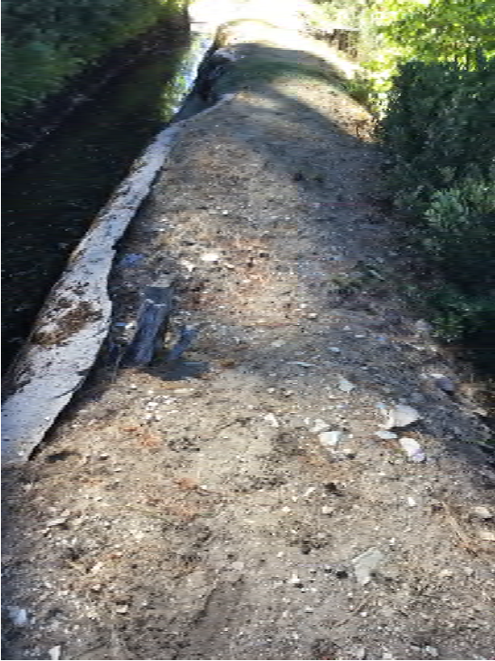
Photo 18 Slump in Bench with Cracking in Canal
