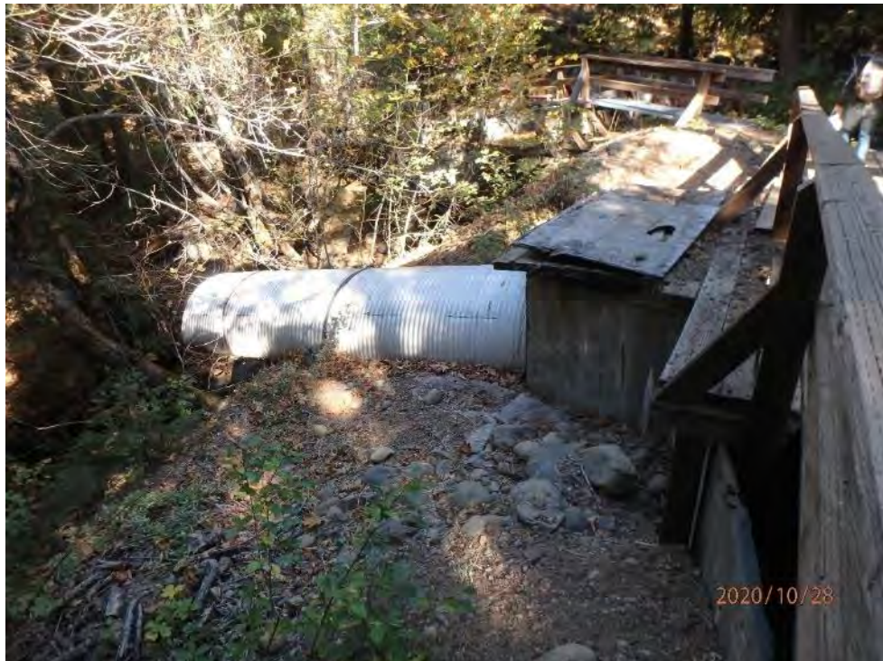
Photo 91 - View of Excelsior Point Flashboard Weir
