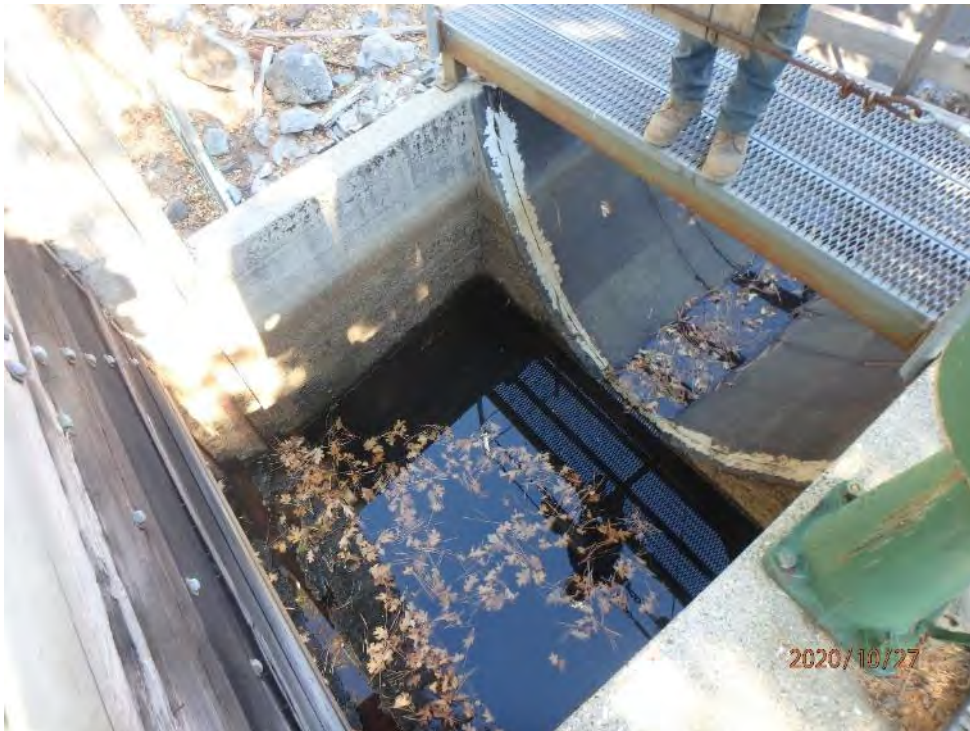
Photo 15 - View of Bear Valley Spillway
