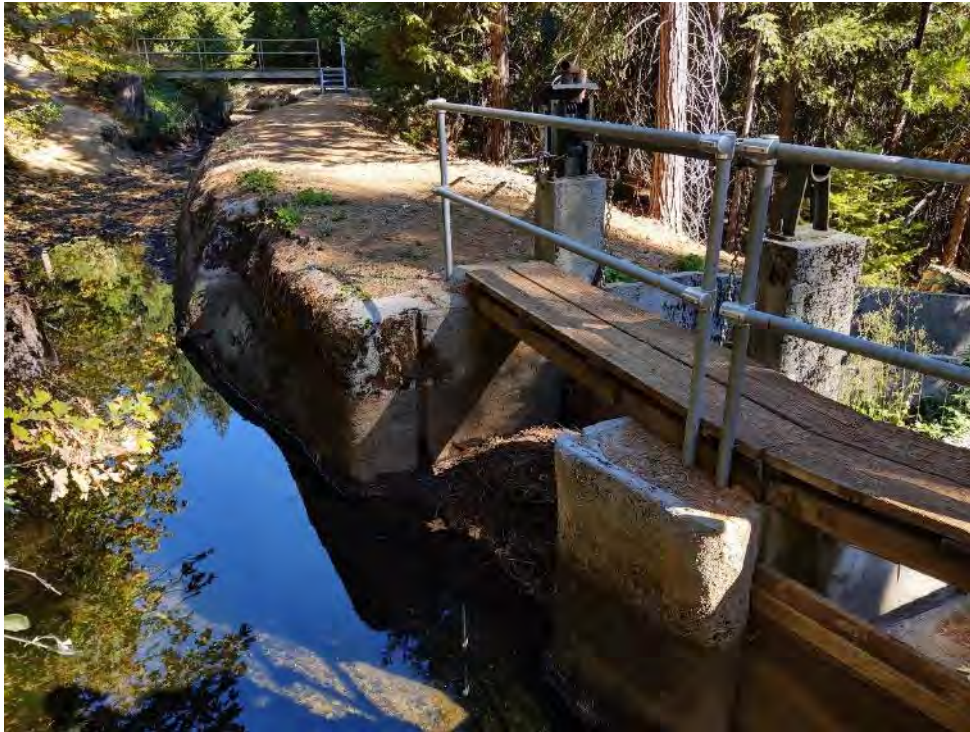
Photo 36 - View of Little Tunnel Spillway
