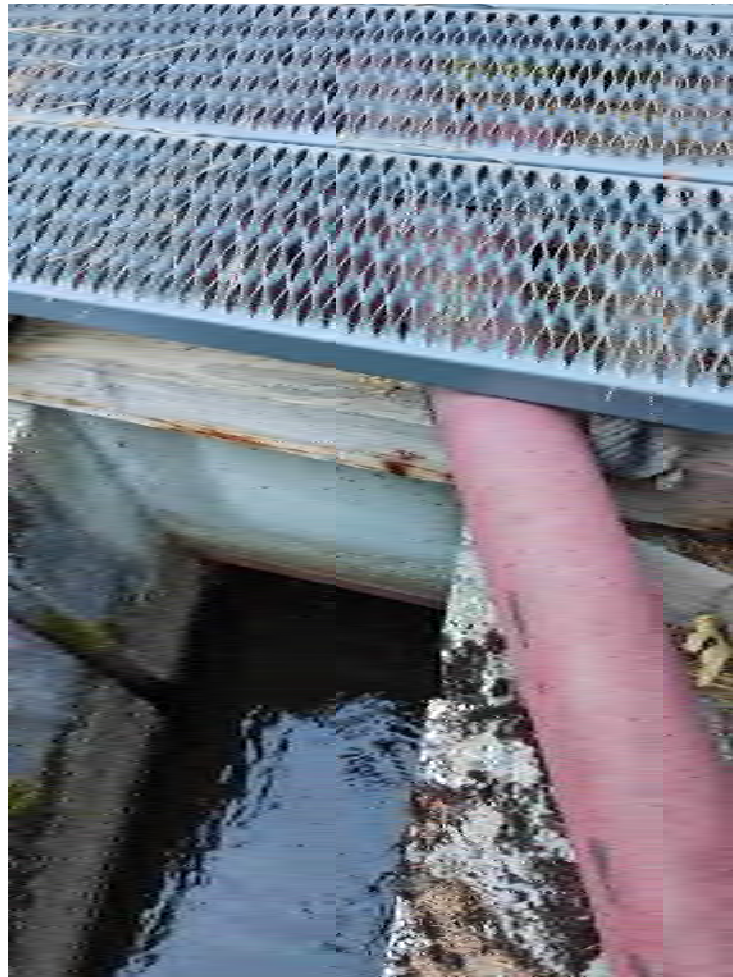
Photo 67 - View of 9 ½ Mile Spill Siphon
