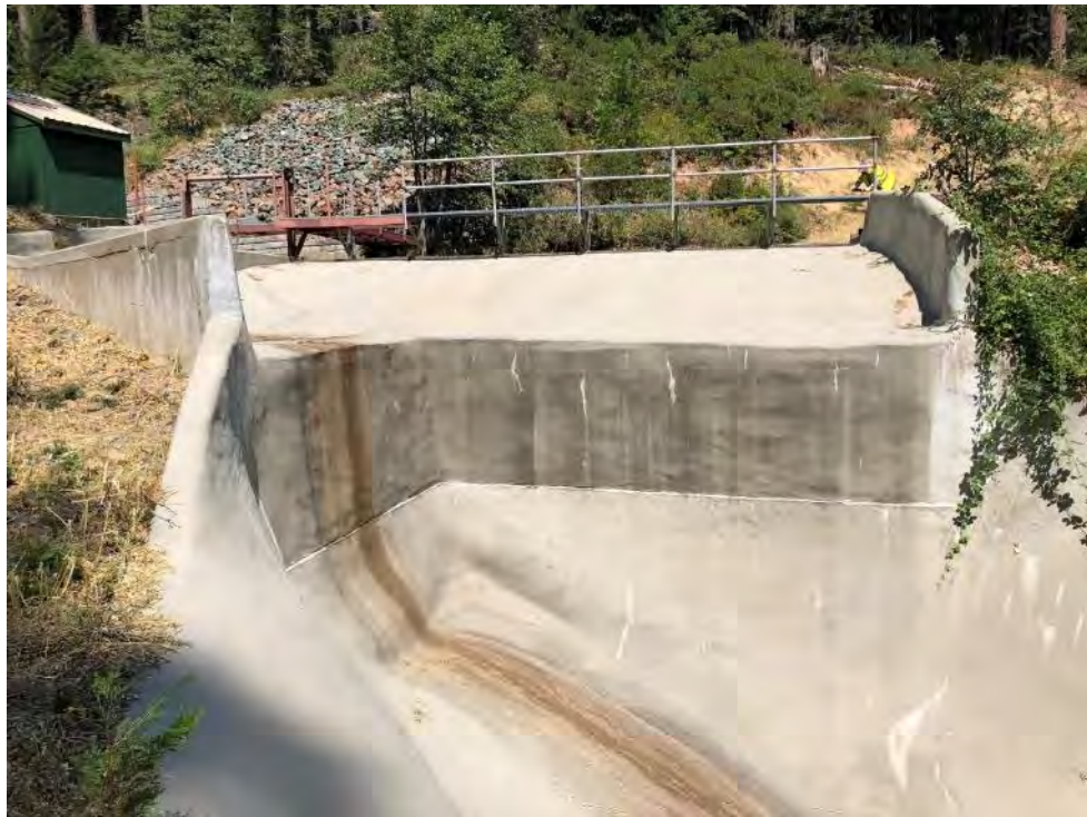
Photo 133 - View of Big Tunnel Spillway
