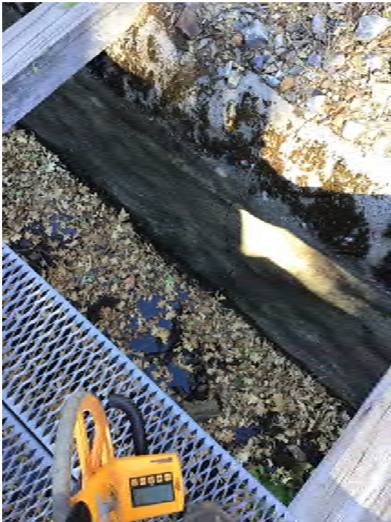
Photo 3 Cracking in Liner
