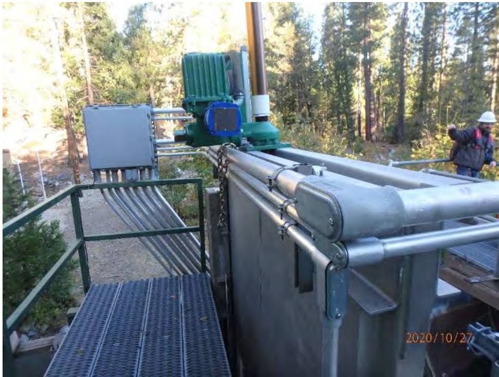
Photo 5 - View of YB139 Spillway
