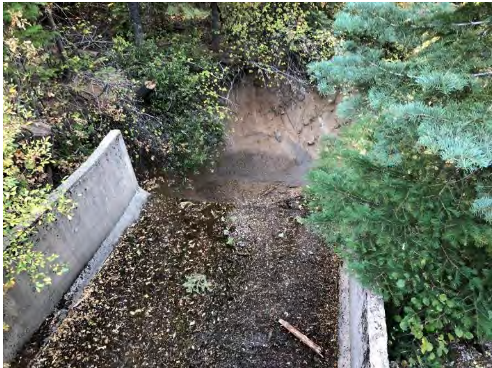
Photo 157 - View of Sandsettler Spillway
