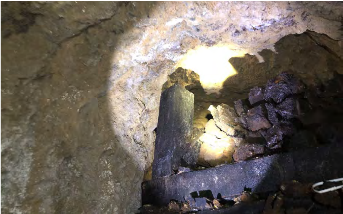
Big Tunnel Timber Crib 8+43
