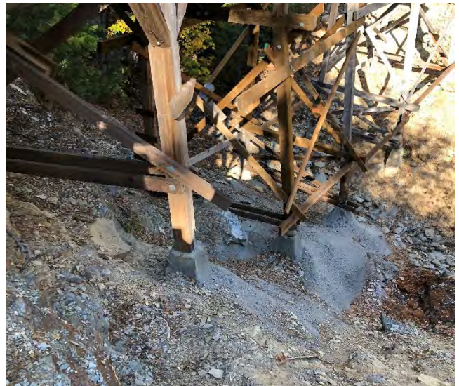
Photo 33 Shotcrete Repair at Flume Abutment
