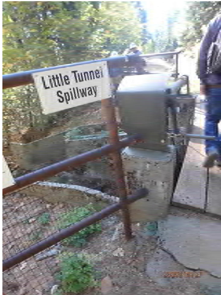
Photo 40 - View of Little Tunnel Spillway
