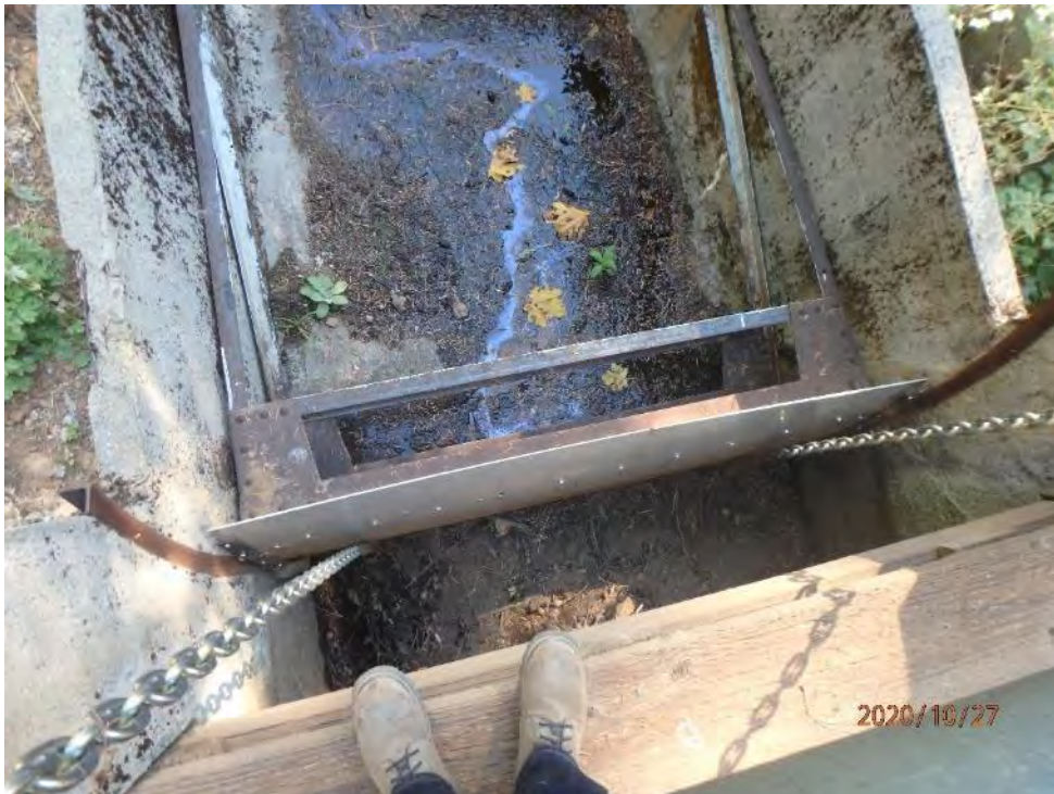
Photo 42 - View of Little Tunnel Spillway
