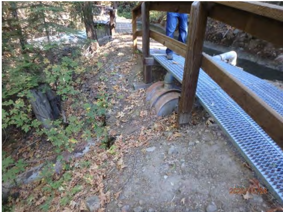
Photo 87 - View of Excelsior Point Spill Siphon
