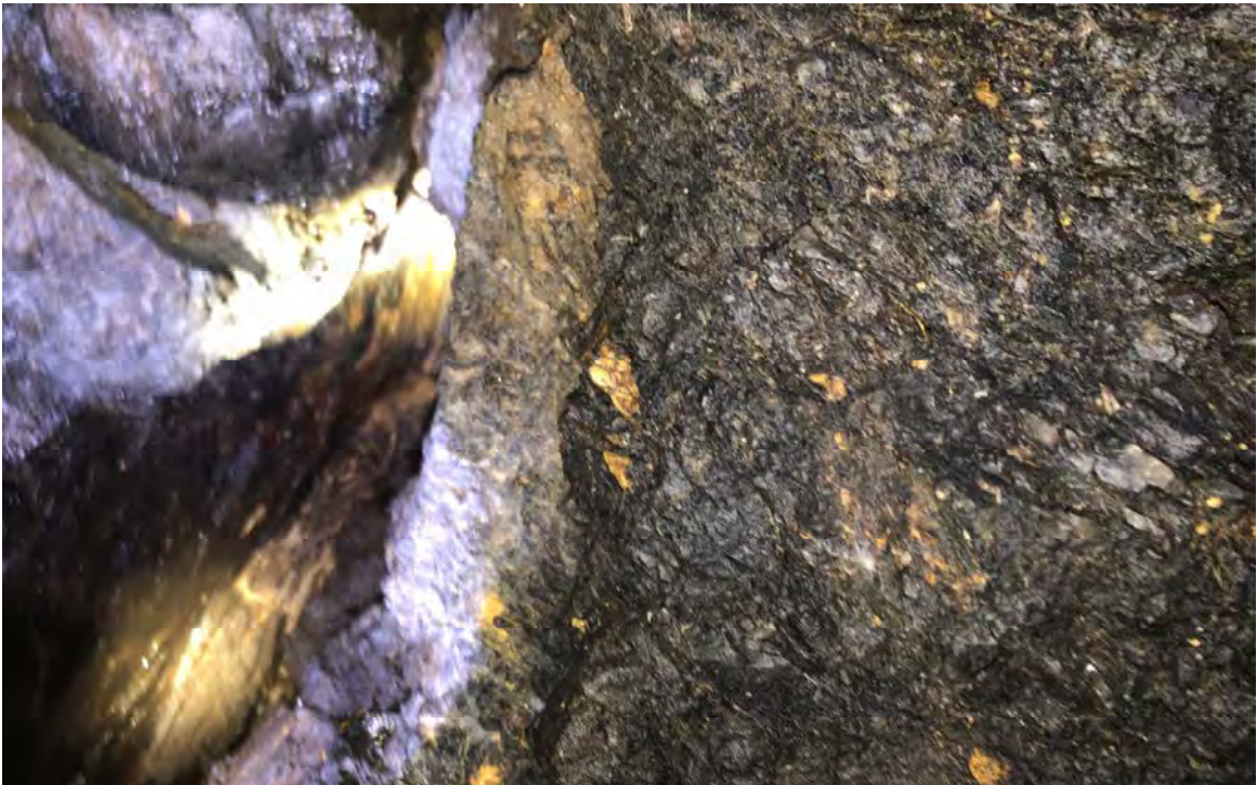
Big Tunnel 19+91 Shear
