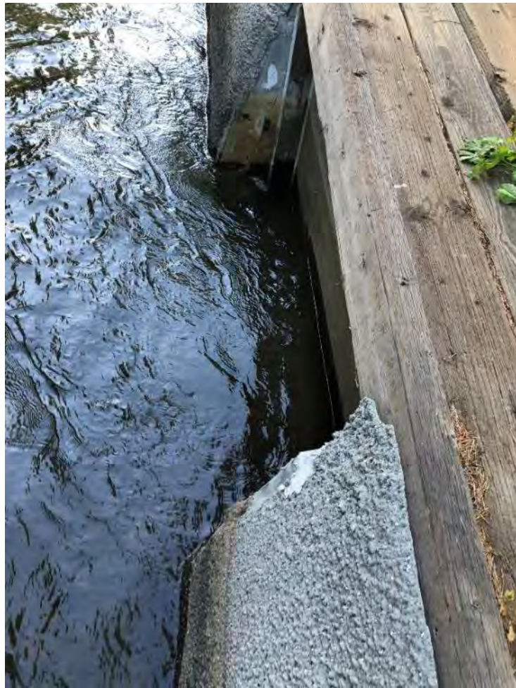
Photo 163 - View of Yunks Spill
