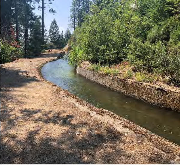
Photo 34 Slump in Bench
