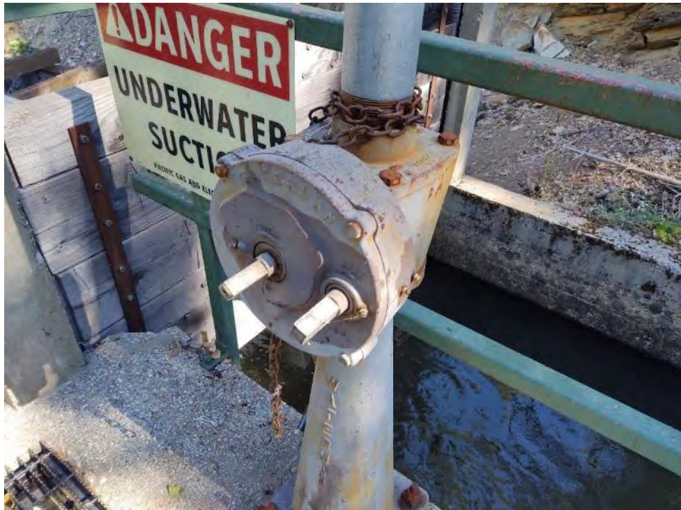
Photo 108 - View of 13 Mile Spillway
