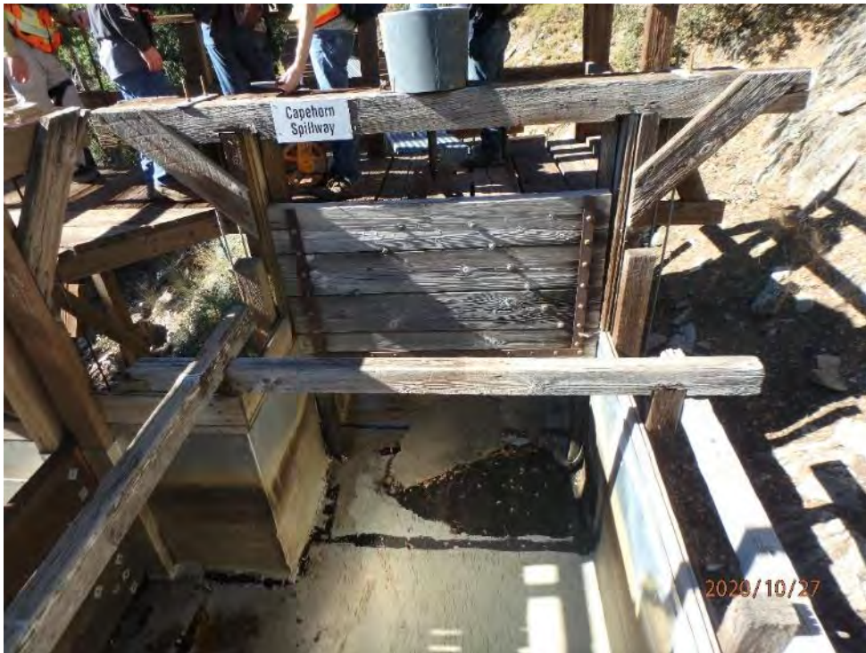
Photo 27 - View of Capehorn Spillway
