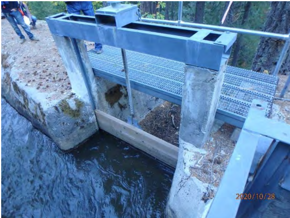
Photo 60 - View of 9 1/2 Mile Spill
