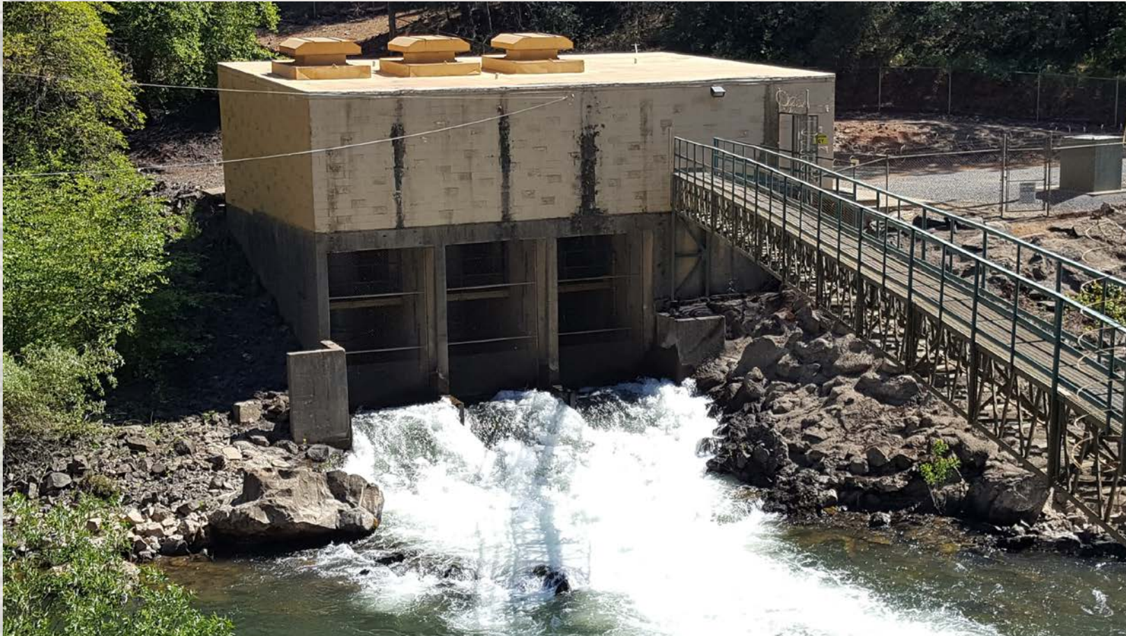
Combie South Powerhouse Access Improvement
