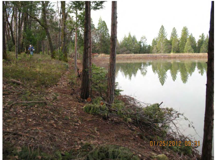
Photo 4. South shore and dam.
