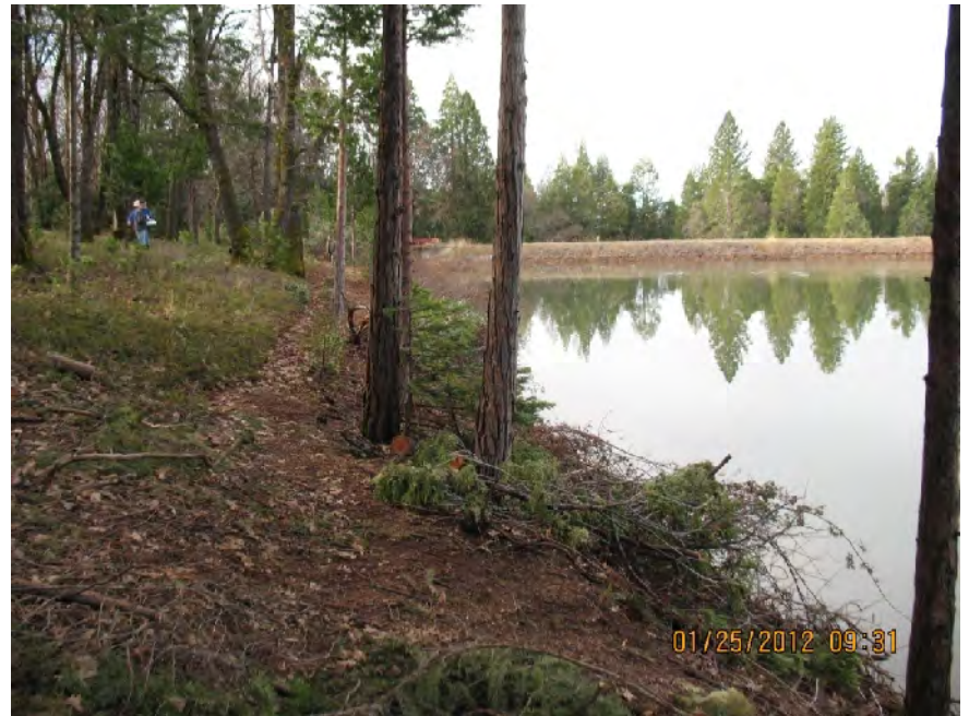
Photo 4. South shore and dam.
