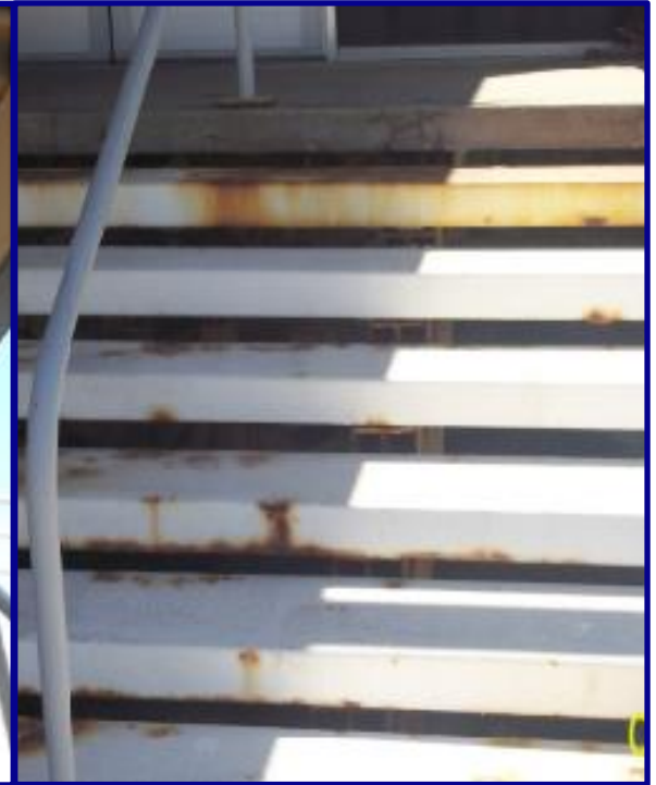
Stairs to lobby, customer service
