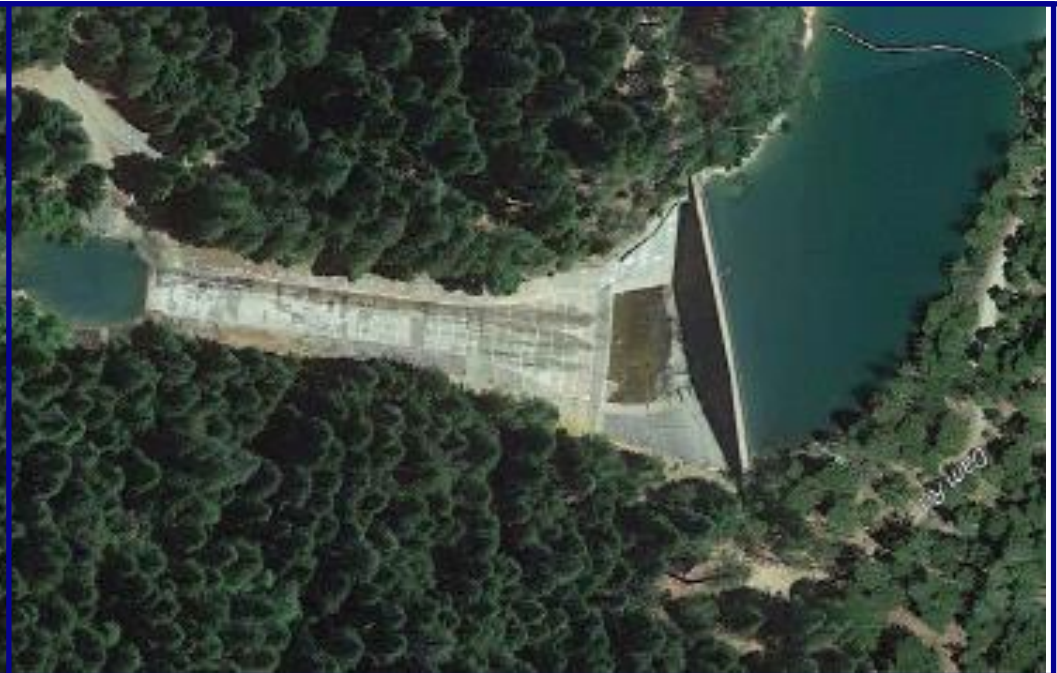
Scotts Flat Spillway
