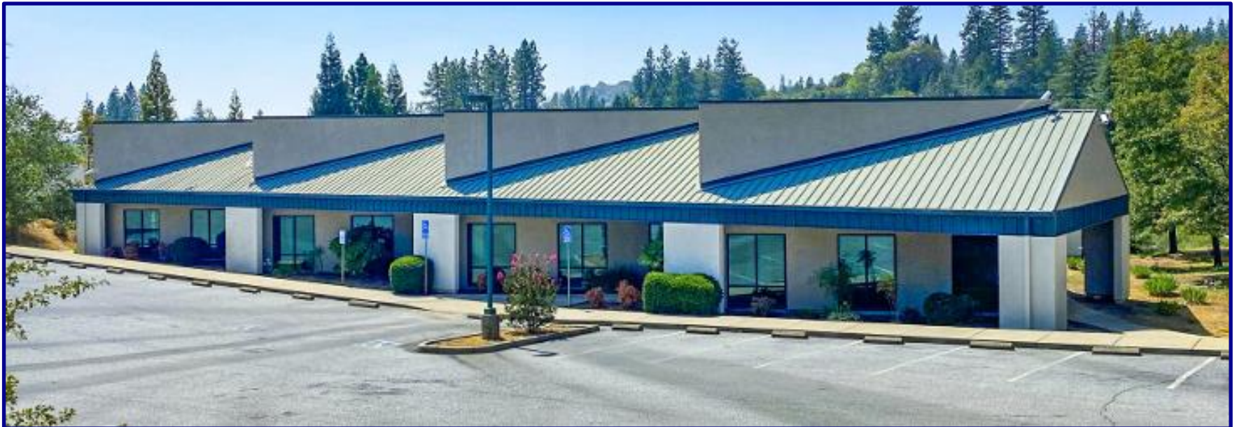
New Hydroelectric Field Office - Colfax
