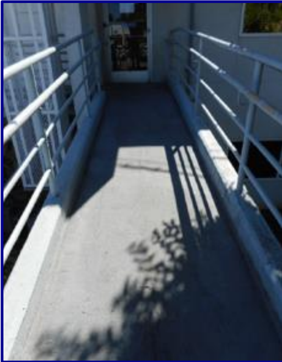
Walkway to Operations entrance
