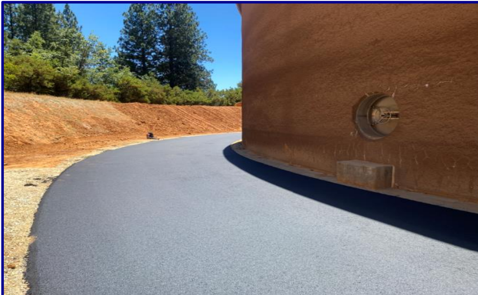
Side view of water tank
