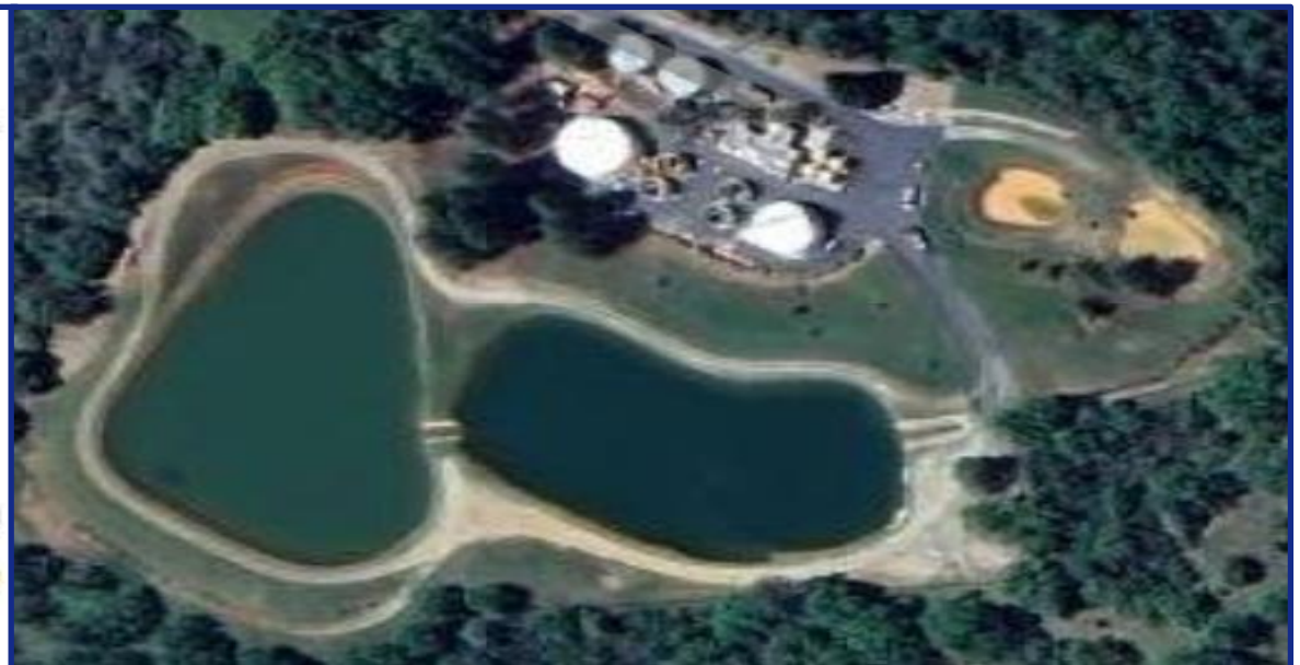
Lake Wildwood Water Treatment Plant
