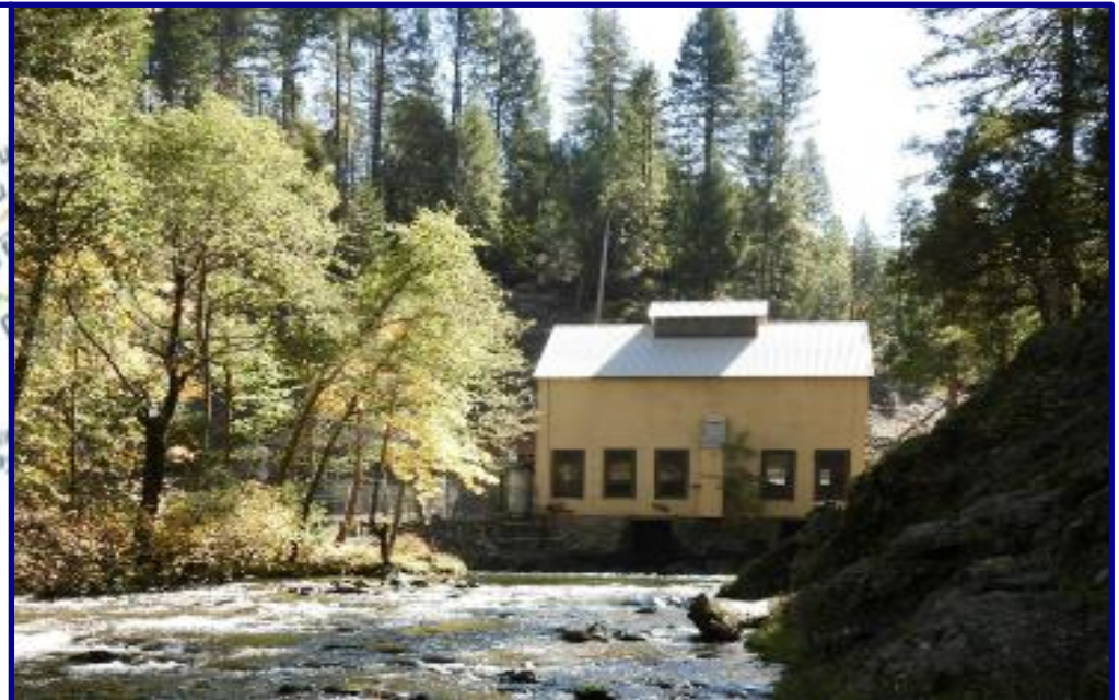
Deer Creek Powerhouse
