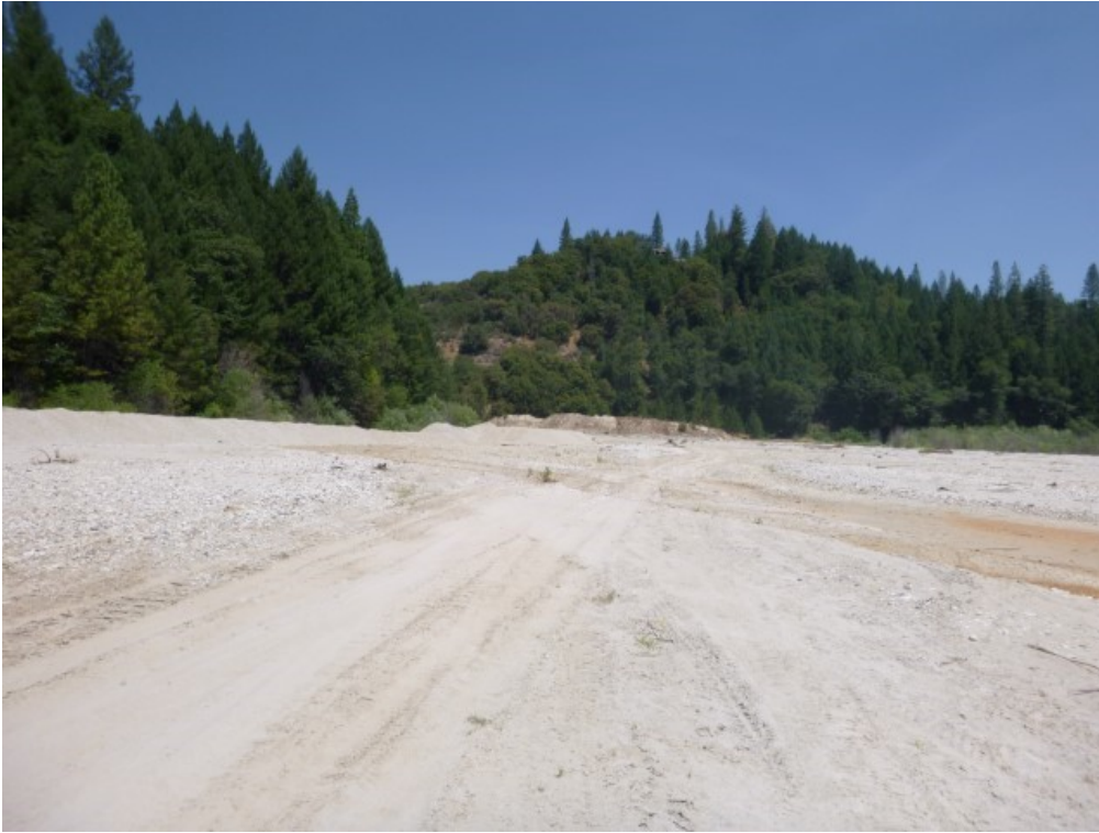
Photo 3.1-5 SA-2 and stockpile area, facing southeast.
