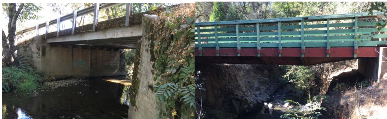
Figure 4-7: Bridge Crossing on Rough and Ready Highway (Left), and Bridge Crossing on Cook Road (Right)
