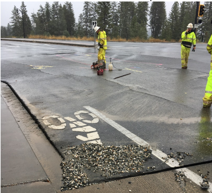
Maintenance Department: Dorsey Drive, transmission line break
