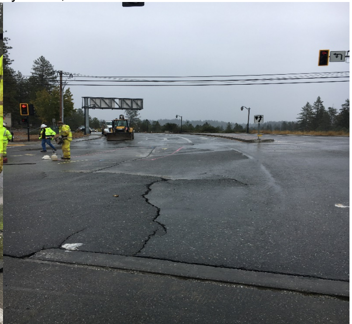
Maintenance Department: Dorsey Drive, transmission line break
