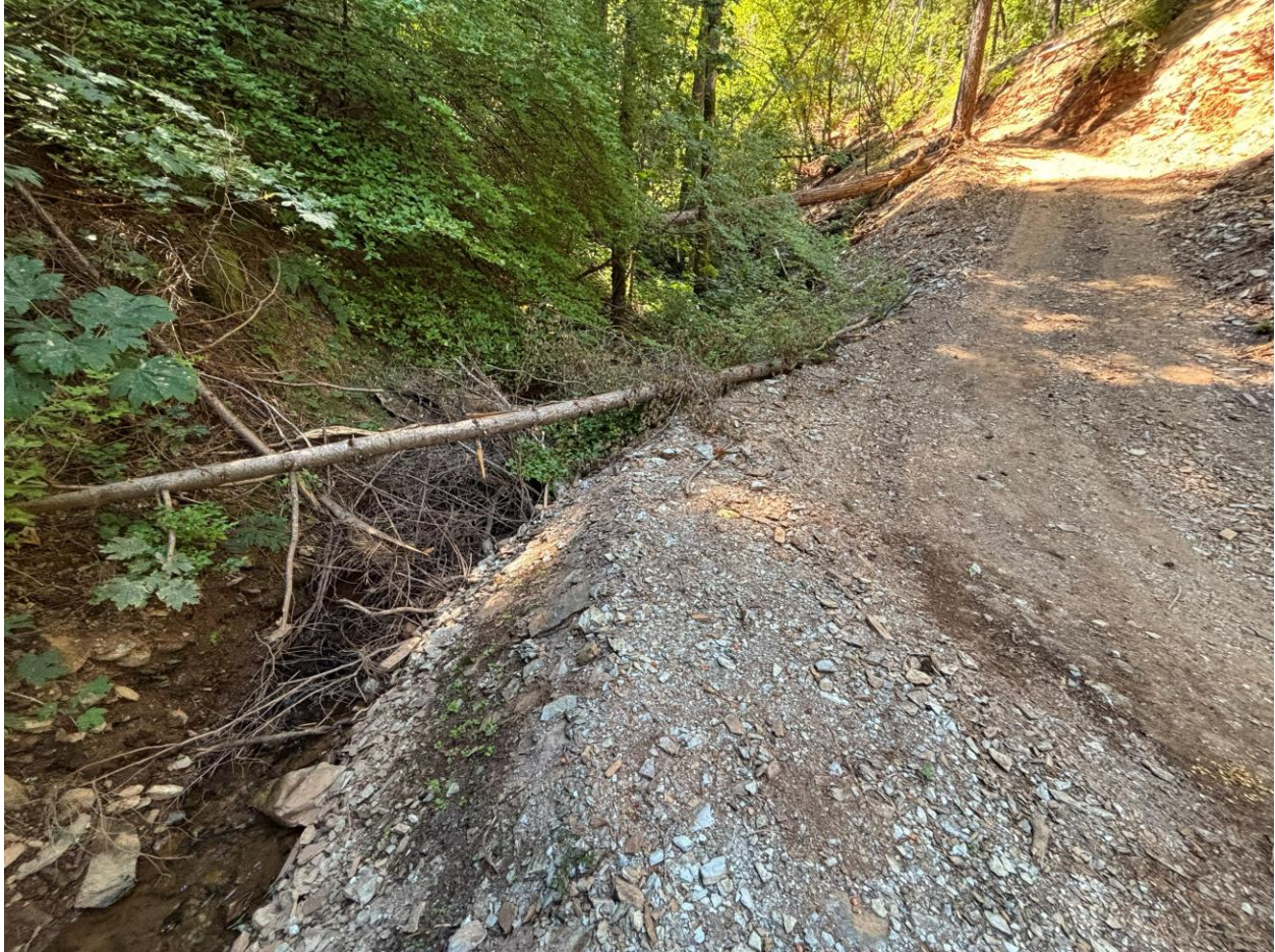
Road cut looking uphill (south) on NID property. Notice amount of debris / sediment pushed into Stampede Canyon creek on the left of the photo.
