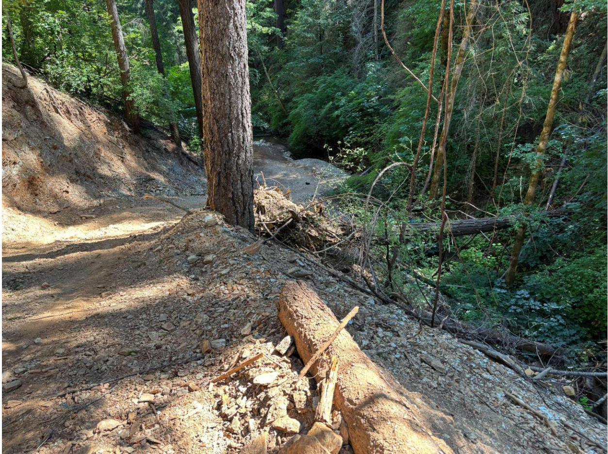
Road cut looking downhill (north), Stampede Canyon creek on the right side of the photo. Landing pad / Rollins Reservoir in the background.
