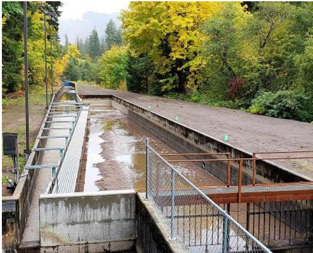
Figure 23 – The re-built Davenport screen prior to operation
