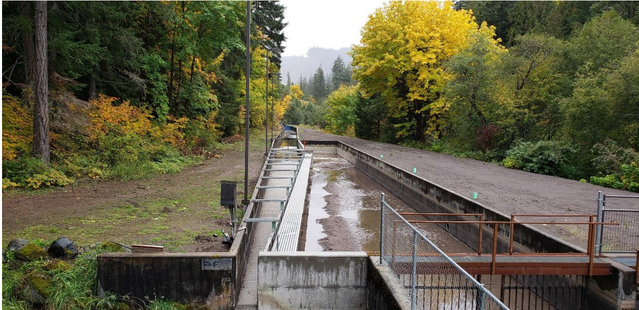
Figure 1. Finished retrofitted Davenport screen with a 14 to 1 taper ratio, emulating the geometry of the screen at the Derby Dam.
