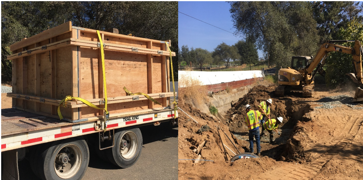
Placer Maintenance Department, headwall structure installation, Fruitvale Road
